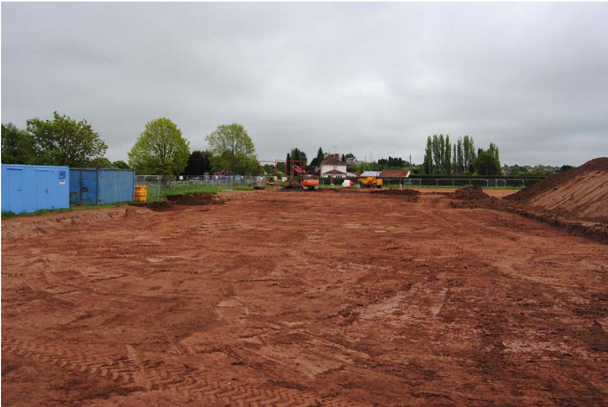
Plate 1 The site looking south.
