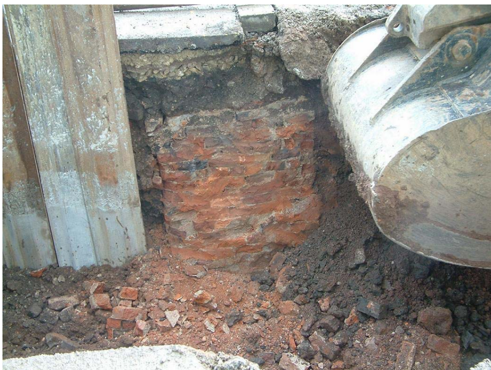
Plate 2. Brick structure extant in south-east section, view south-east
