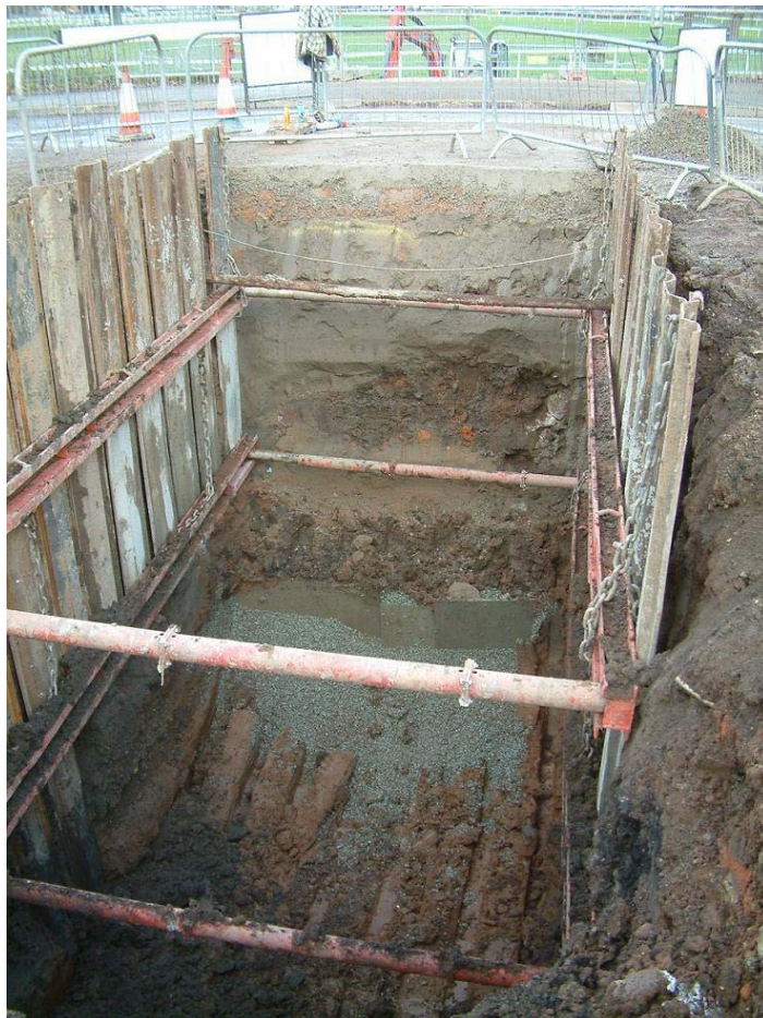
Plate 4. General shot of trench, view north-east
