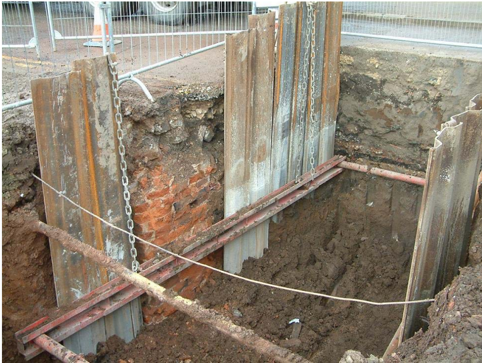
Plate 3. Brick structure extant in north-west section, view north
