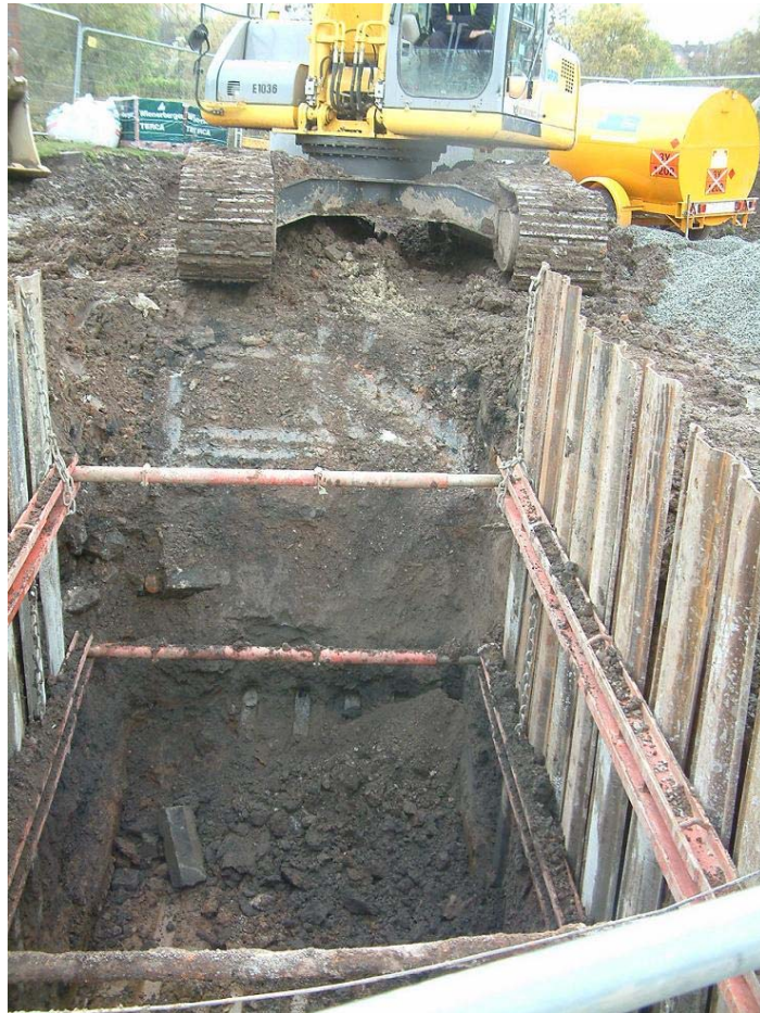
Plate 5. General shot of trench in progress, view south-west
