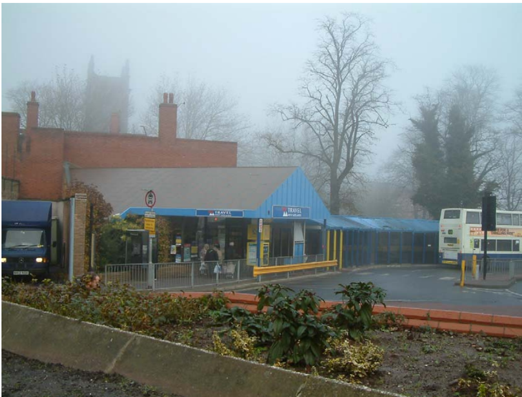
Plate 4. West midlands Travel Centre with St Edmund's Church in the background
