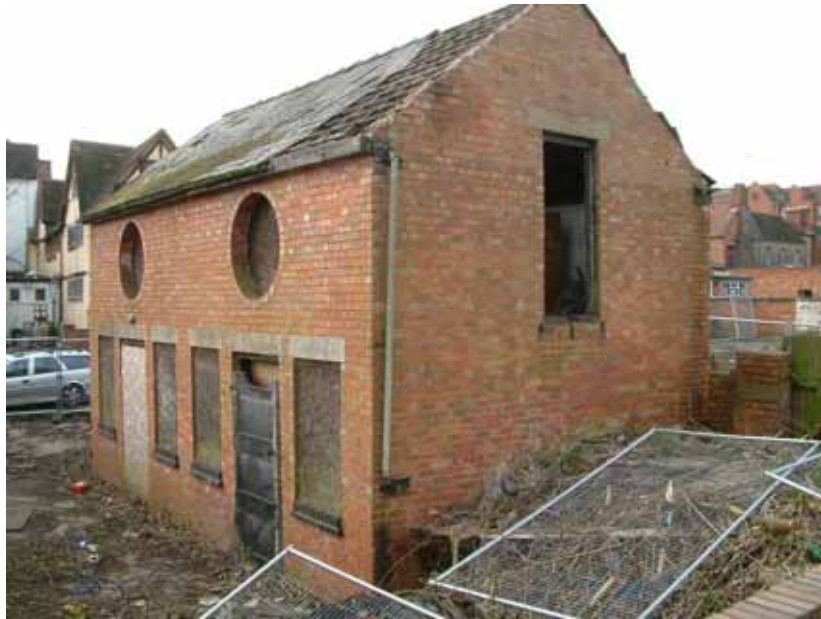
Plate 3: "Brewery building" prior to demolition
