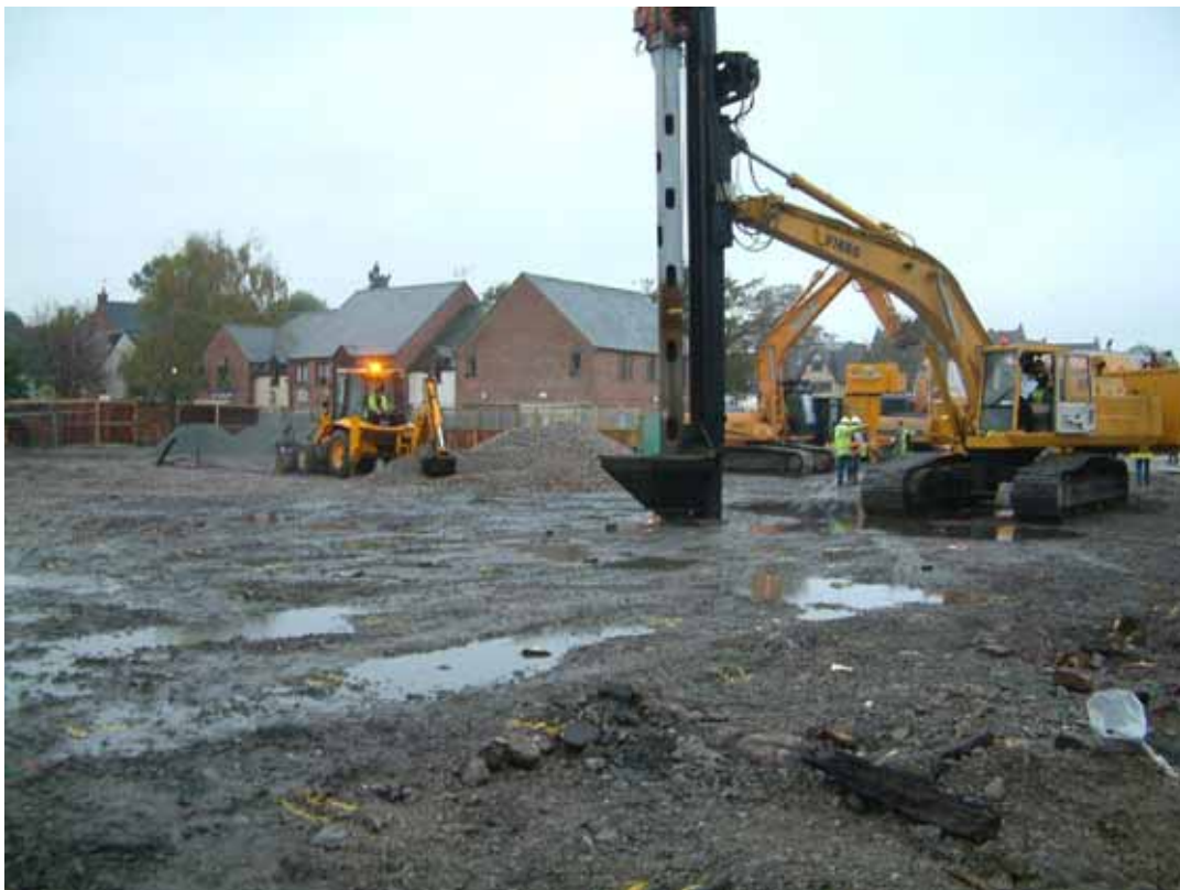
Plate 8: Vibroplacement works taking place
