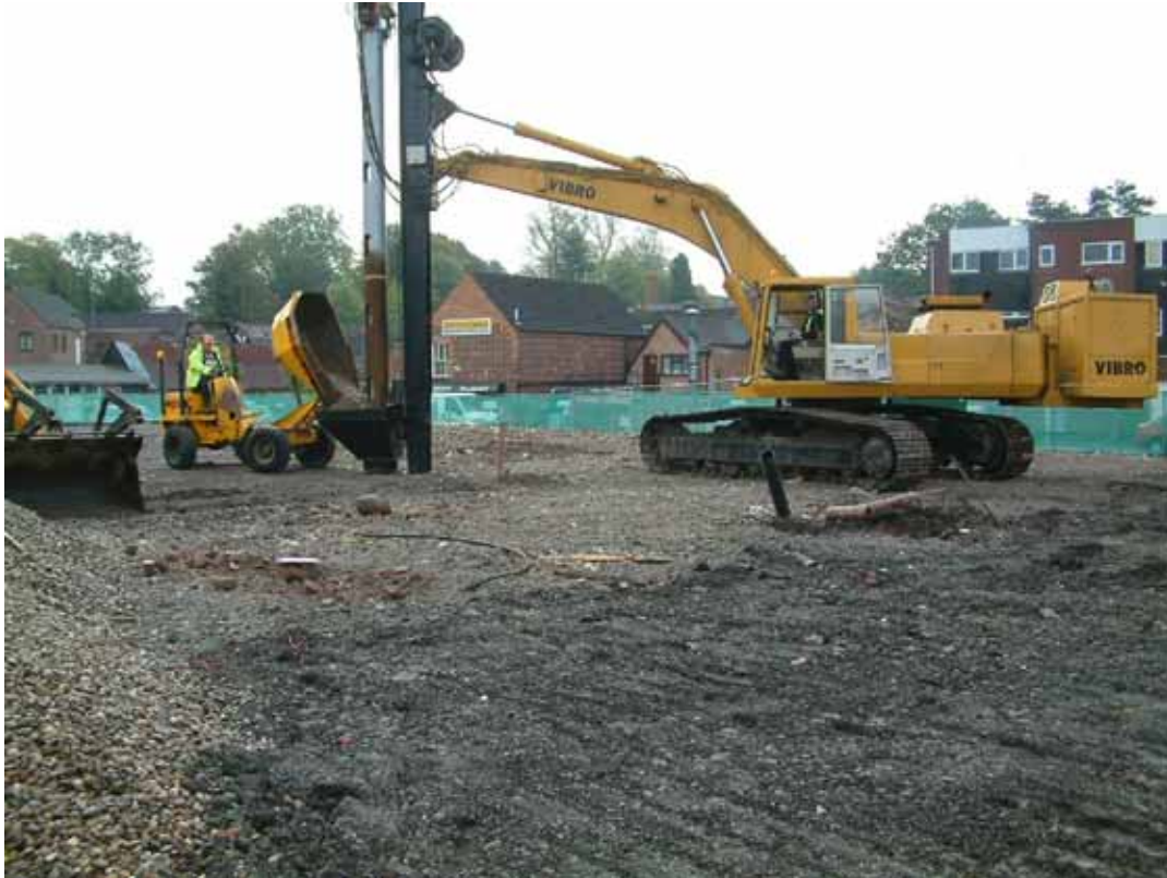
Plate 9: Hopper being loaded with aggregate
