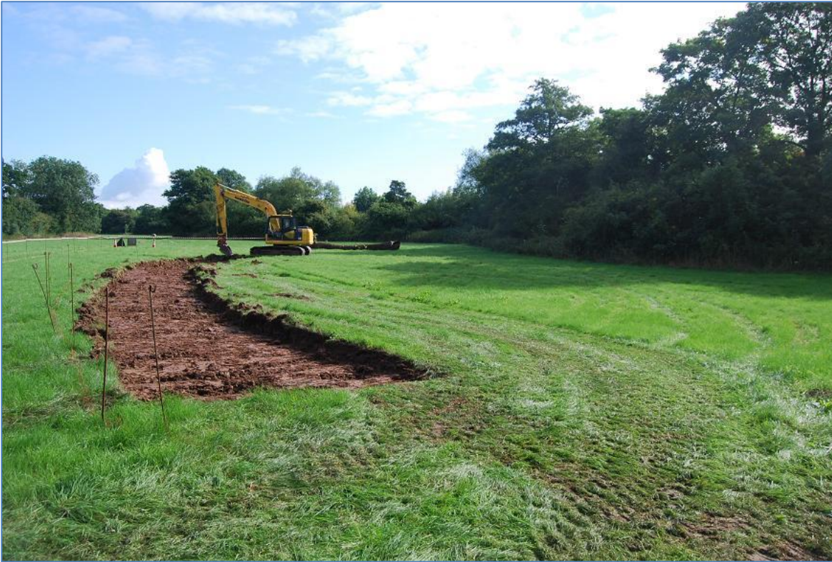
Plate 1 Topsoil strip showing natural hollow at location for pond, view north
