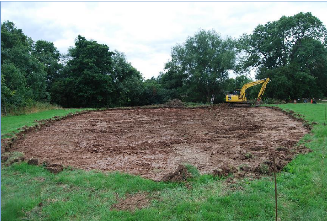
Plate 5 Wetland pond site strip complete, reduced to natural clays, view south
