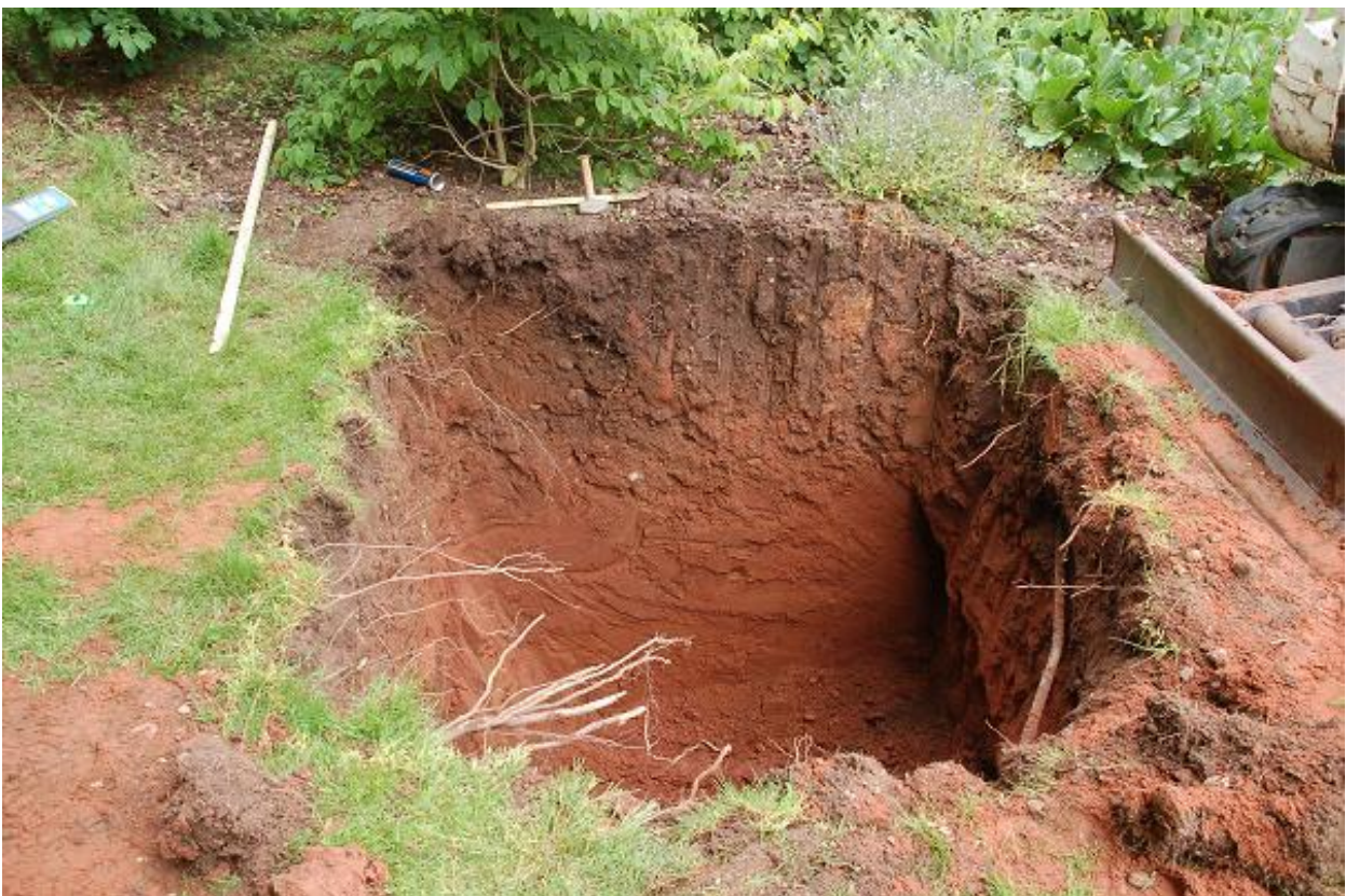
Plate 2 The area excavated for the septic tank (Trench 1), looking west
