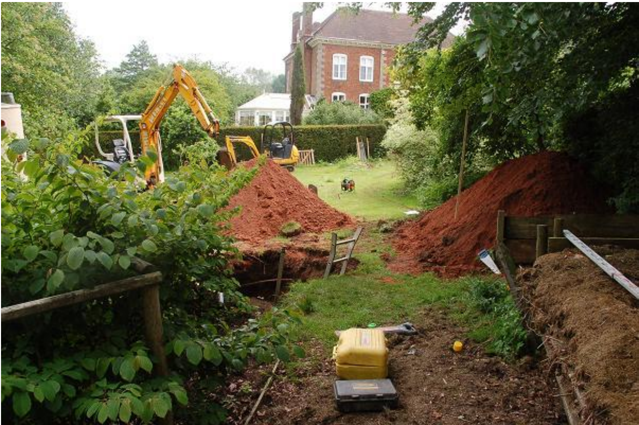
Plate 1 The site looking east during the excavation of Trench 1
