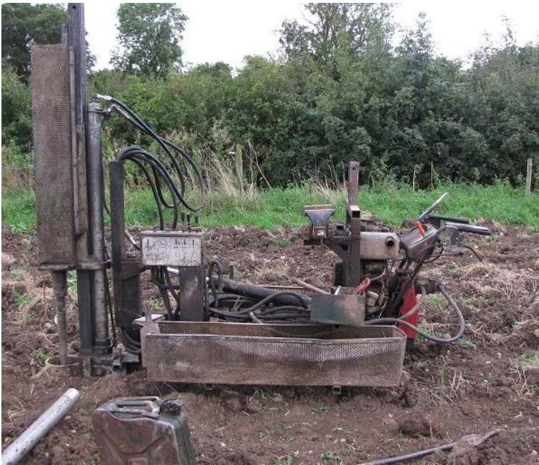
Plate 3 Borehole rig in operation at Borehole 3
