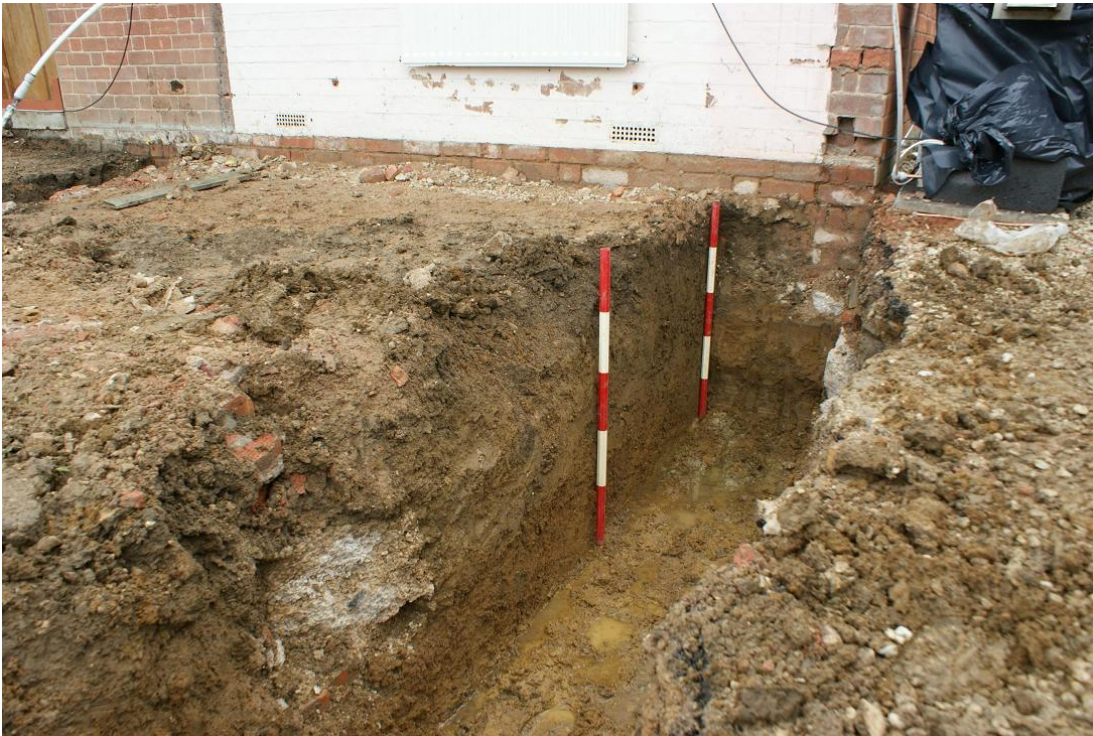
Plate 5 Trench 5 (foundation) section, view east
