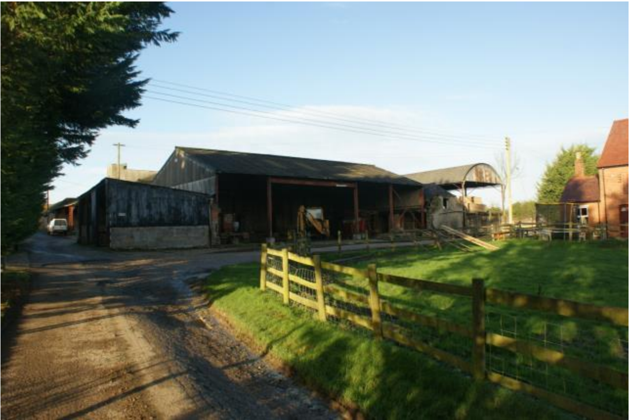
Plate 54 General view of the farm buildings, looking north-west
