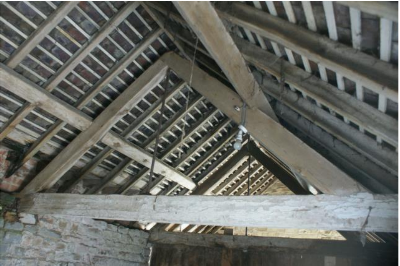
Plate 40 Phase 2 iron truss fixings
