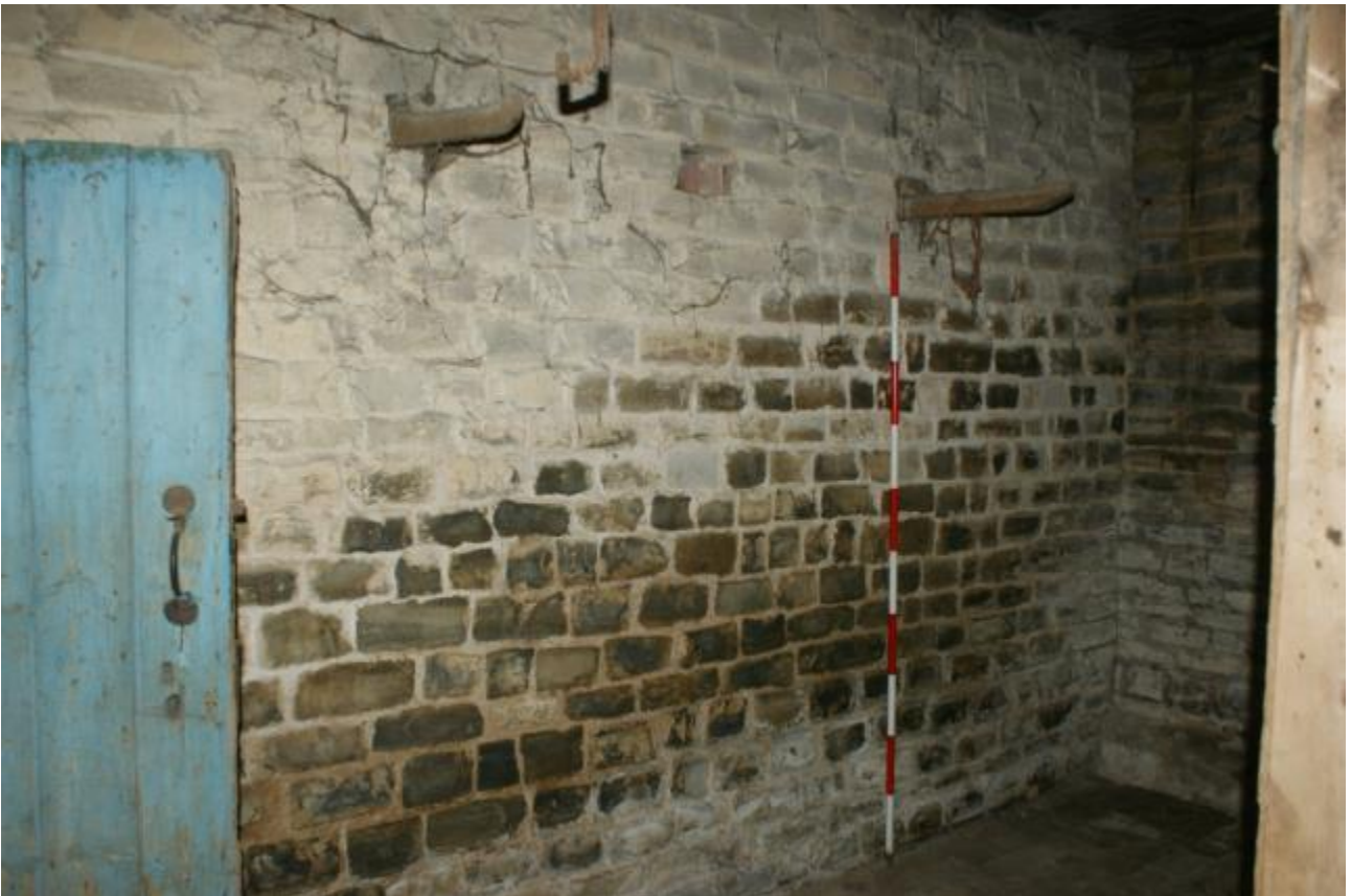
Plate 36 Phase 1 western north to south range
