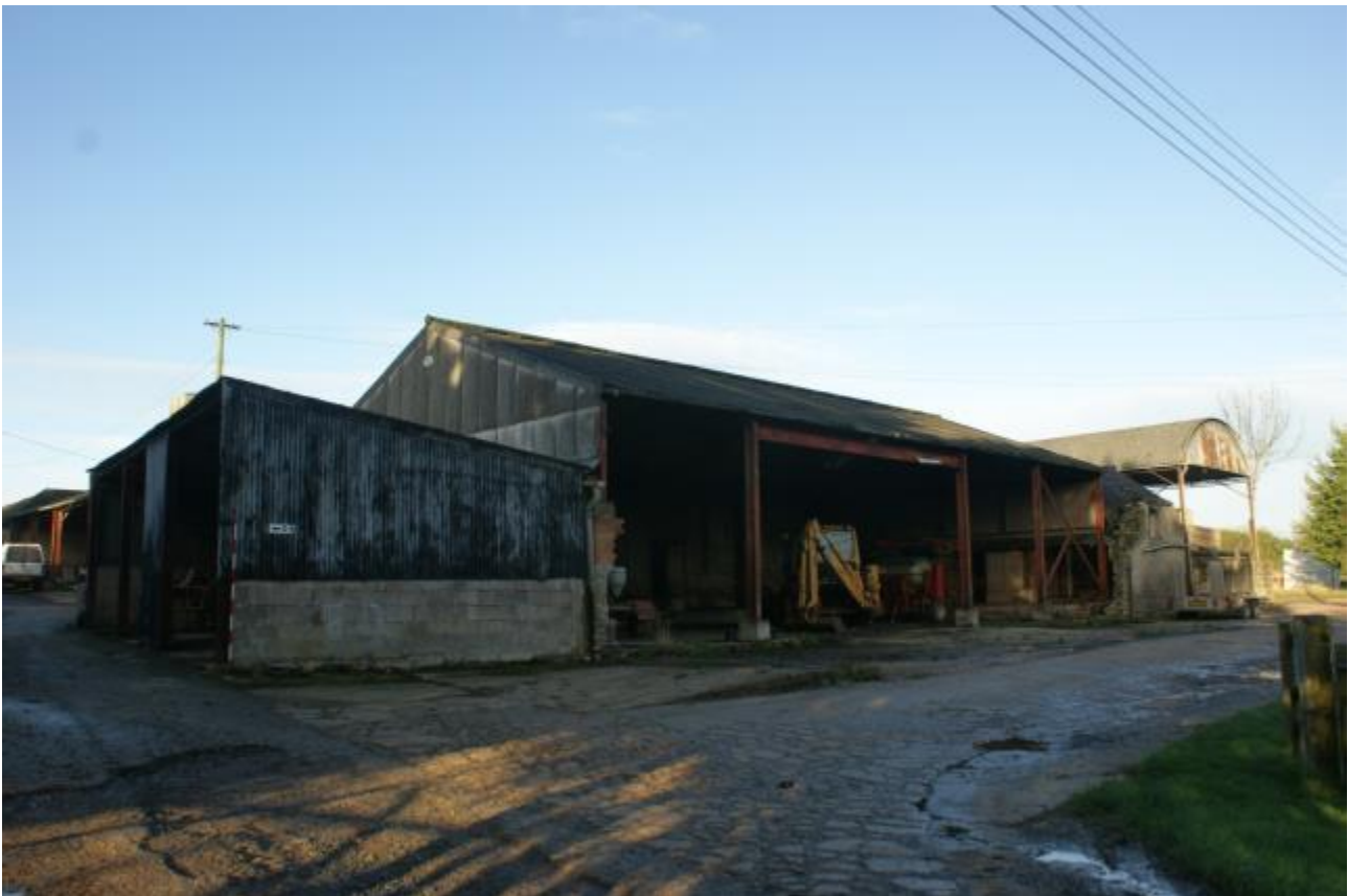
Plate 53 Phase 3 steel framed buildings
