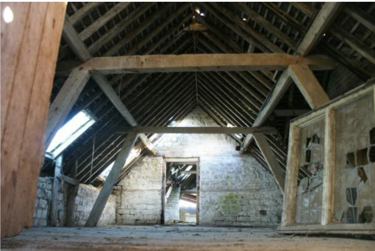
Plate 25 Phase 1 central east to west range
