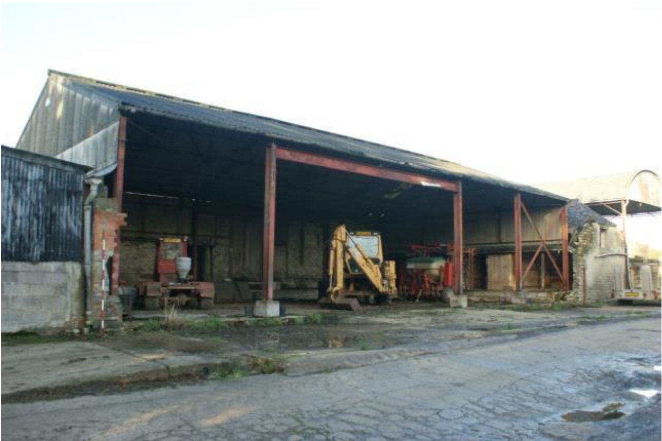
Plate 52 Phase 3 steel framed buildings
