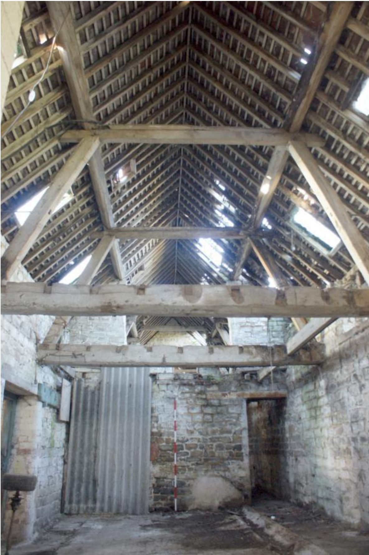
Plate 26 Phase 1 central east to west range
