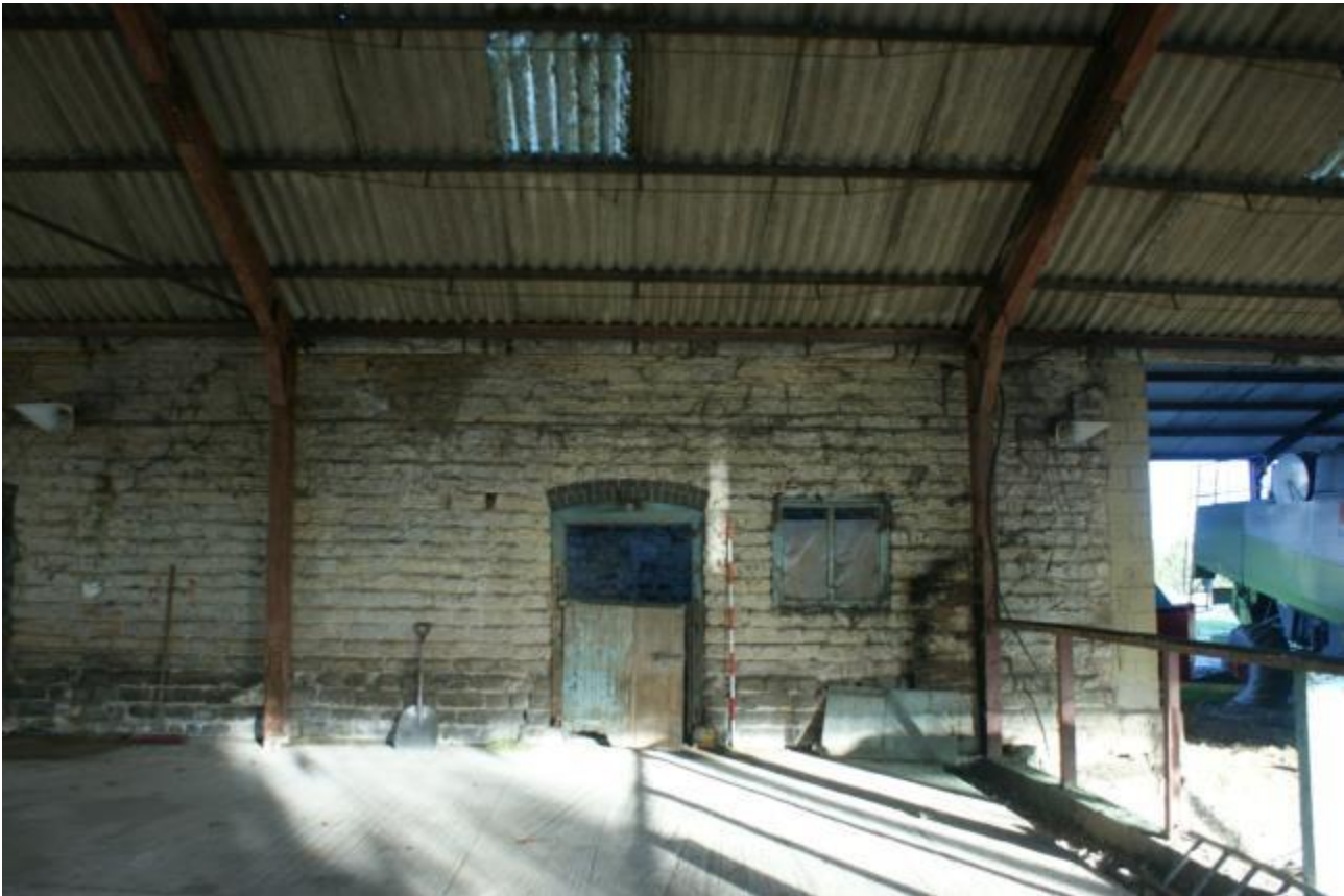
Plate 23 Phase 1 central east to west range
