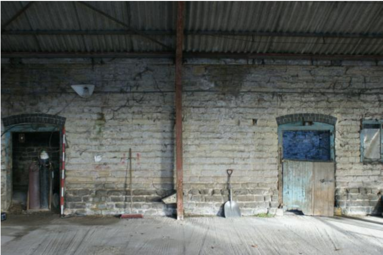
Plate 22 Phase 1 central east to west range
