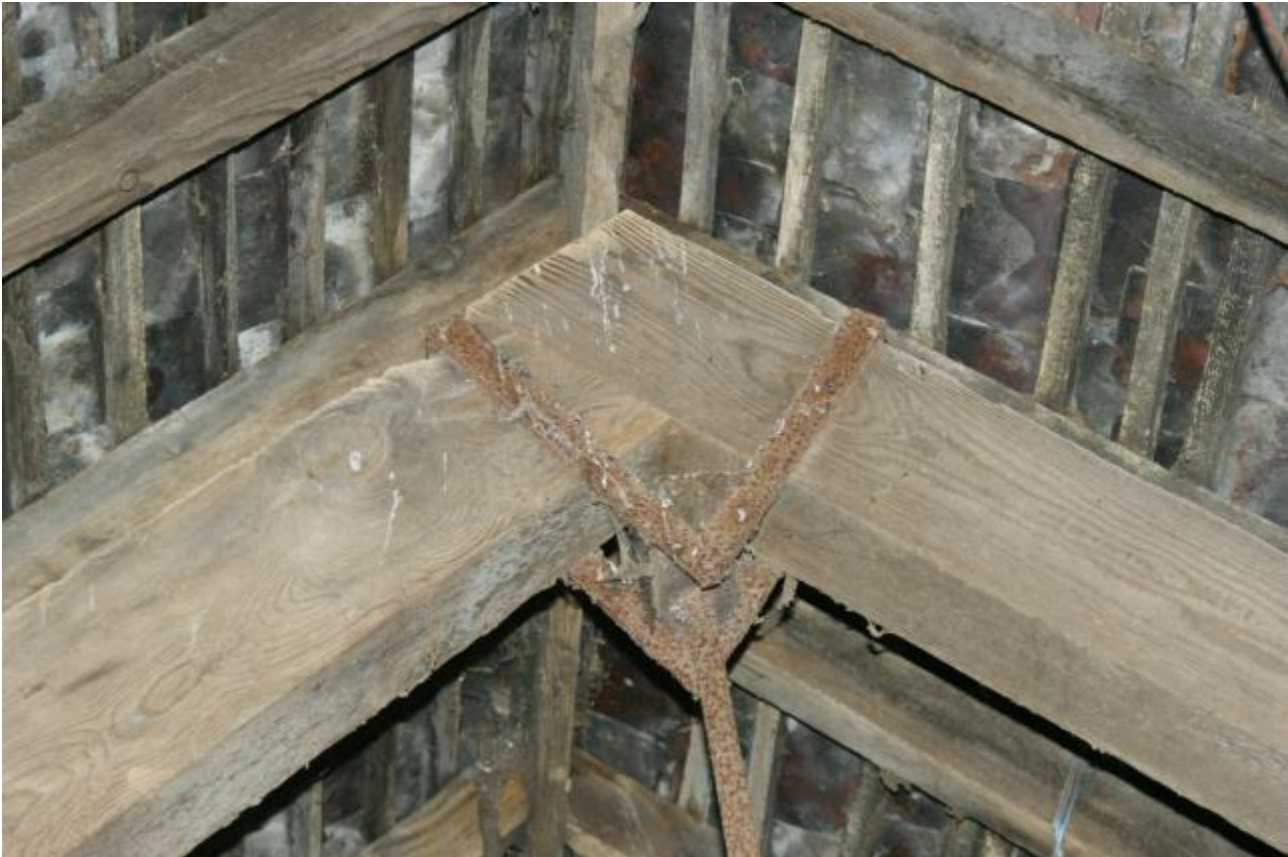
Plate 39 Phase 1 iron truss fixings
