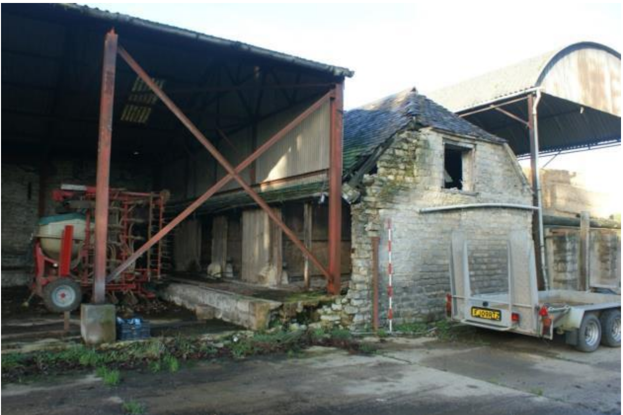
Plate 2 Evidence of a former boundary wall
