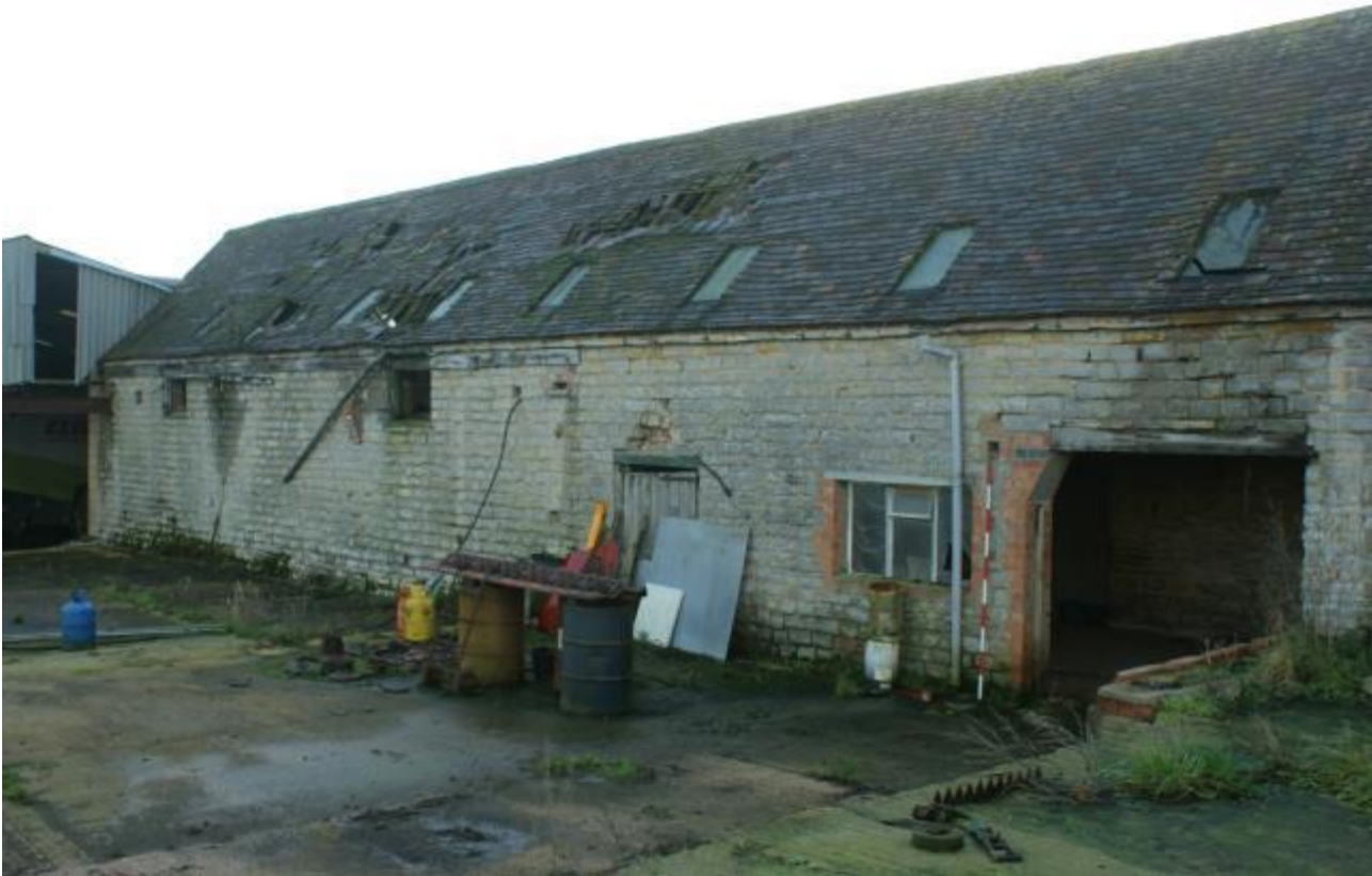
Plate 3 Phase 1 Structure showing string course detailing
