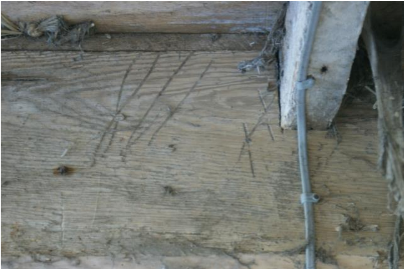
Plate 38 Phase 1 Baltic timber marks
