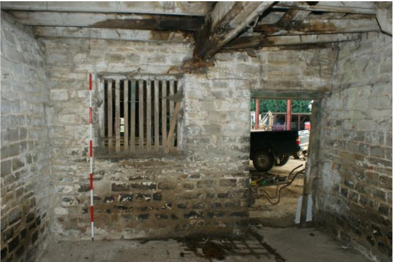
Plate 35 Phase 1 western north to south range
