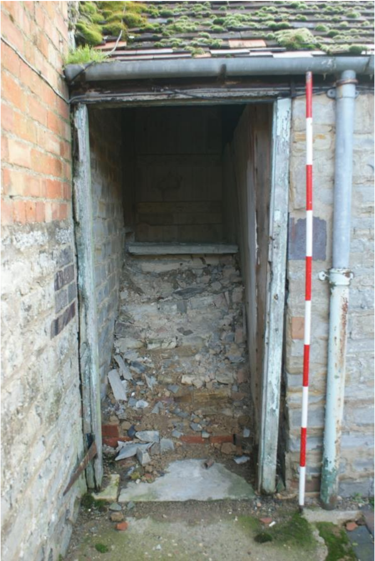
Plate 37 Phase 1 western north to south range
