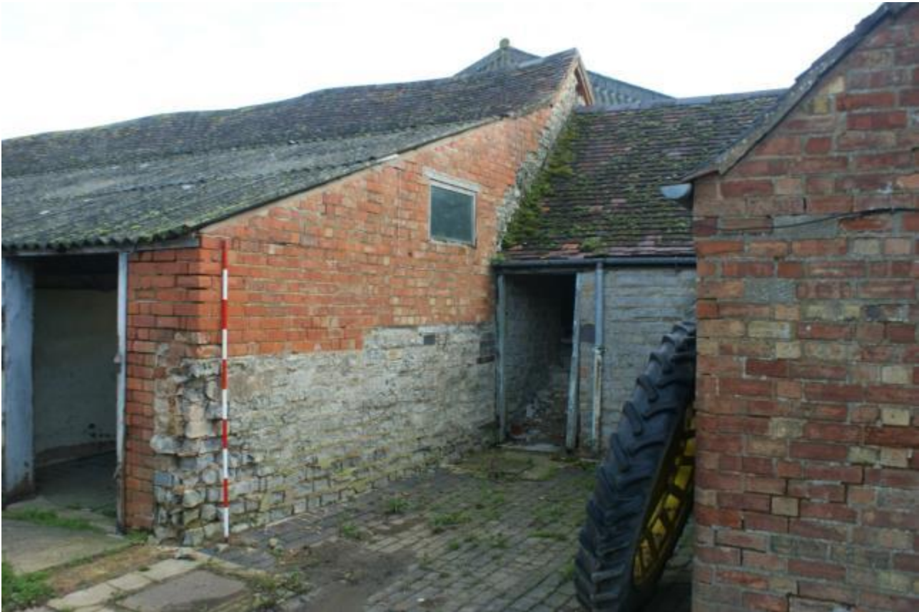
Plate 44 Phase 2 boundary wall
