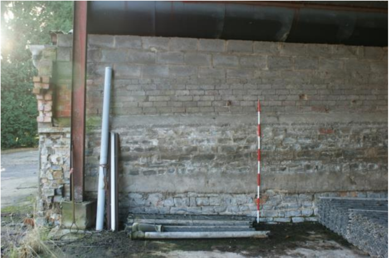
Plate 1 Former boundary wall
