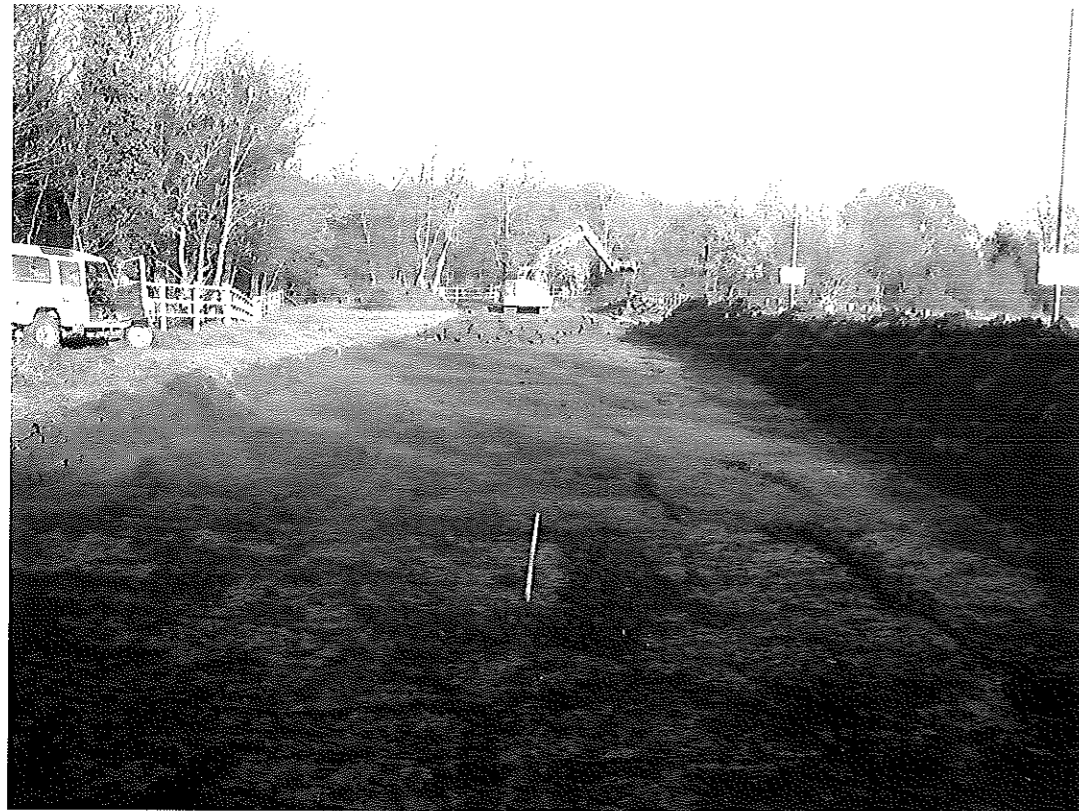
Plate 2: General view of Area 2, facing north-east
