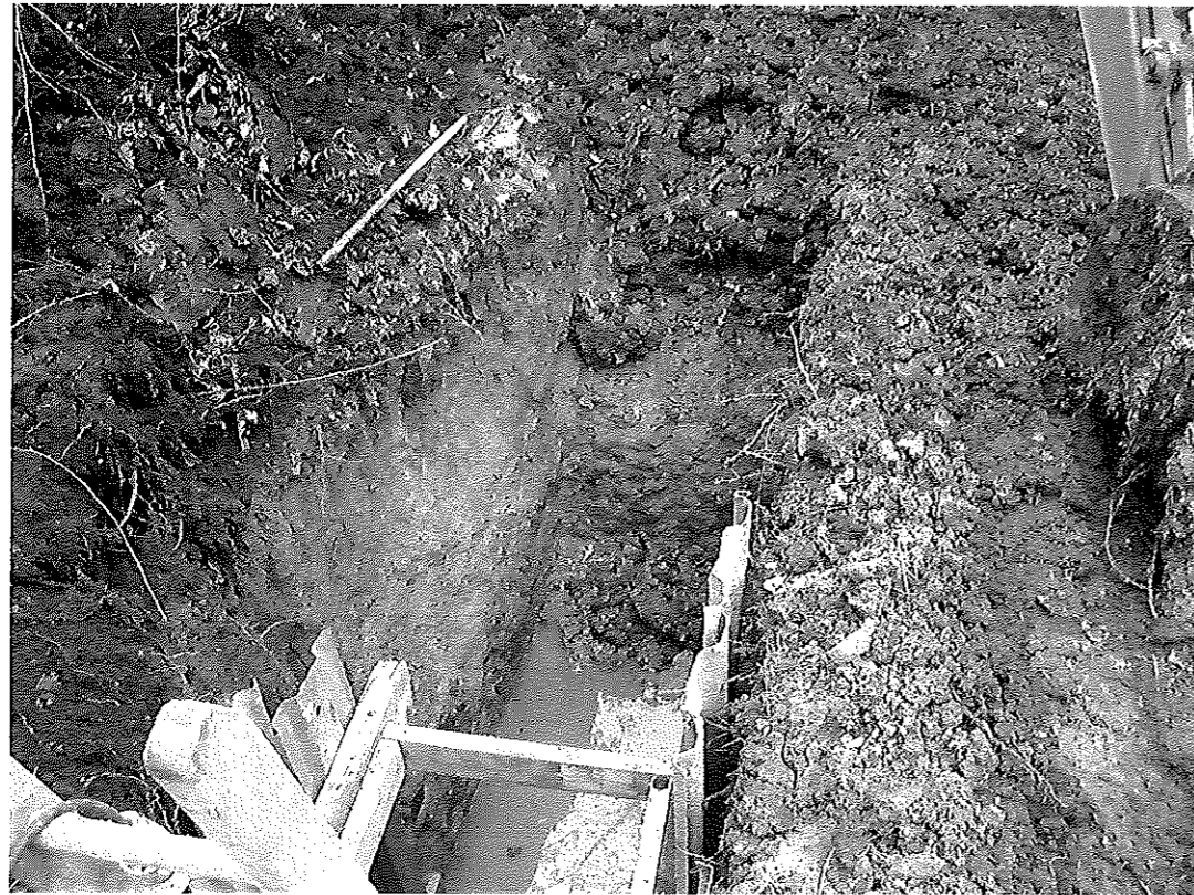
Plate 3: Excavation of service trench at southern end of Area 3, facing north-west
