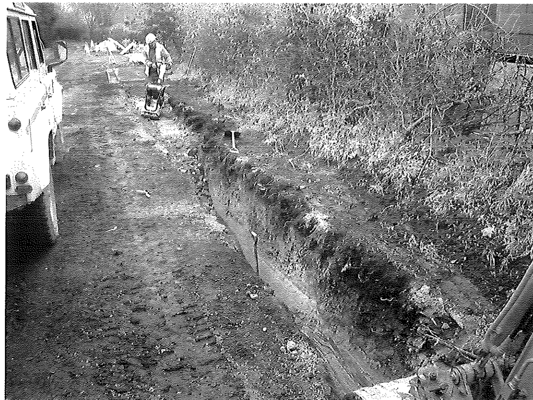
Plate 4: General view of service trench in Area 4, facing south-west
