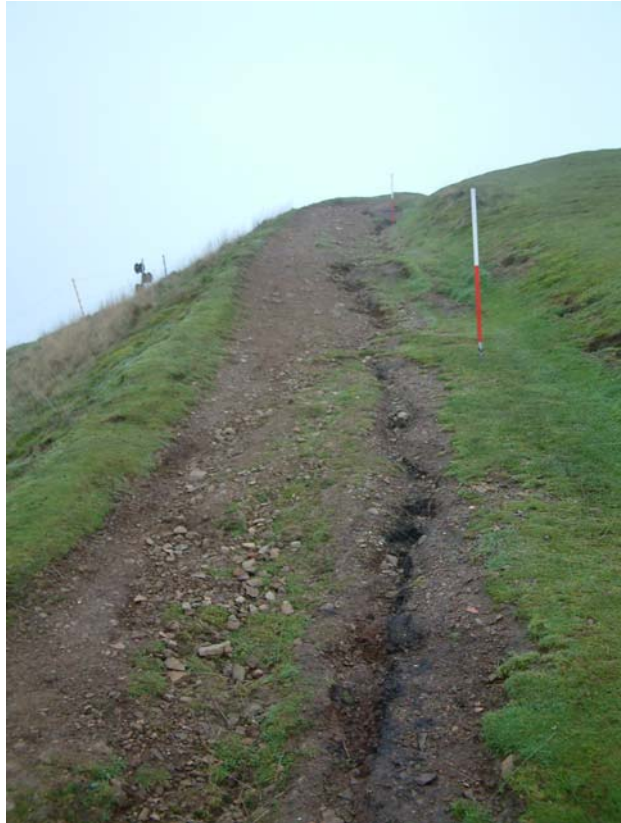
Plate 9: Unit 16, view south south east of water erosion to path on bank on Pinnacle Hill (Photo 128).
