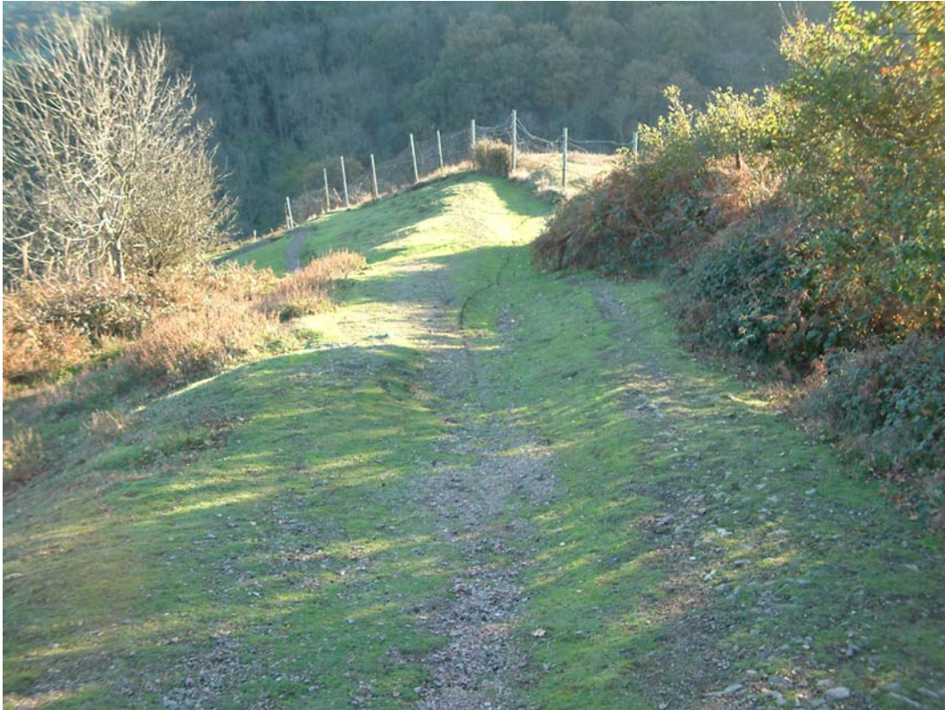
Plate 3: Unit 6, view south of erosion to bank and ditch on Swinyard Hill toward the Gullet Quarry (Photo 30).
