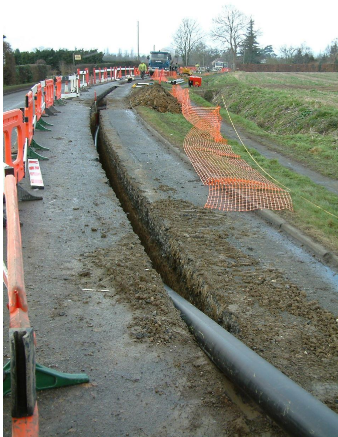
Plate 4: Trench 5, view west
