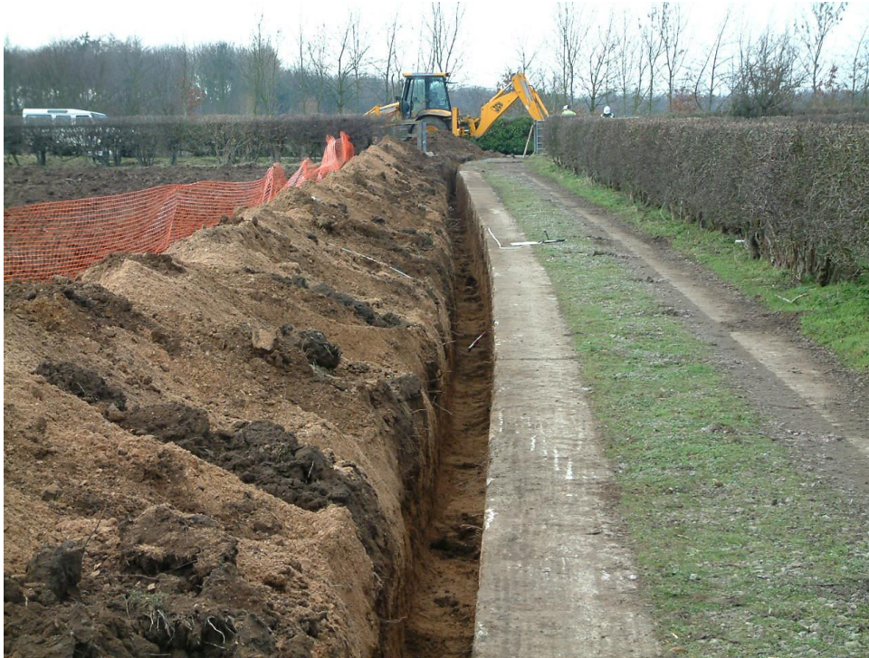
Plate 3: Trench 4, view west-north-west
