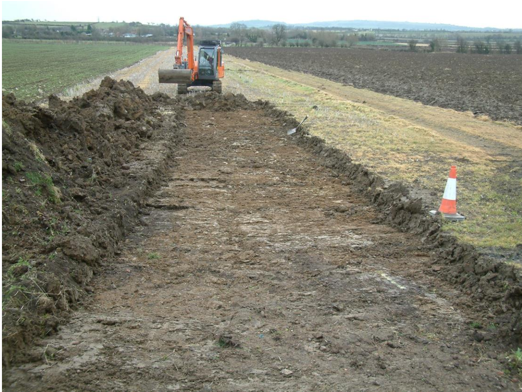
Plate 1: Removal of topsoil in Field 1, facing east
