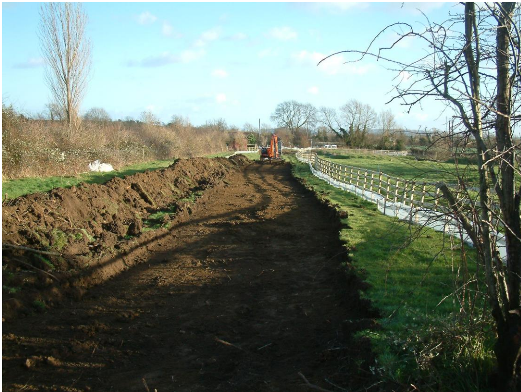
Plate 6: Removal of topsoil in Field 2, facing east
