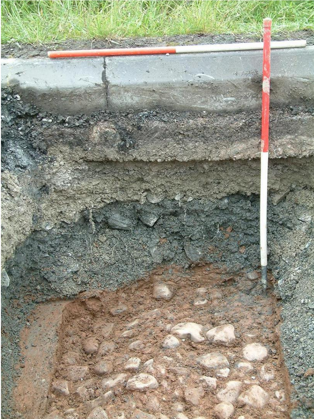
Plate 15, Cobbled road surface below existing modern road surface, view north (Fig 4b)
