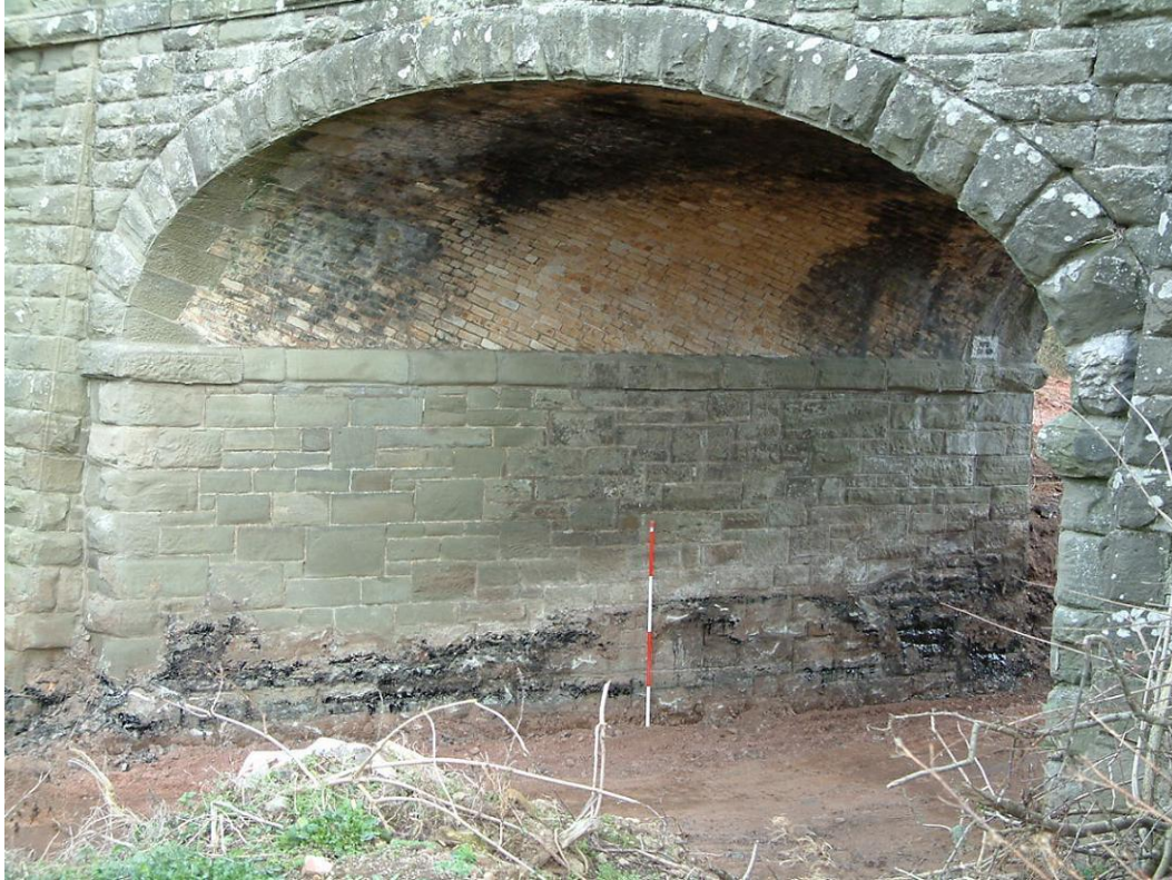
Plate 23, North buttress and spring of vaulting, view north
