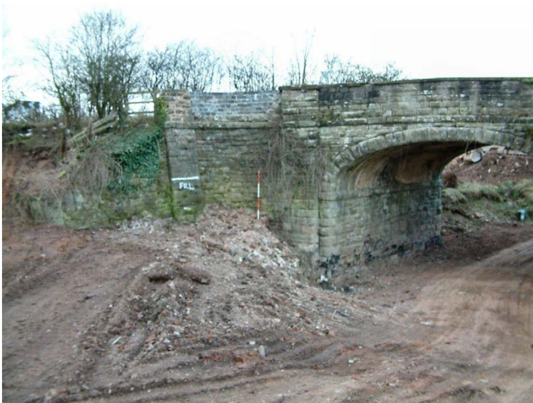
Plate 22, East elevation, north buttress, view west-south-west
