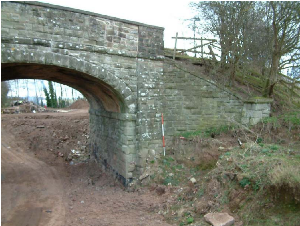
Plate 20, West elevation, south buttress, view east-south-east
