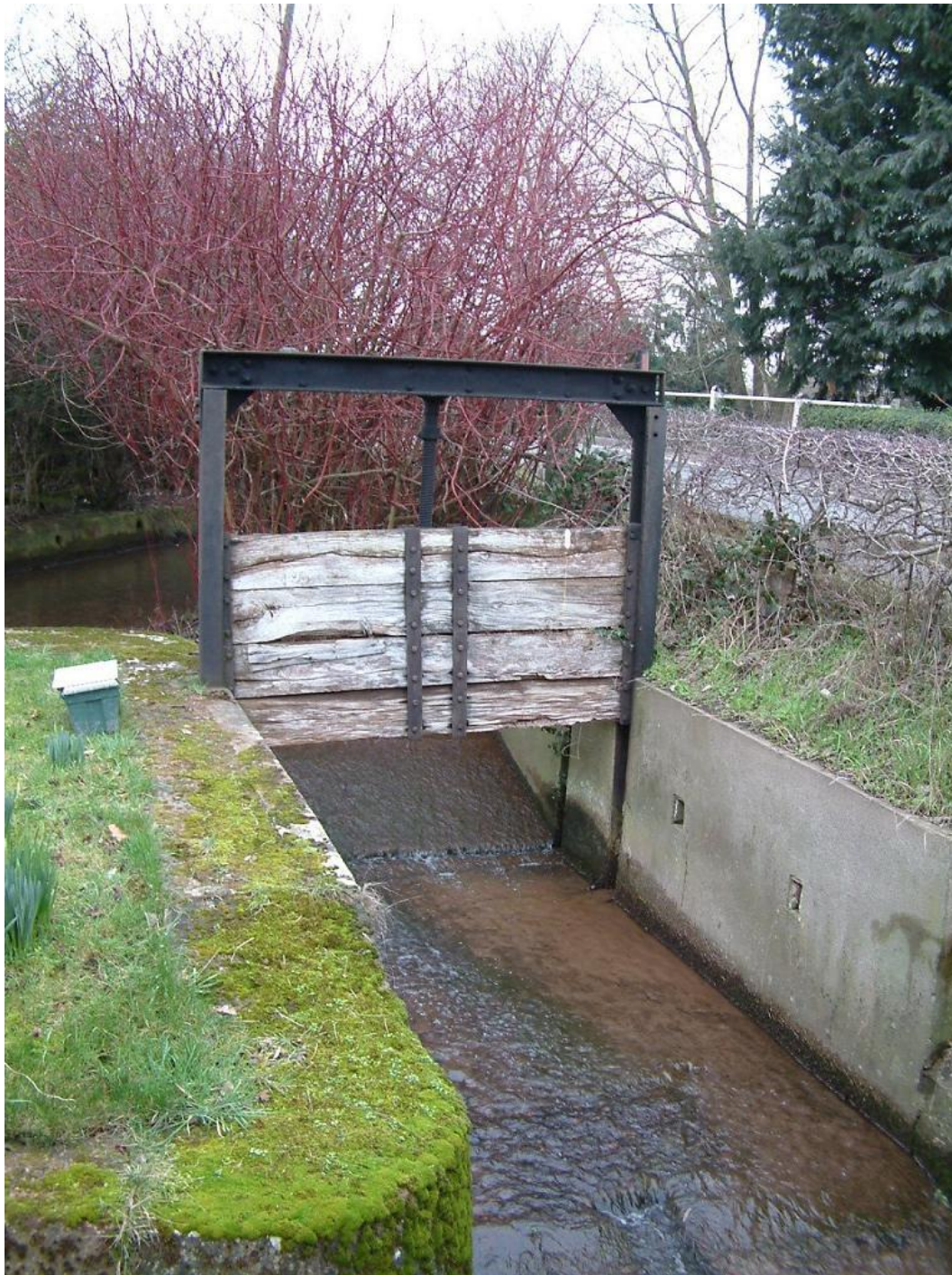
Plate 17, Sluice gate, view west
