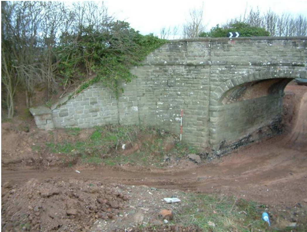
Plate 19, West elevation, north buttress, view east-north-east
