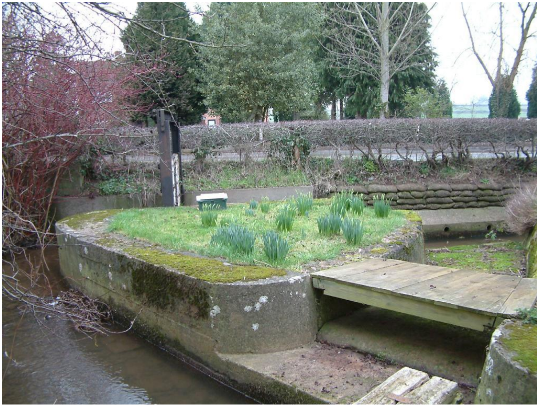
Plate 18, Sluice and leat, general view north
