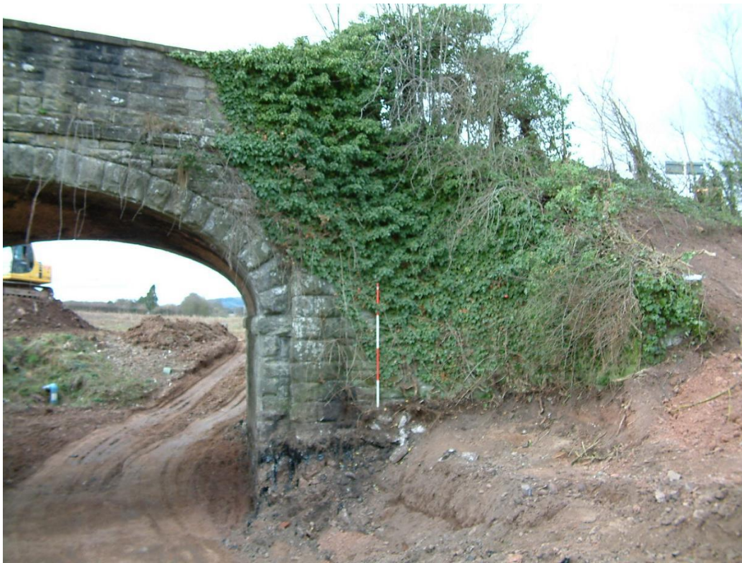
Plate 21, East elevation, north buttress, view west
