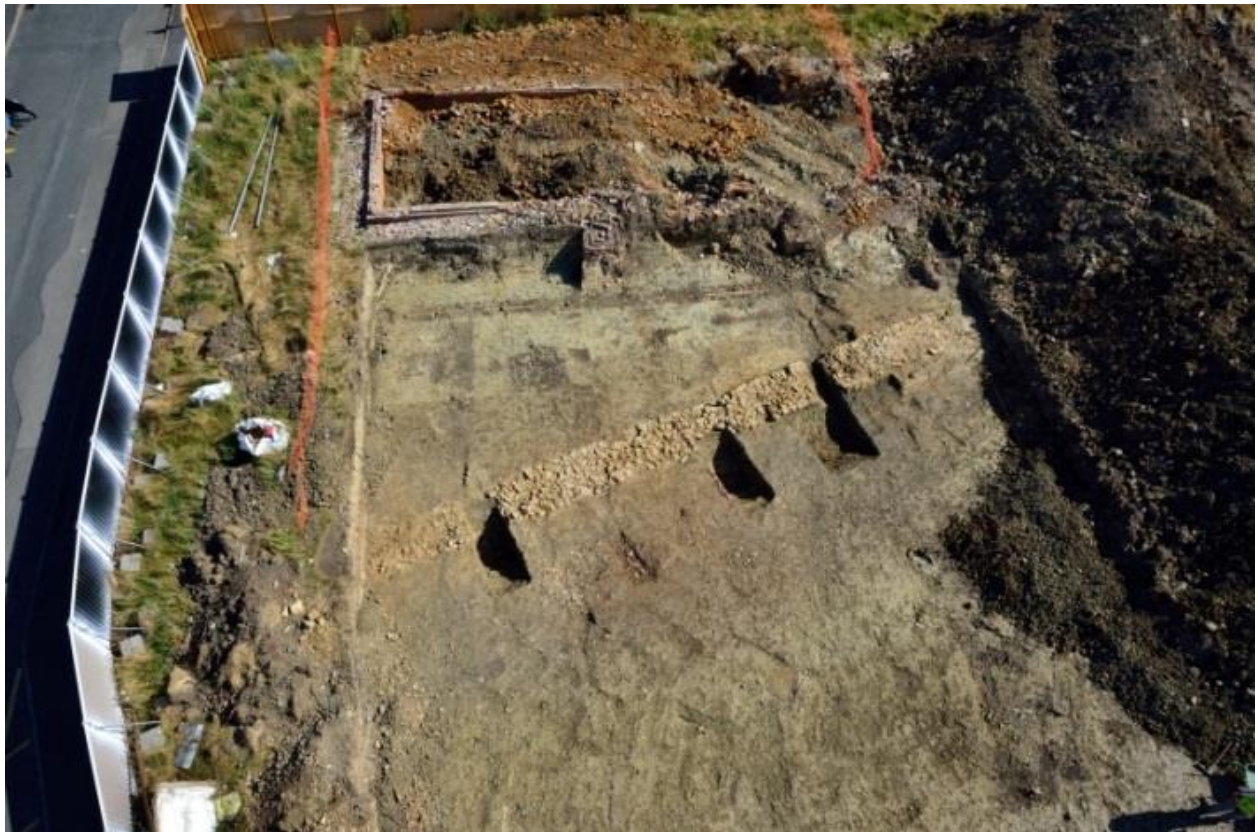
Plate 4: Aerial view of the boundary wall and Roman ditch, facing north-east (Aerial-Cam)
