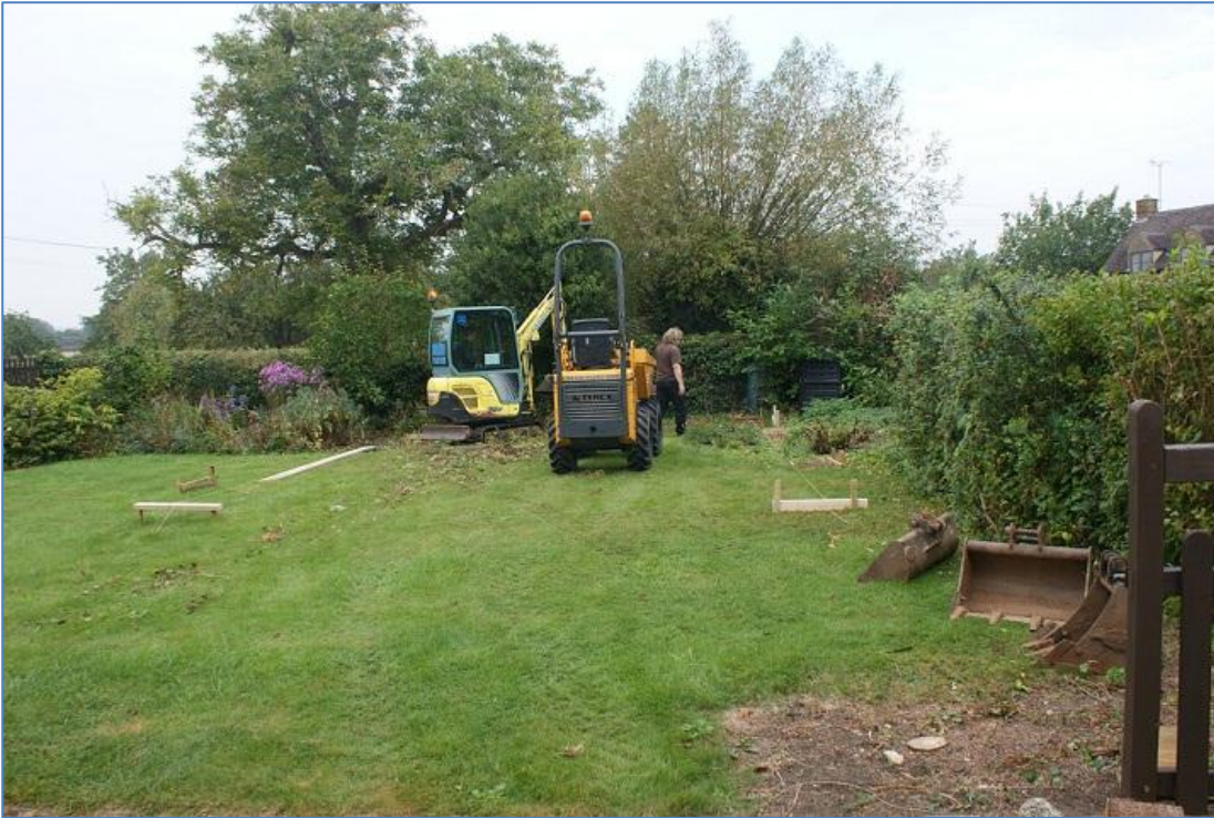
Plate 1: The site location prior to work, view west
