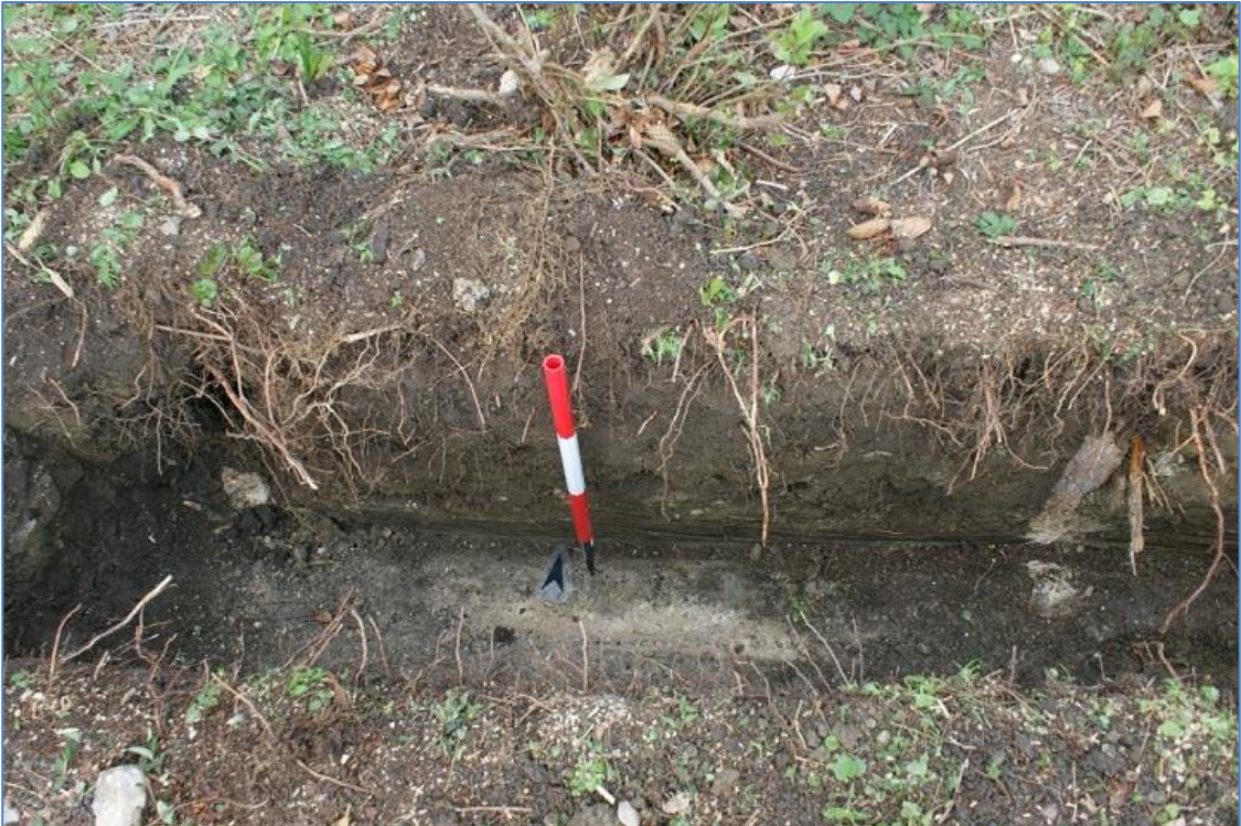
Plate 5: South-facing section showing concrete blocks in section from previous building on site
