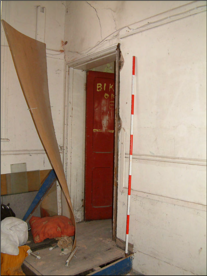
Plate 39: Door and wooden toilets area in the infants school
