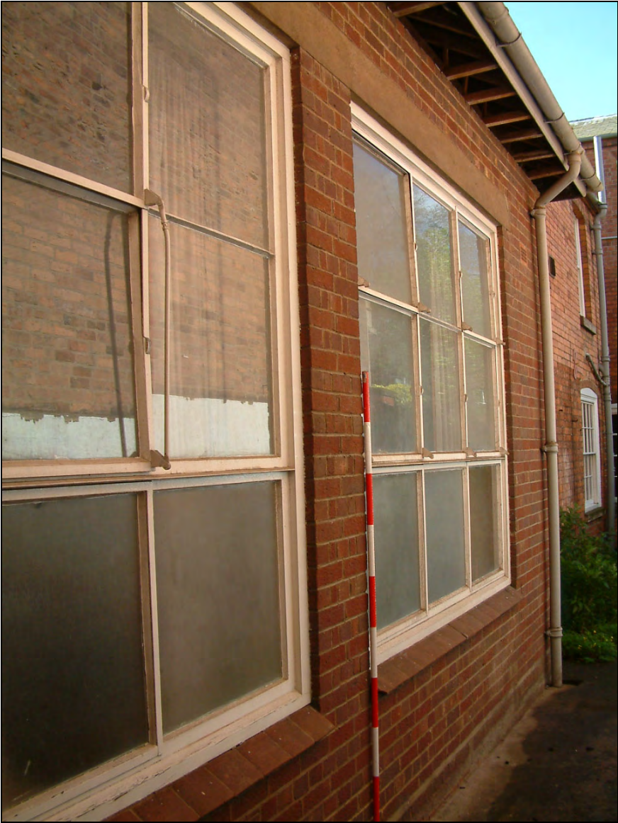
Plate 46: North elevation windows of Moran Room
