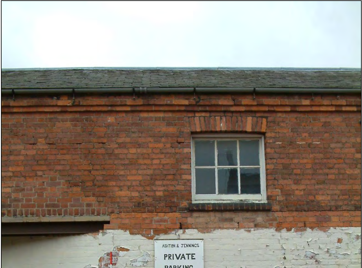
Plate 36: Example of small windows akin to stable windows
