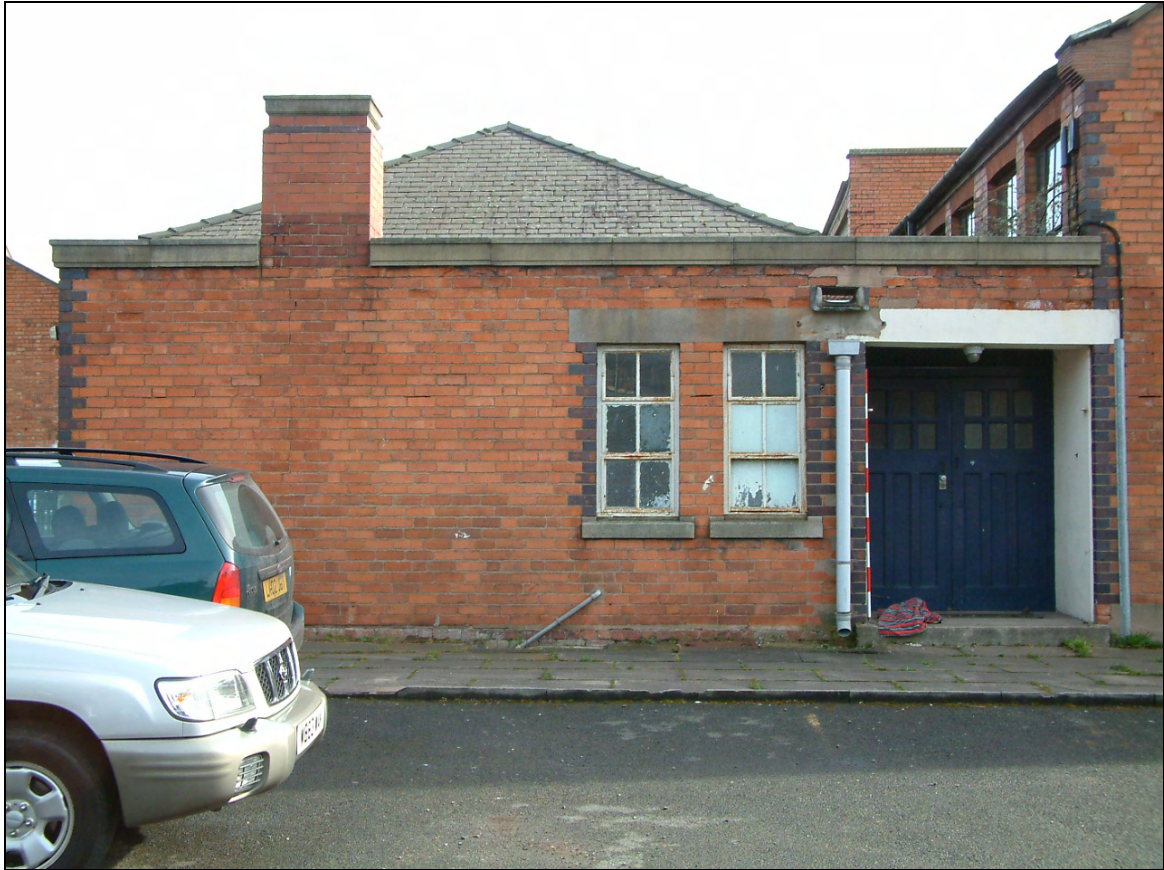
Plate 25: West elevation showing cornice on headmaster's rooms
