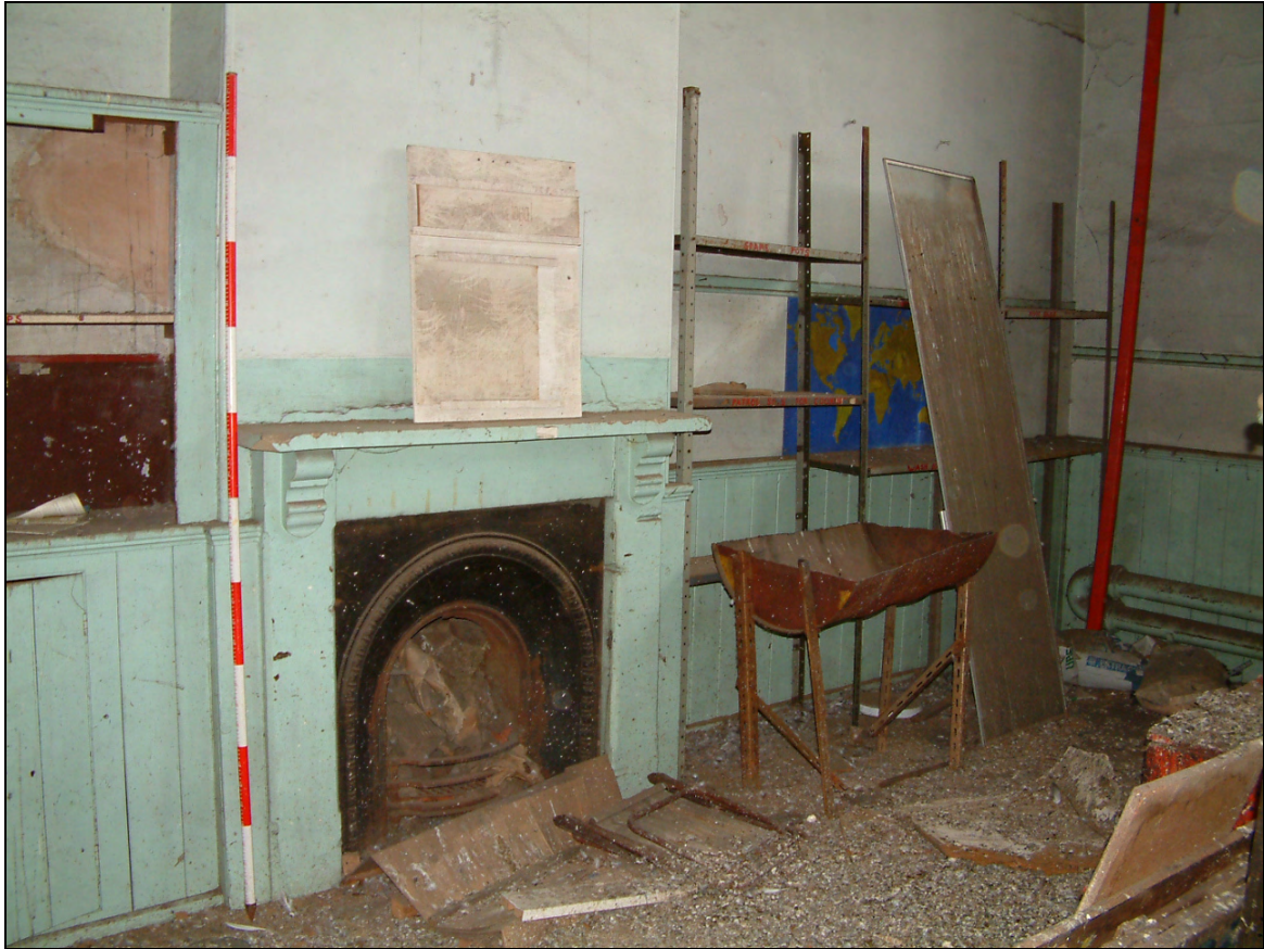
Plate 40: Dividing wall in scout hut main room
