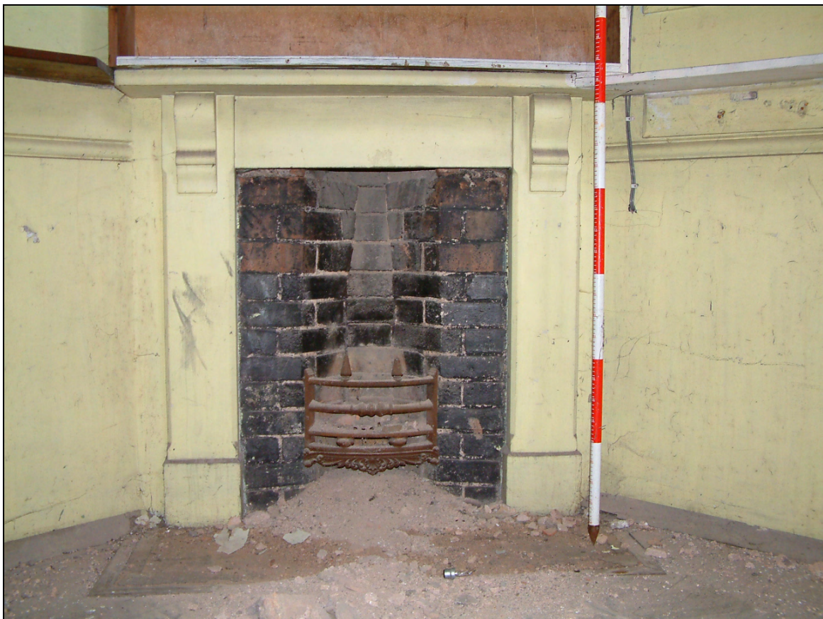
Plate 6: Fireplace in south east room of infants school
