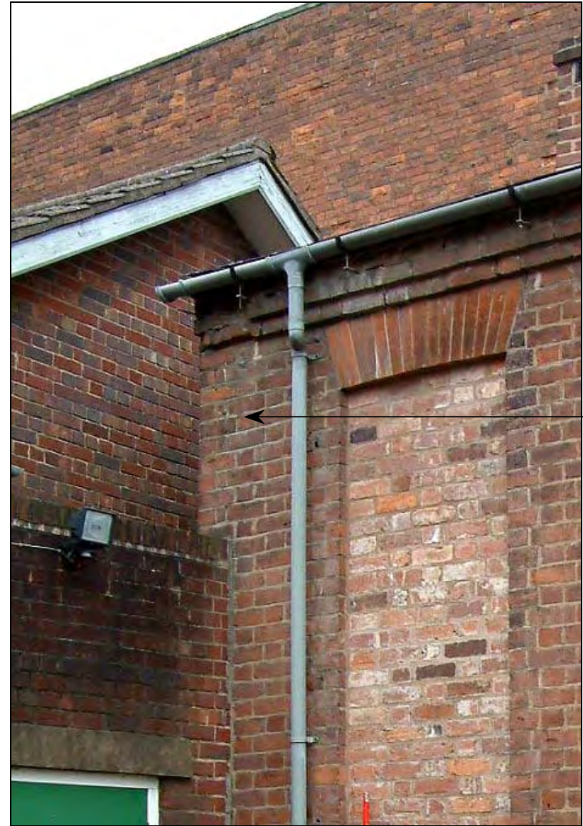
Plate 38: Evidence of possible rebuild of frontage
