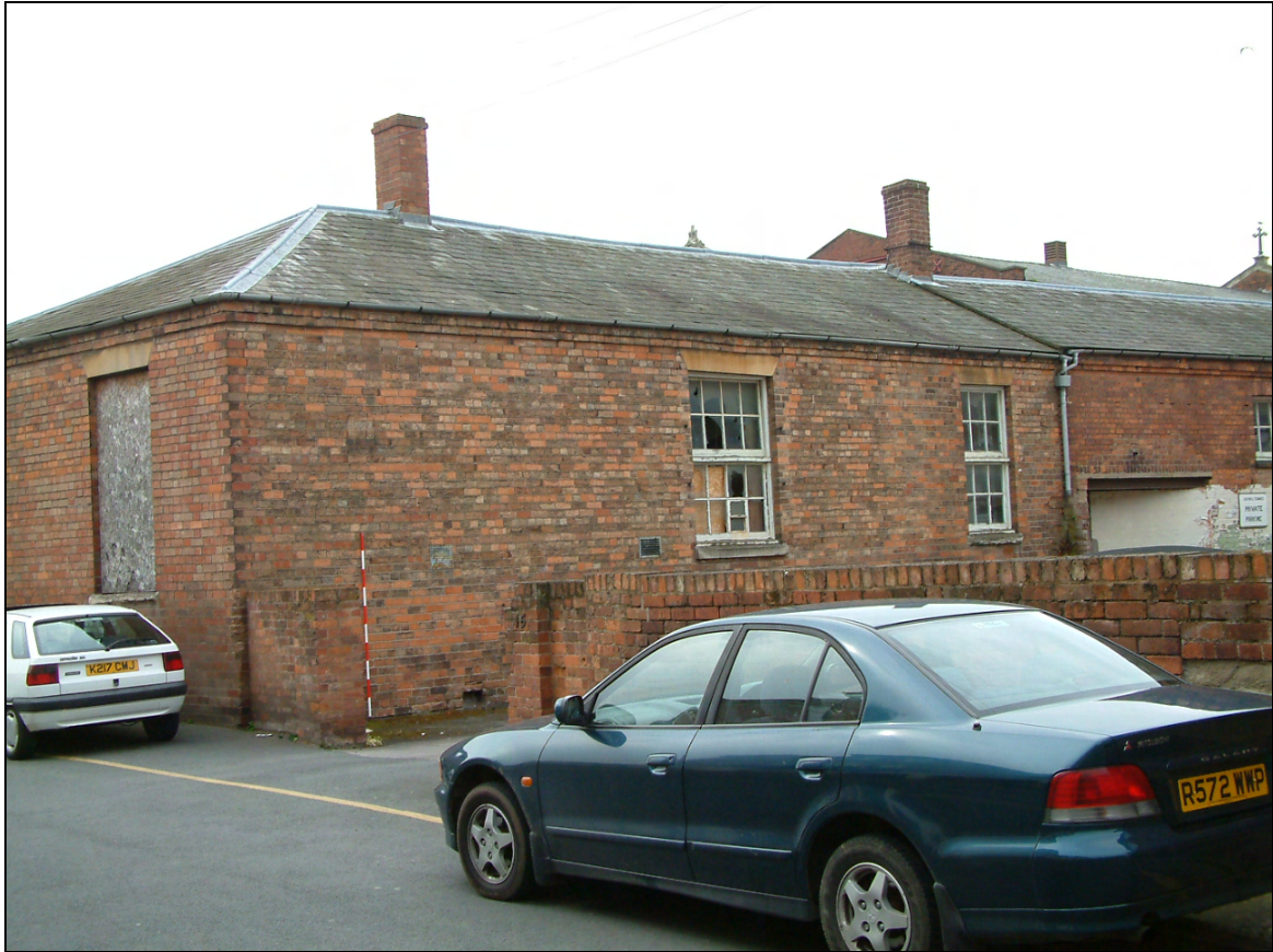
Plate 7: North elevation of old scout hut
