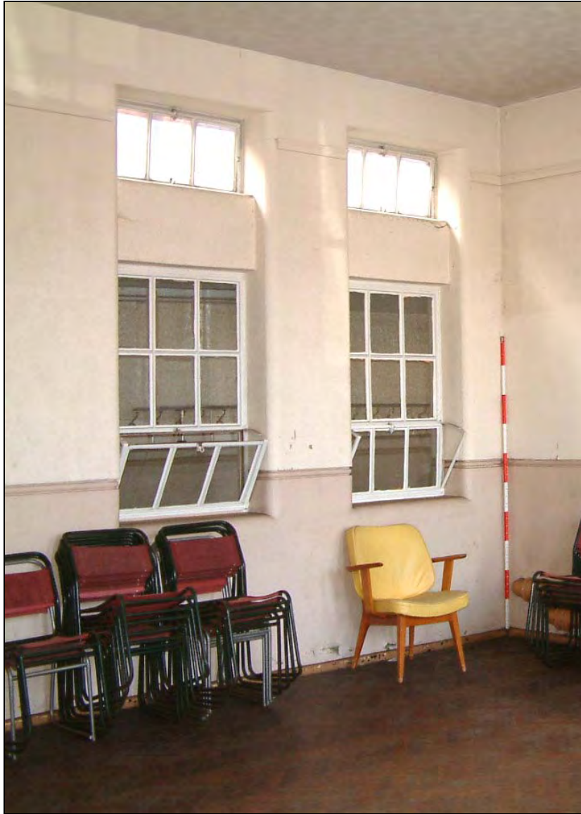
Plate 27: Internal metal frame windows opening onto corridor
