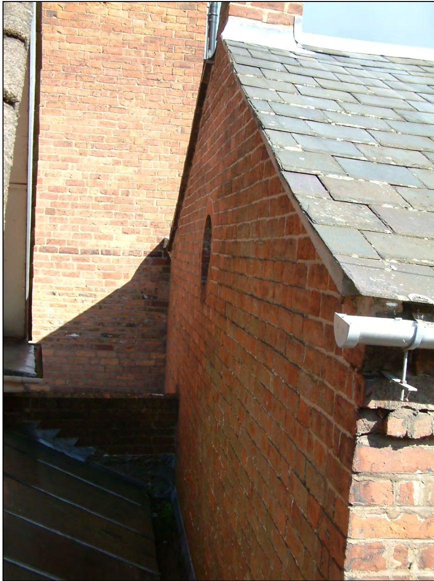
Plate 37: Pitching eye on west elevation
