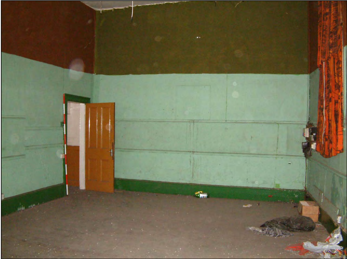
Plate 9: Interior of scout hut, east room
