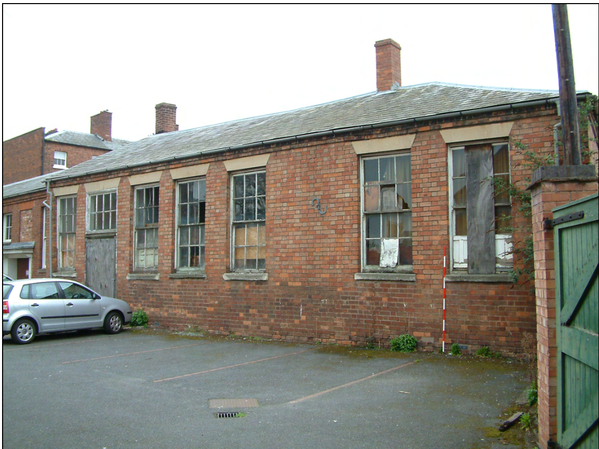
Plate 8: South elevation of old scout hut
