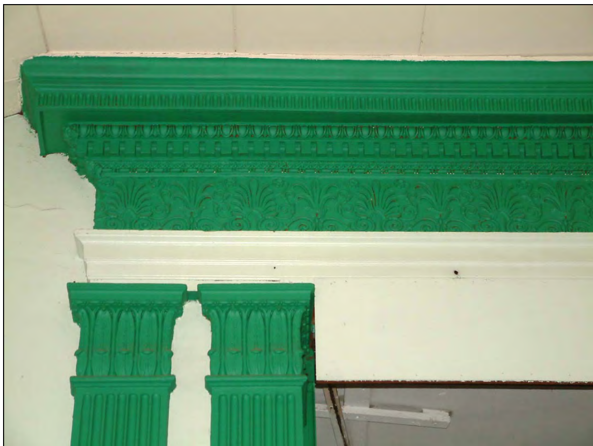
Plate 16: Plasterwork around stage in parish hall
