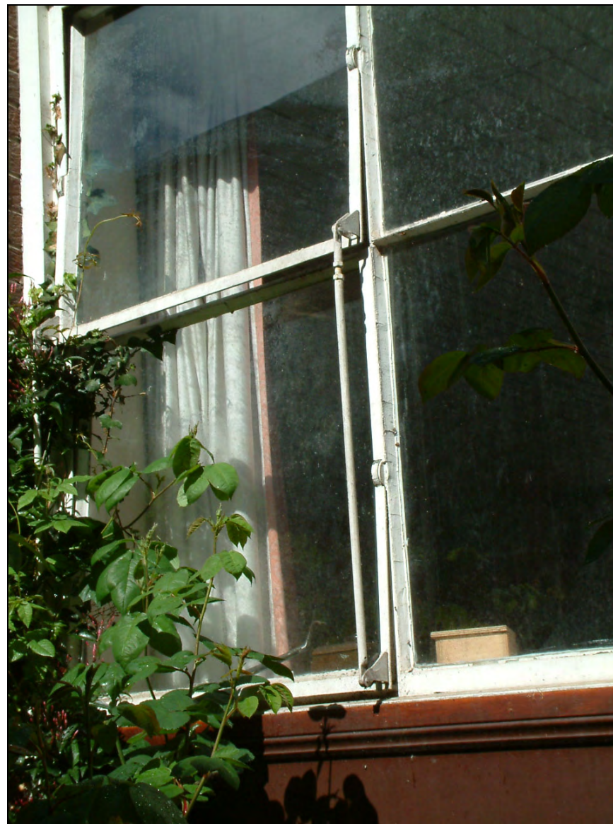
Plate 33: Example of sliding hinge to central sections of windows
