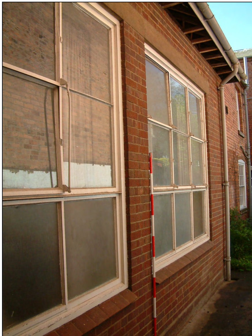
Plate 32: Metal frame windows on north elevation
