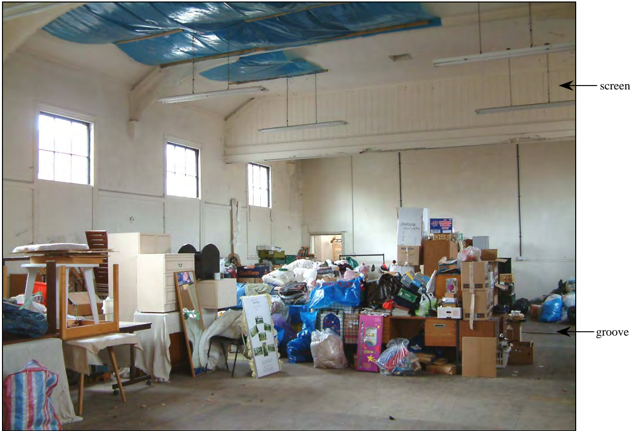
Plate 5: Infants school interior showing screen and groove for sliding partition
