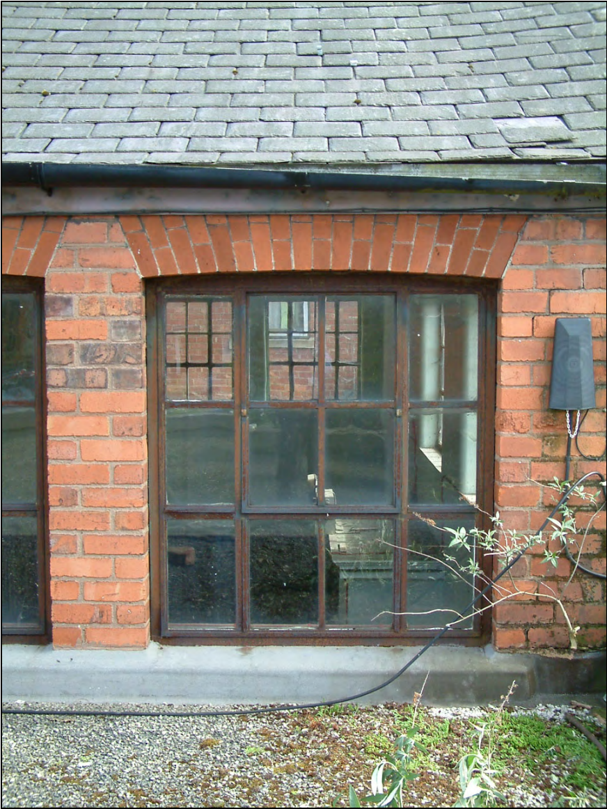
Plate 21: Metal frame window with central hinged section
