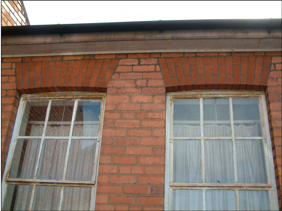
Plate 28: External metal frame windows
