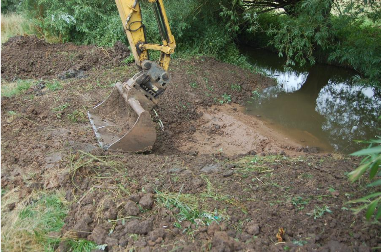
Plate 5, Watching Brief Area 3 work in progress, view north-west
