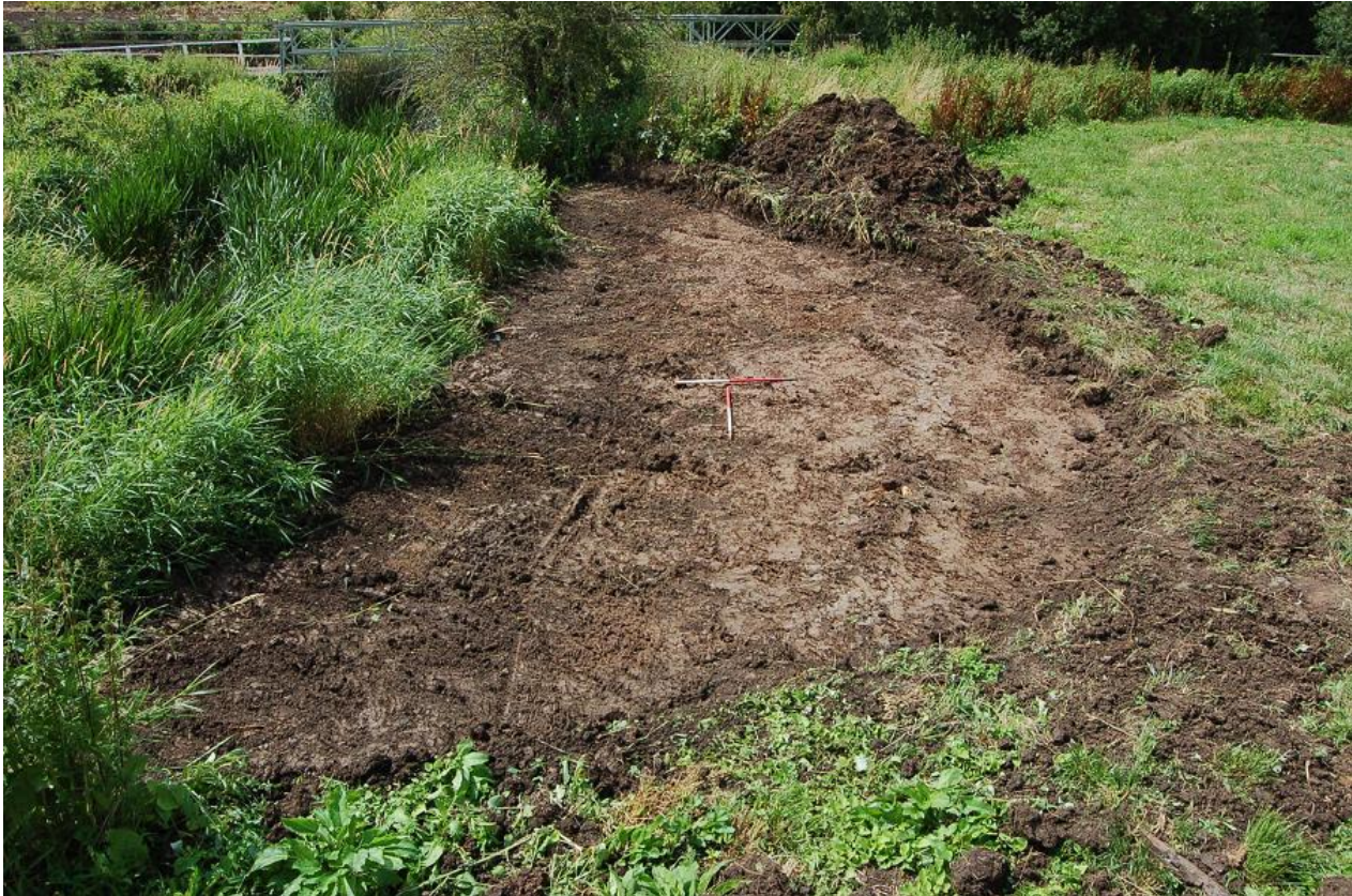
Plate 3, Watching Brief Area 1 topsoil strip complete, view west
