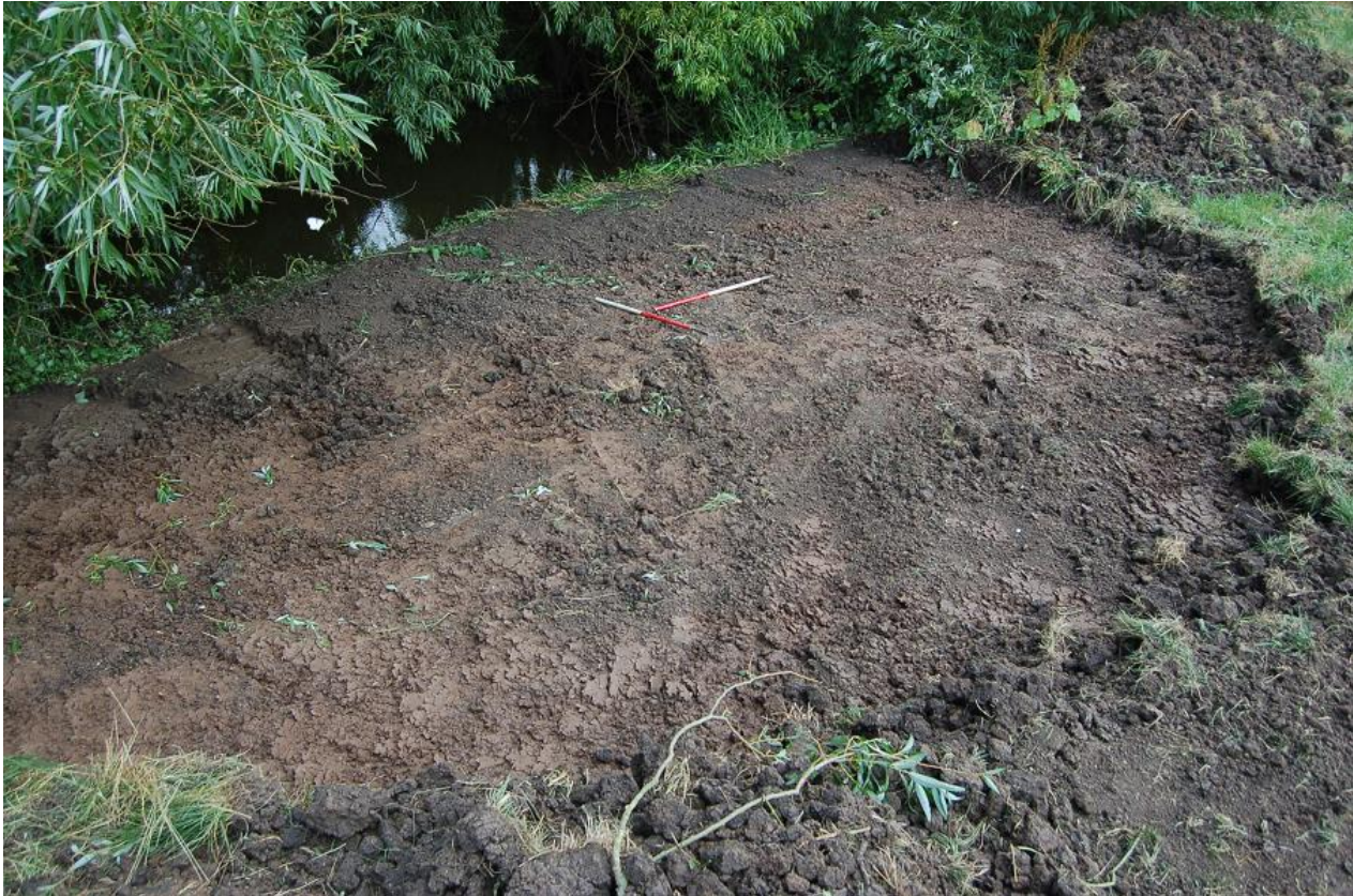
Plate 4, Watching Brief Area 2 topsoil strip complete, view east-north-east
