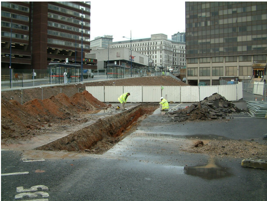
Plate 5: Trench 3, general view of trench, looking west
