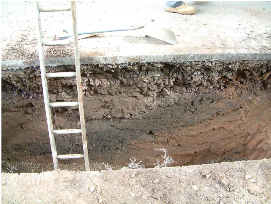
Plate 3 South side of ditch 308, facing east.
