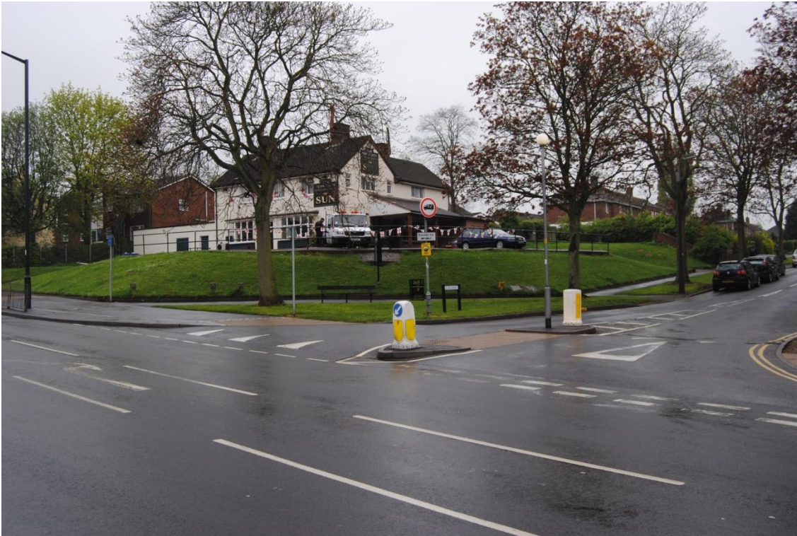
Plate 1: The Sun public house occupies the north-eastern part of the site
