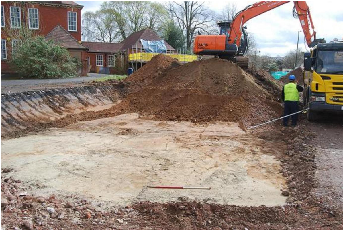
Plate 1 The deepest area of Trench 1, excavated to natural sand (101), view south-east
