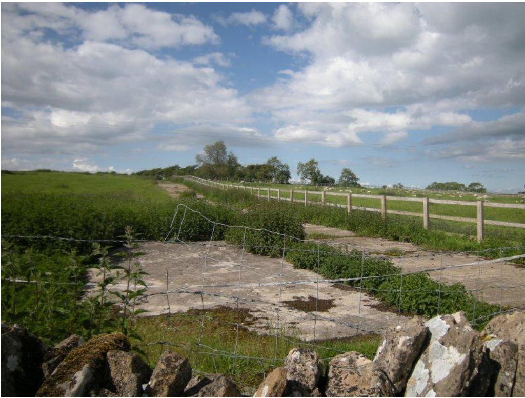
Plate 9 Looking north-west along concrete trackway
