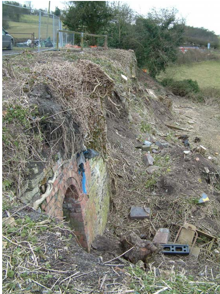
27. Lime kiln bank, general south-east view of bank, as exposed
