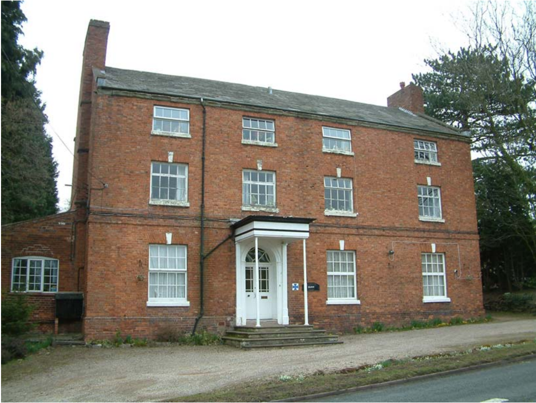
9. Plymouth House, south-west elevation
