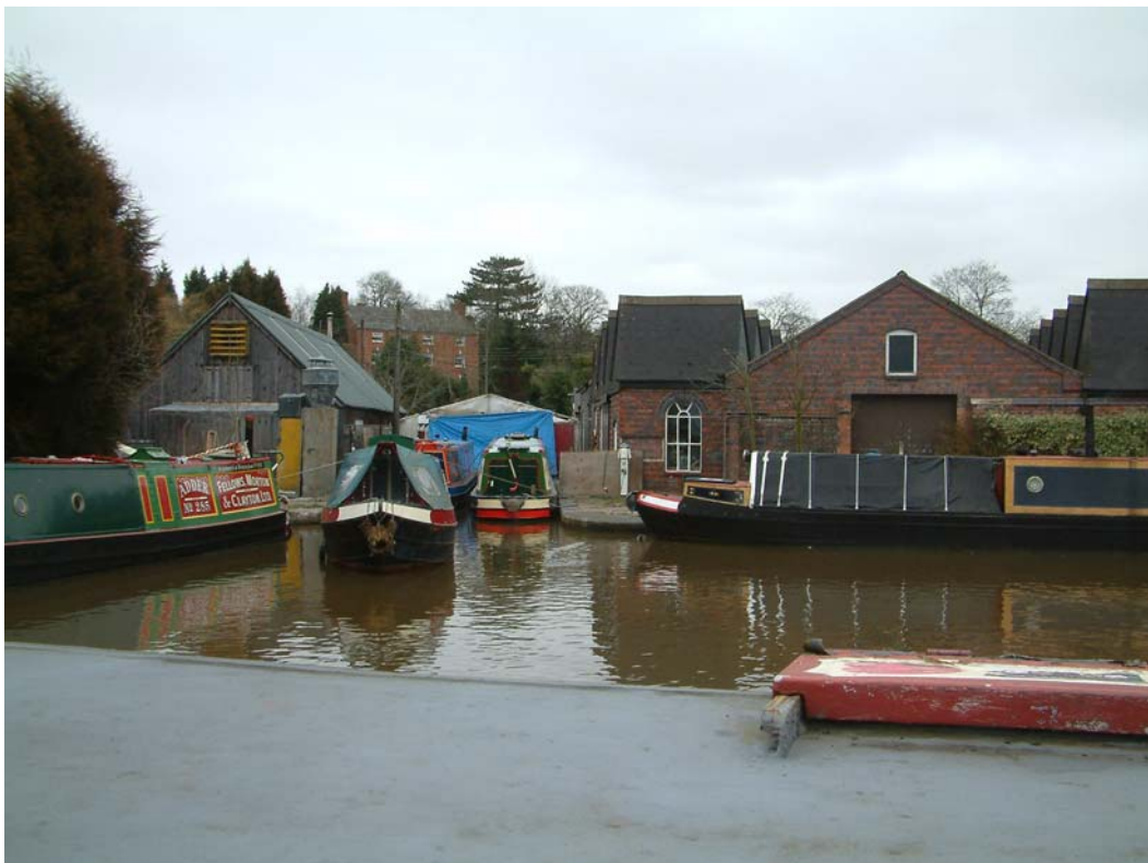
24. Canal sluice arm and wooden workshop, view north-east
