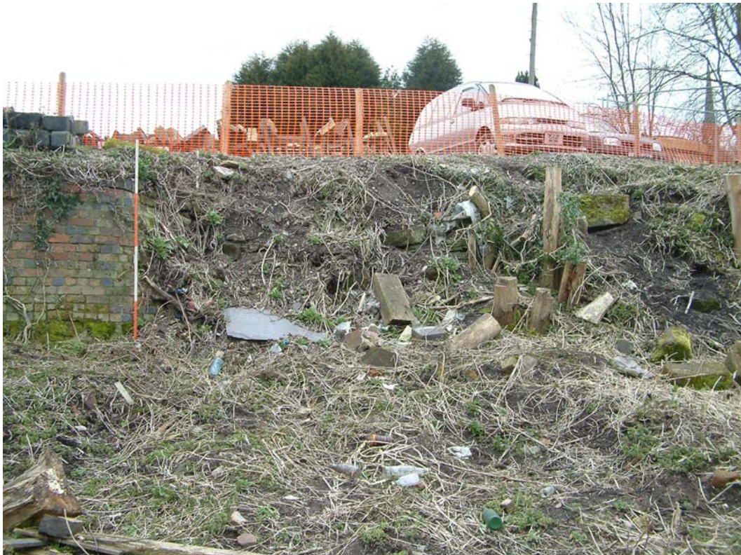
30. Kiln 1, probable location (collapsed), view south-east
