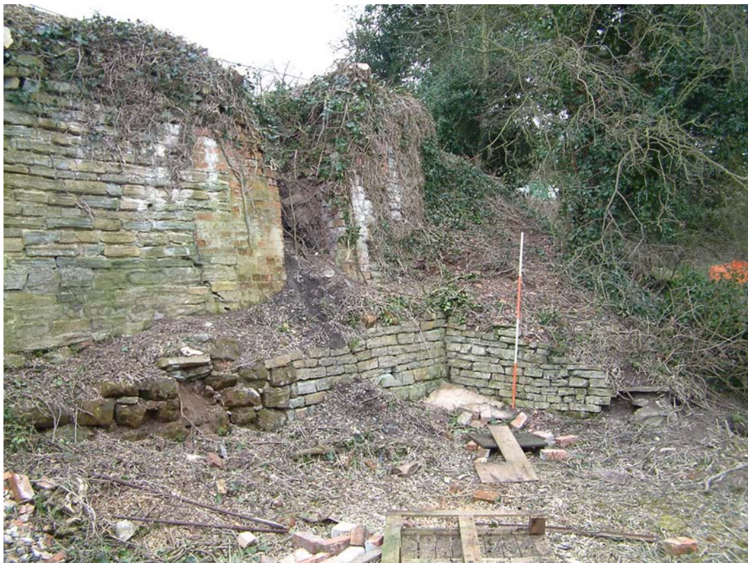
36. Kiln 5, external retaining wall and abutment, view south
