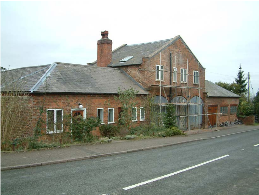
6. Plymcot, former Plymouth Inn coaching house and stables, north-east elevation
