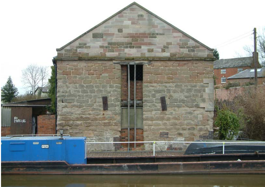
4. Stone warehouse, south-east elevation
