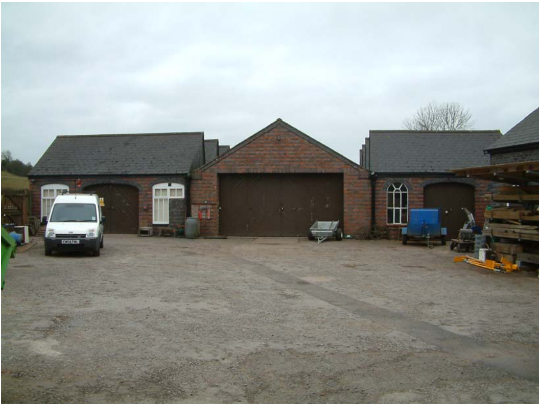
18. Sharpness New Docks workshop, north-east elevation
