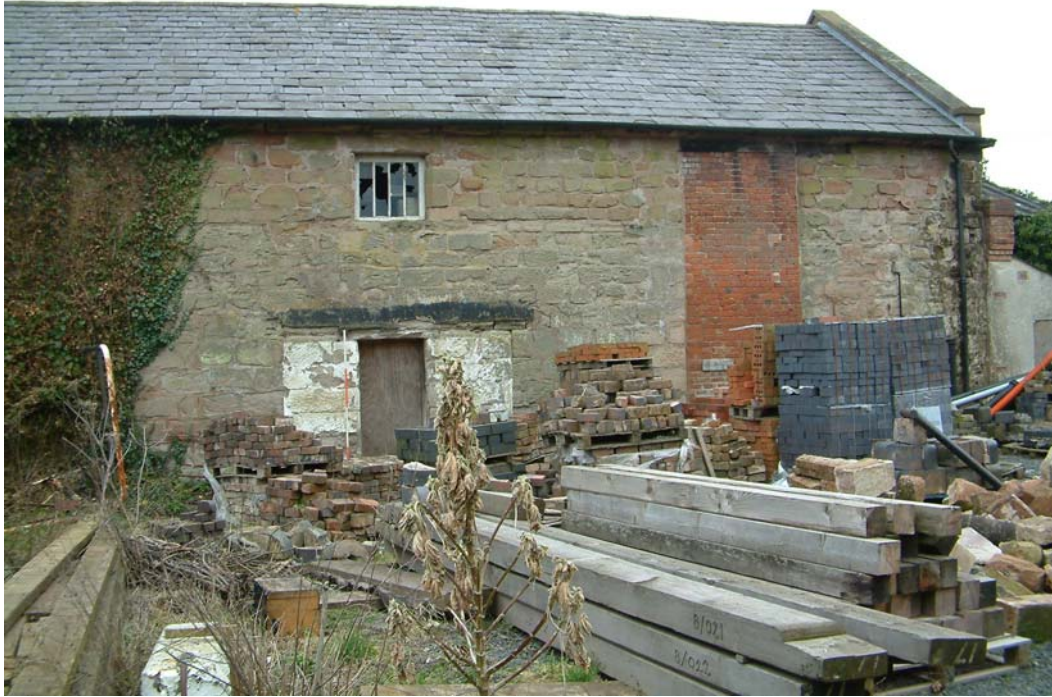
3. Stone warehouse, north-east elevation
