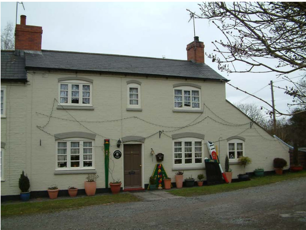
12. Former weigh house, 1, New Wharf Cottages, and site of weighbridge, south-east elevation
