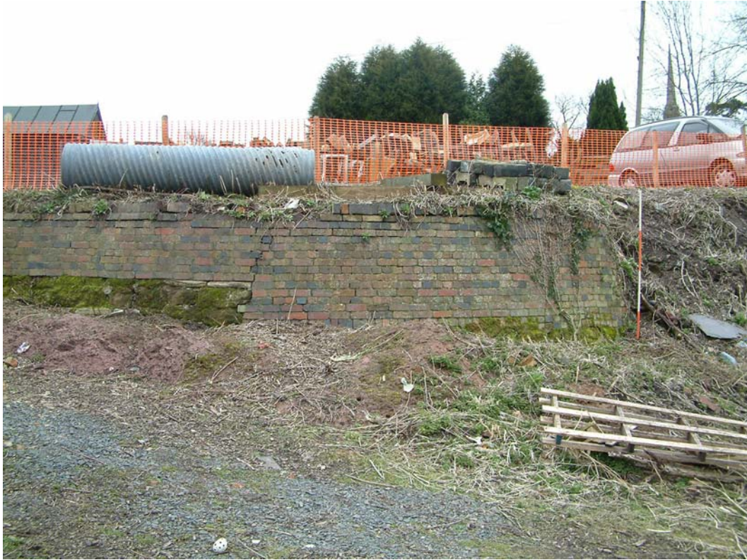
29. Kiln bank façade, north-west end, view south-east
