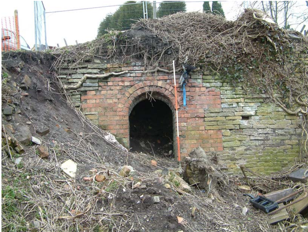
31. Kiln 2 draw hole, view south-west
