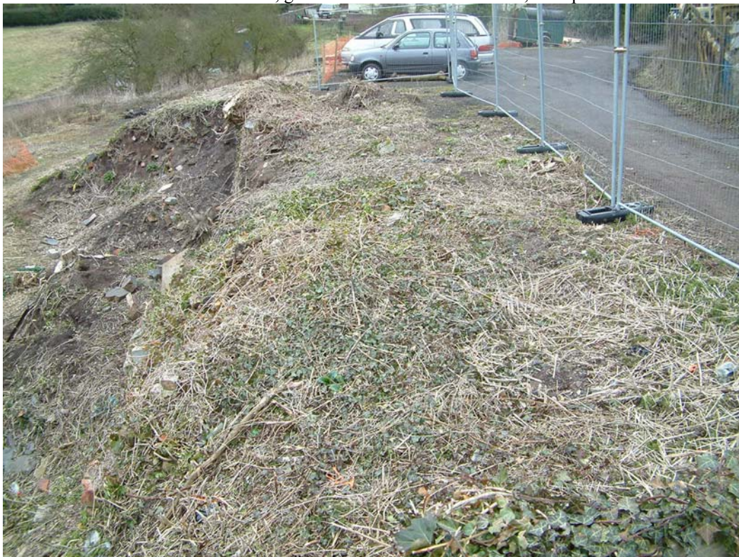
28. Lime kiln bank, general north-west view of flues, as exposed
