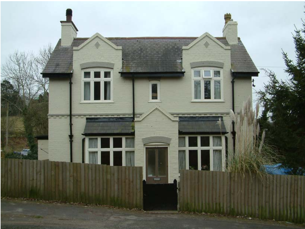
10. Superintendent's house, north-east elevation
