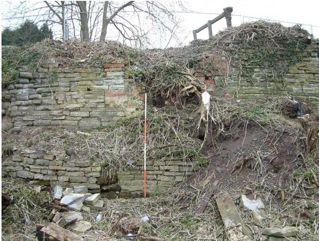
33. Kiln 3 and external retaining wall, view south-east
