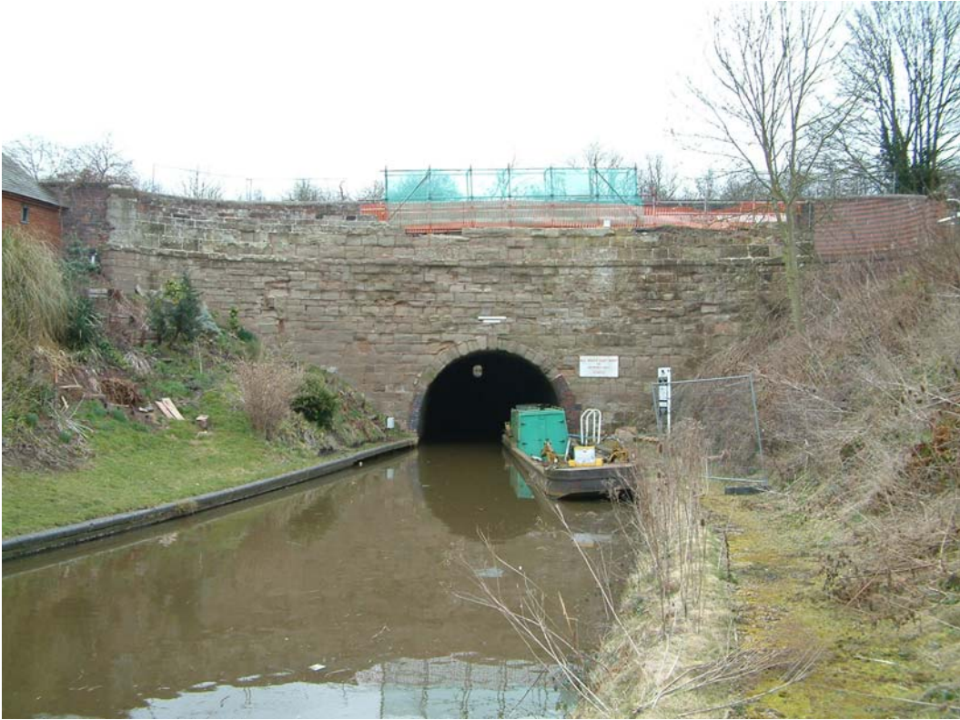
5. Tunnel portal, south-east end
