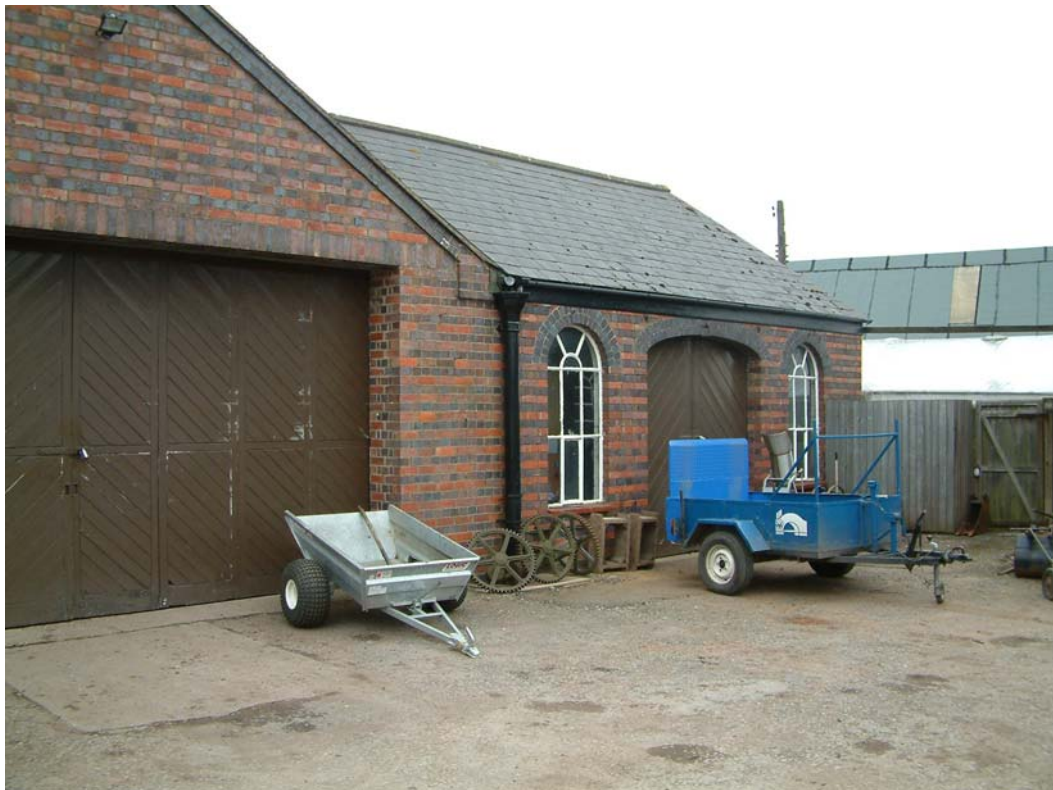
20. Sharpness New Docks workshop, north-east elevation, north-west side
