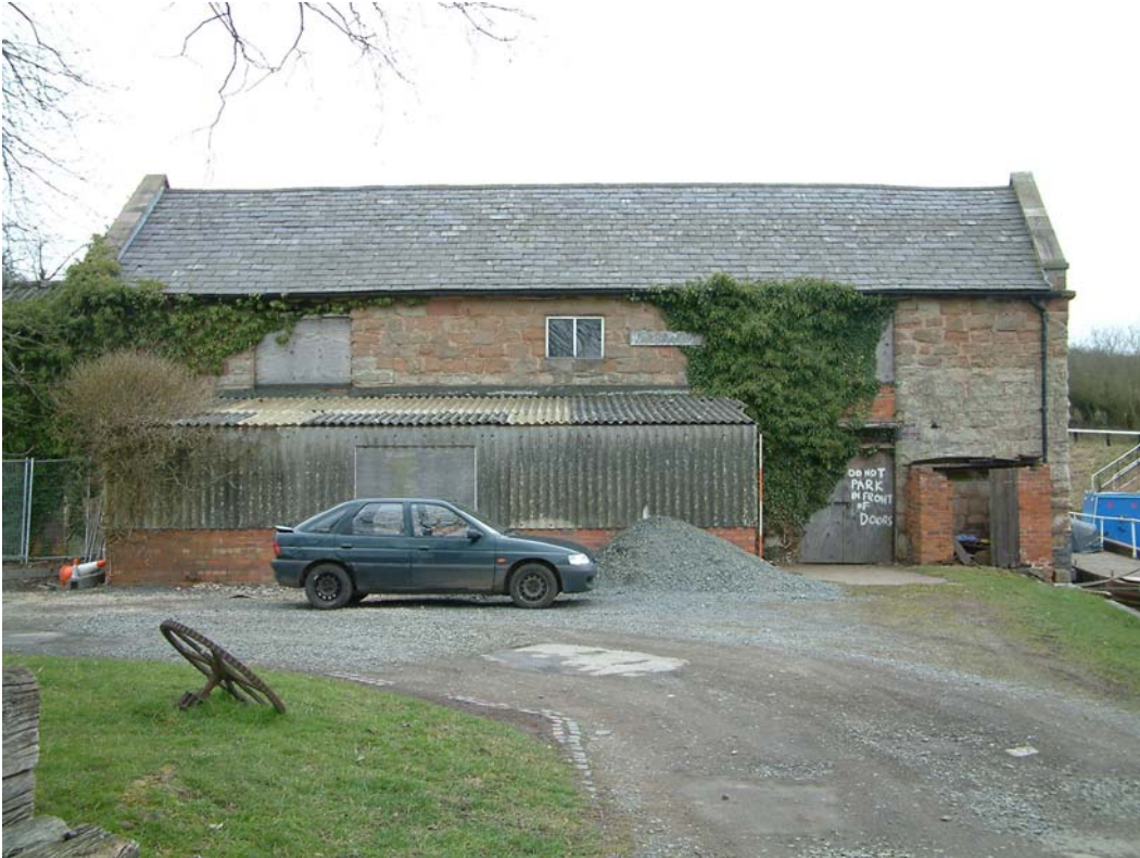
1. Stone warehouse, west-south-west elevation
