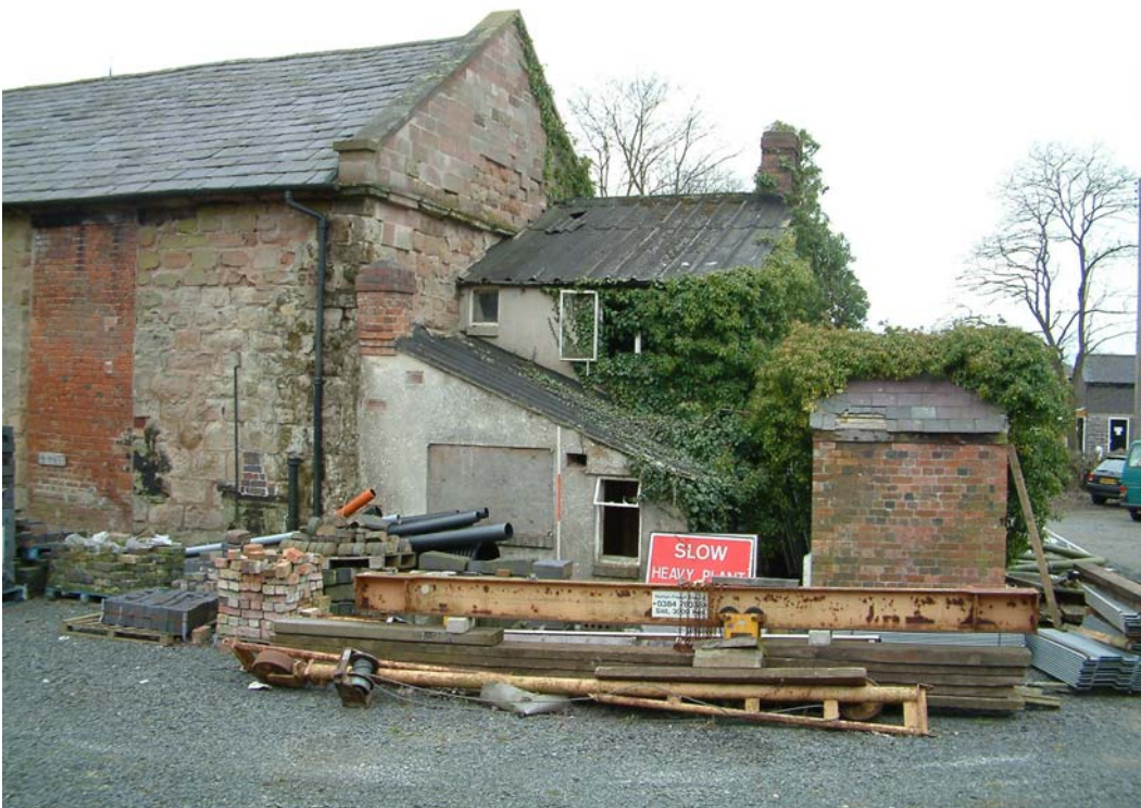
2. Stone warehouse and wharfingers cottage, north-east elevation
