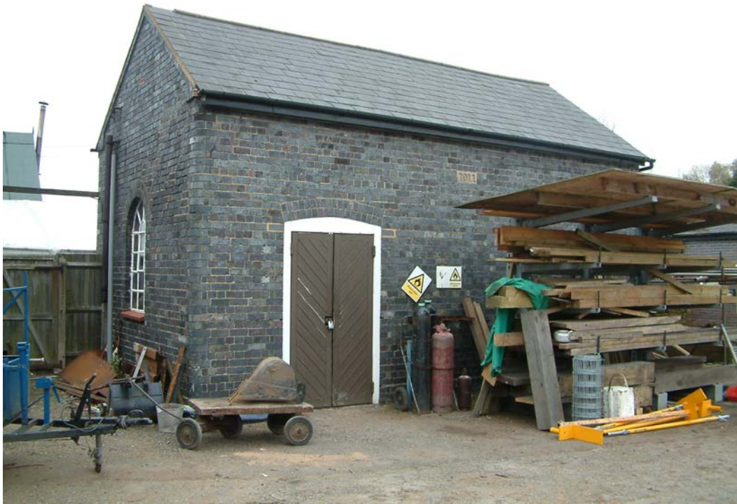
21. Sharpness New Docks blacksmith's shop, south-east elevation
