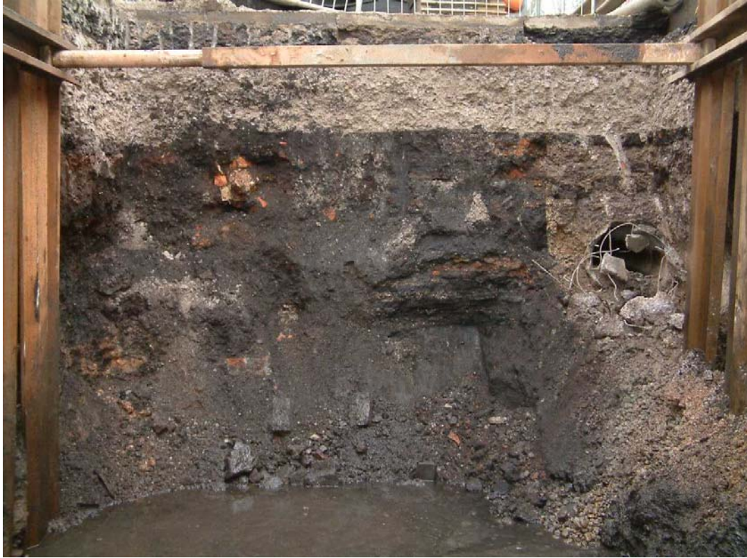
Plate 7: Trench in progress - general stratigraphy - east end - east view
