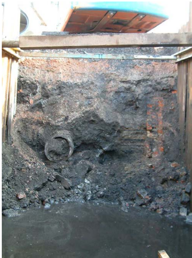
Plate 4: Trench in progress - existing sewer pipe and wall [120] - view east
