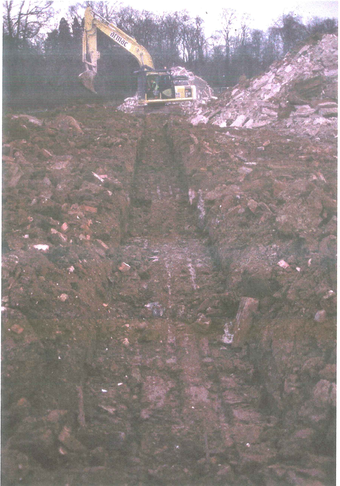
Plate 3: Block 6 demolition phase, looking north.
