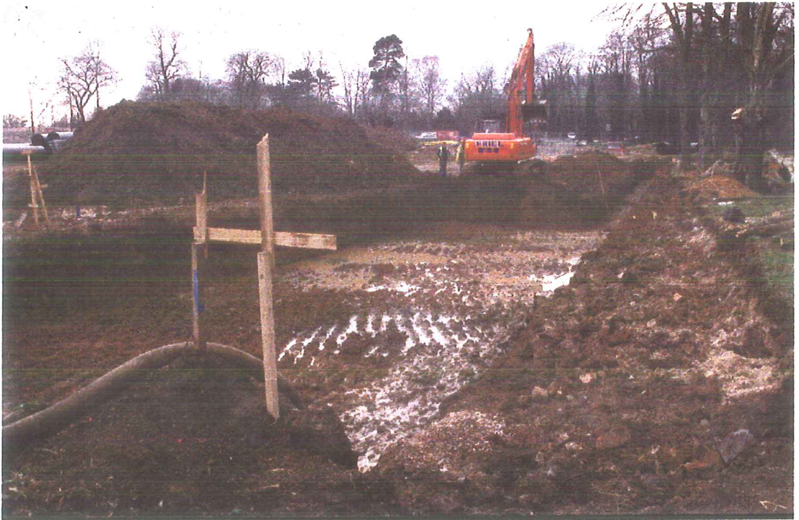
Plate 1: Water tank trench looking west.
