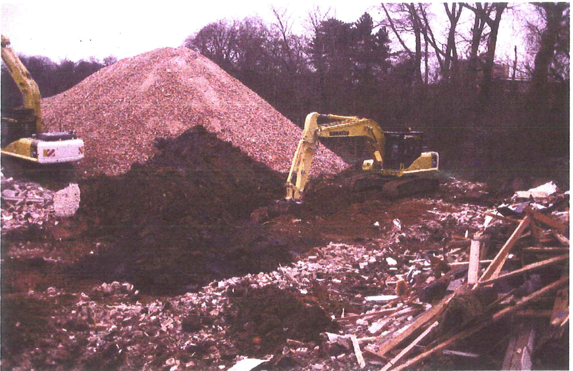
Plate 2: Block 22, working shot looking west.
