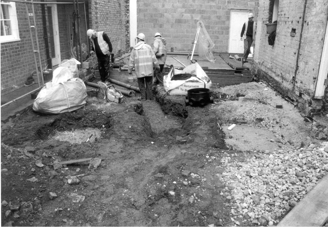
Plate 5: Area of groundworks, looking east.
