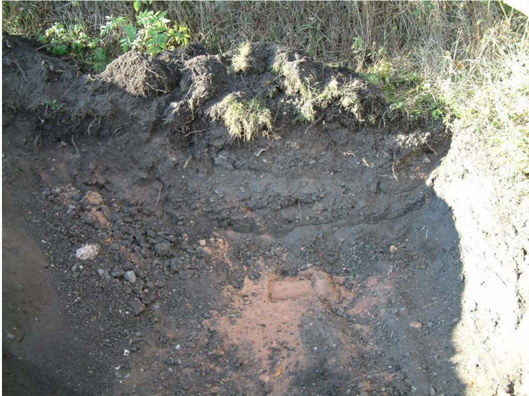
Plate 1: Brine pipe junction in Trench 1
