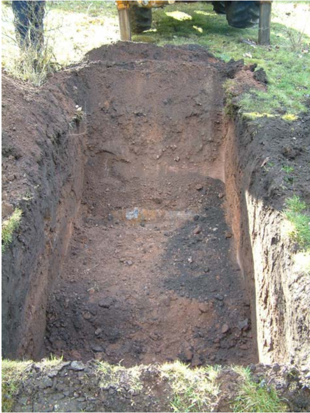
Plate 3: Brine pipe located in Trench 3
