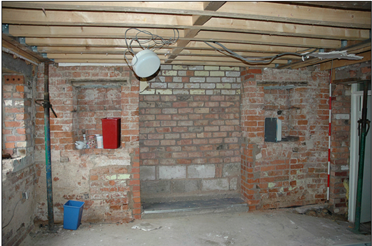
Plate 13: Ground floor, room 16, of original phase building, inglenook added c1825
