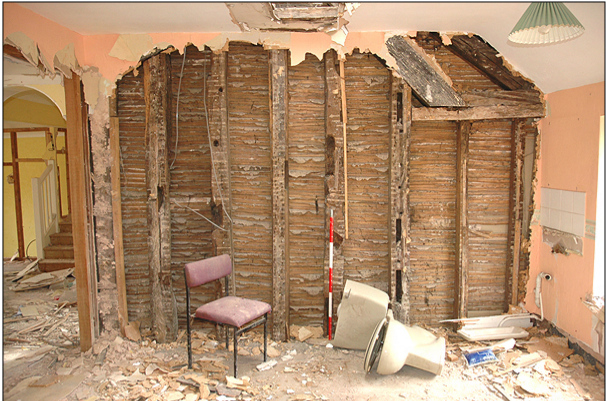
Plate 11: Room 20 showing c1825 stud partition with reused timbers
