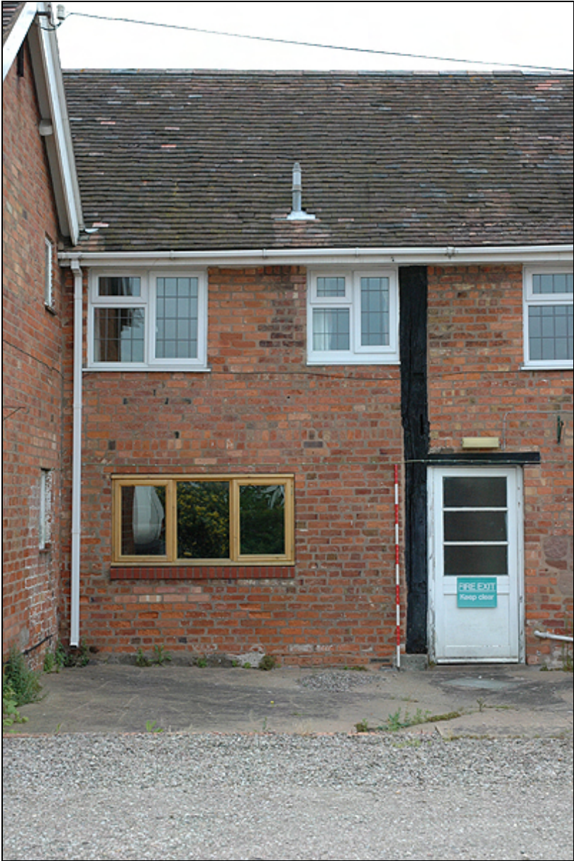
Plate 2: West elevation of Moat House showing timber post and rail
