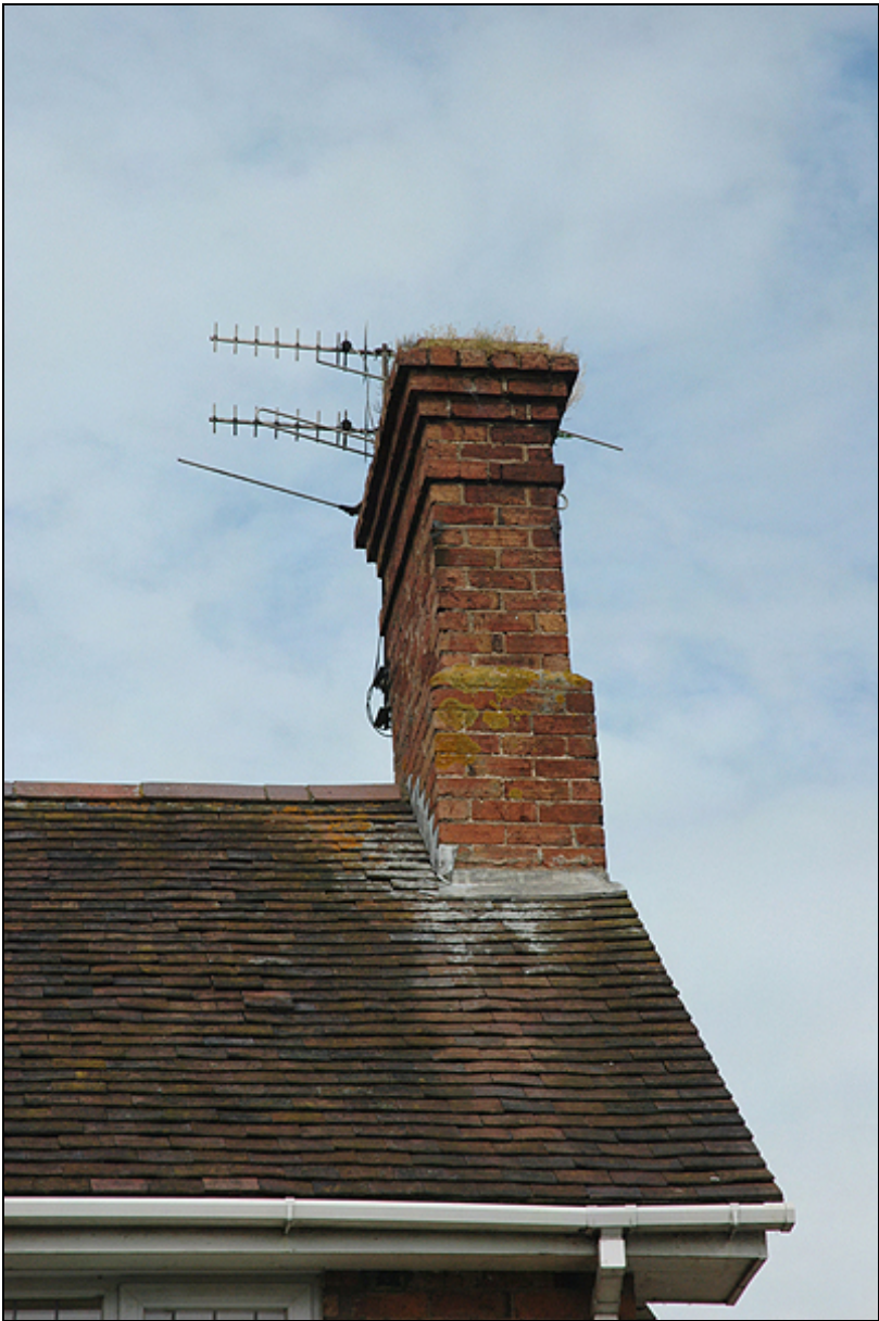
Plate 19: Chimney stack at rear of c1875 extension
