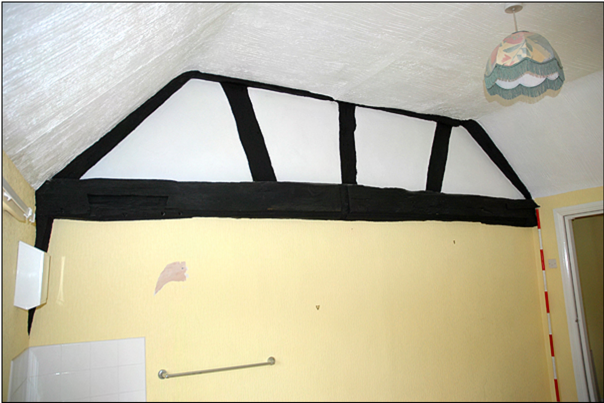
Plate 4: First floor, room 22, timber-frame
