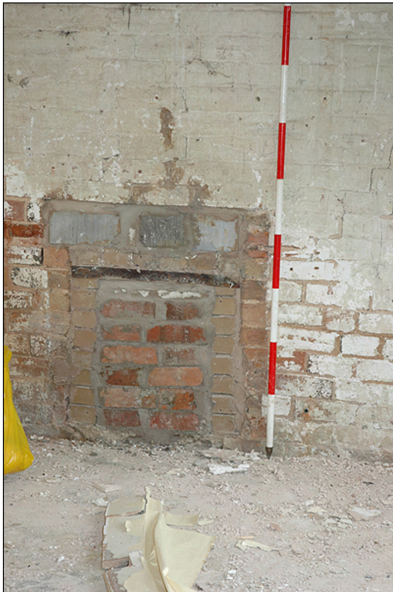
Plate 8: Position of hearth on interior of c1800 building
