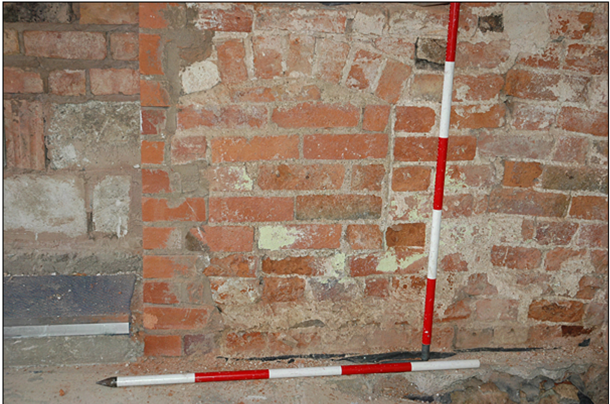
Plate 15: Bread oven on east side of inglenook
