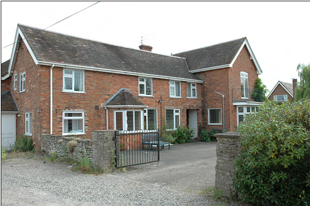
Plate 1: Moat House from the south west
