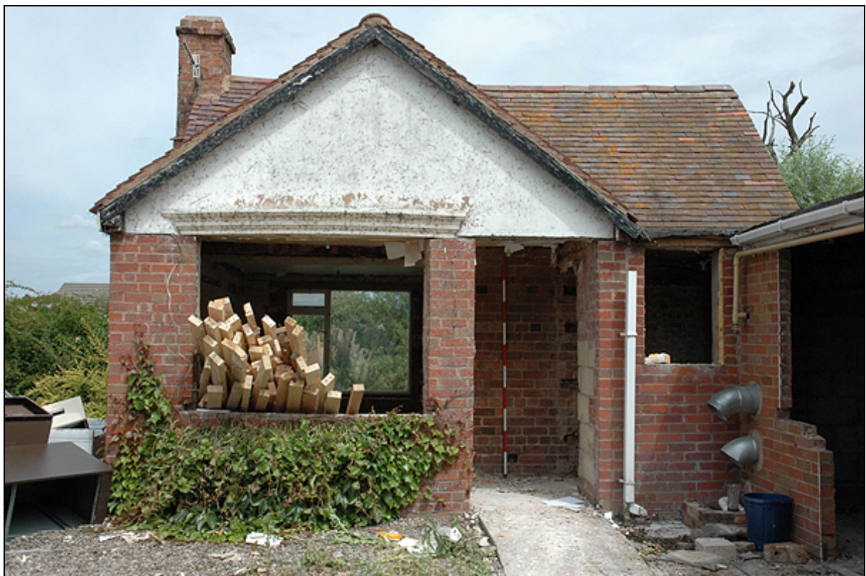
Plate 21: Bow window on extension of former stable
