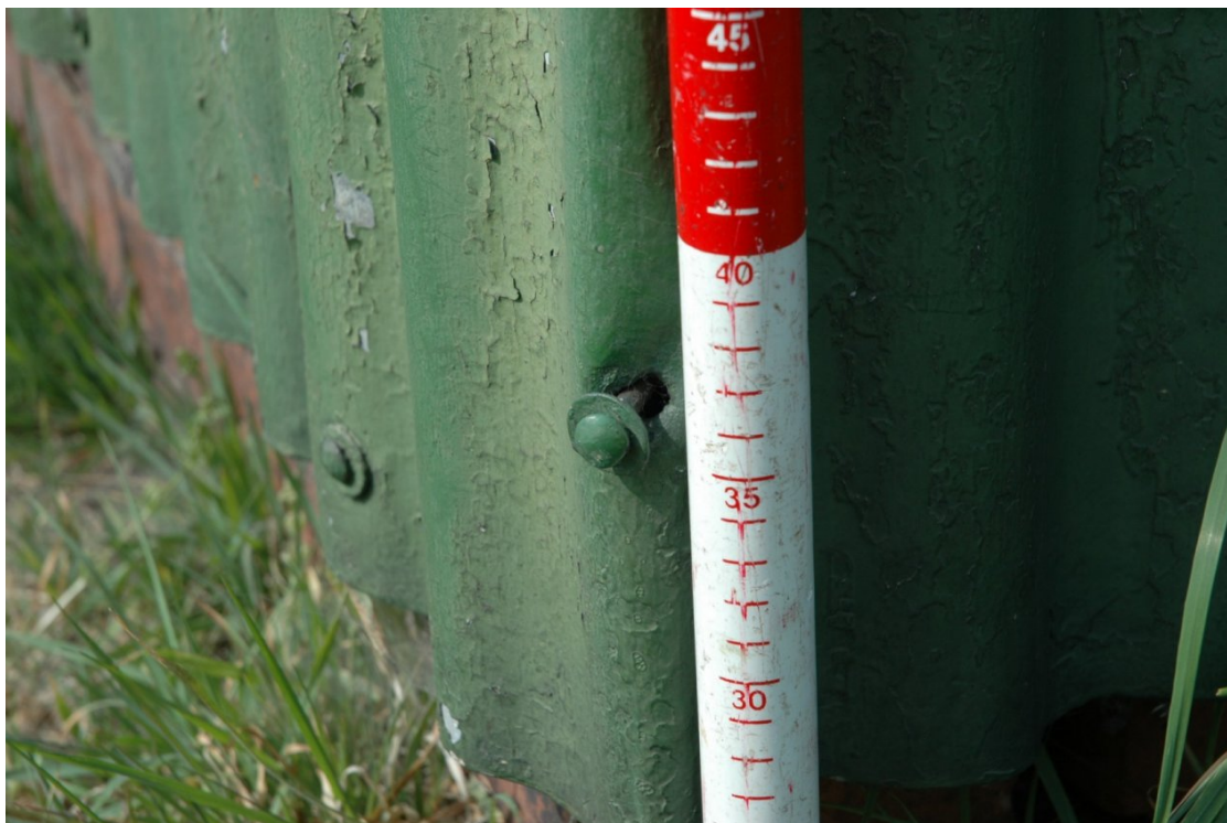
Plate 6 Fixing for sheets
