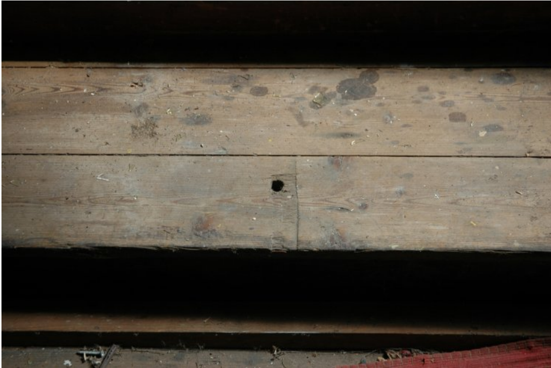
Plate 30 Bolt hole in alcove floor
