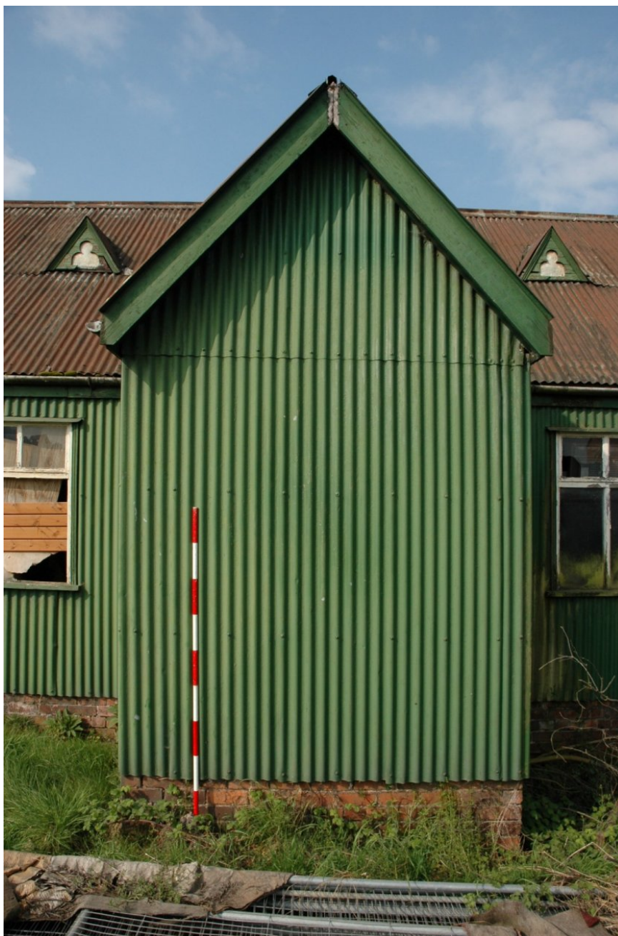
Plate 5 Example of sheeting for gable ends, from east
