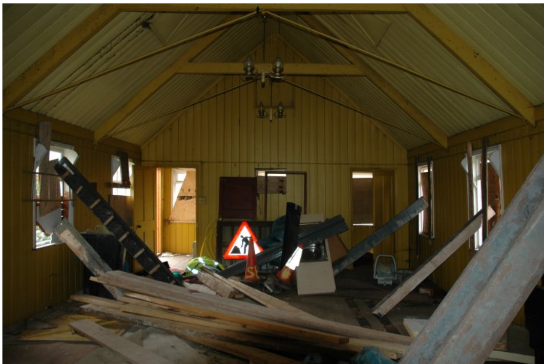
Plate 24 Triangular boards in ceiling covering ventilation holes (top, facing south)
