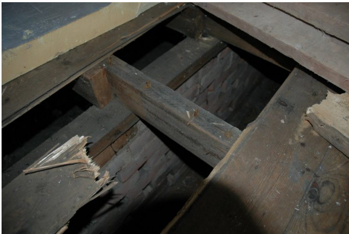
Plate 19 Joists supported on brick plinth
