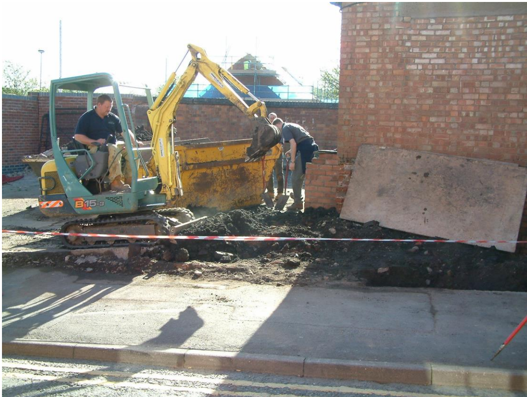
Plate 1: Commencing groundworks at western end, facing east
