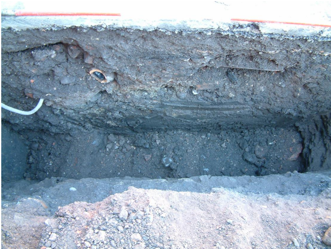
Plate 3: Section 1, facing west
