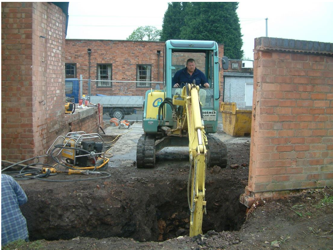
Plate 2: Commencing groundworks at eastern end, facing west
