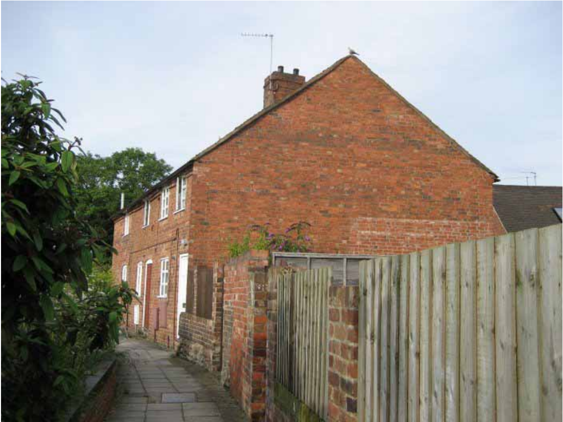
Plate 4. 31 & 32 Whitburn Street, on southern edge of and outside study area. Two small houses, C19th, formerly part of a court called Whitburn Place. View from southwest.
