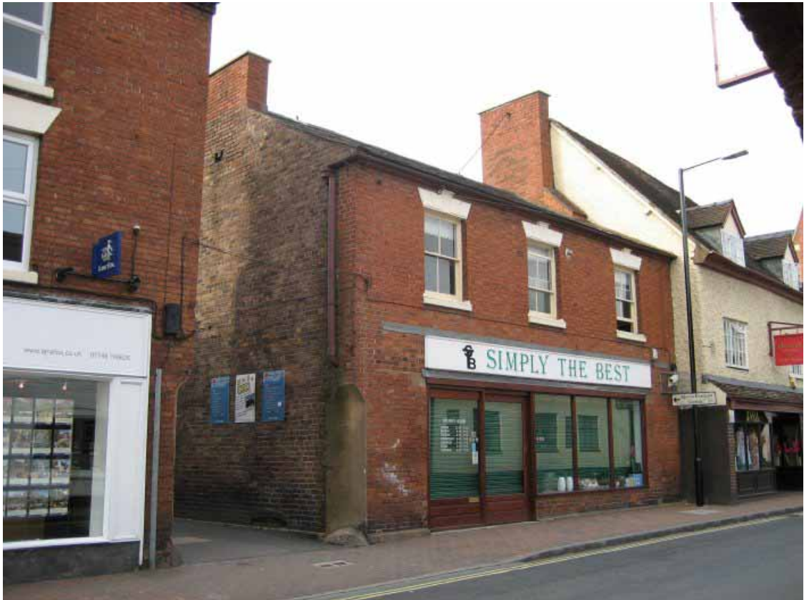
Plate 12. No. 8 Whitburn Street ('Simply The Best'), and adjacent passageway. A 19 th century three-bay, two-storey brick building, with cellar.
