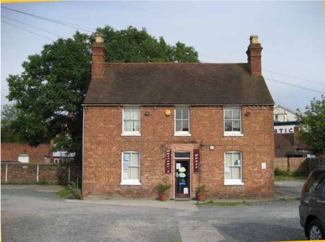
Plate 6. ‘Quilter’s Quest’, commercial premises on south side of the study area. This building is identified for demolition in the planning application. A three-bay, two-storey late 19 th century house, this building originally stood at the end of Whitburn Place. View from northwest.
