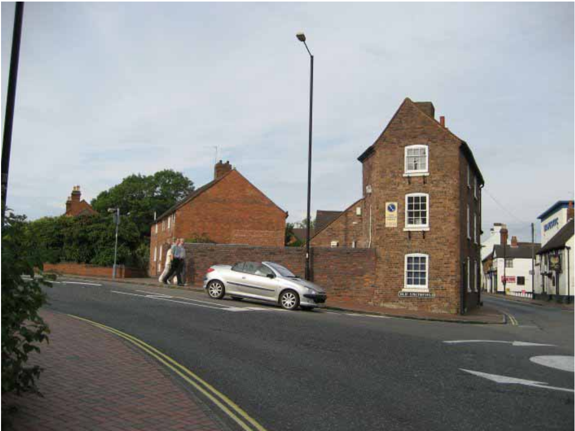
Plate 3. Junction of Whitburn Street (on right) and Old Smithfield (on left). View looking northeast. No. 34 Whitburn Street, on the corner is C19 th .
