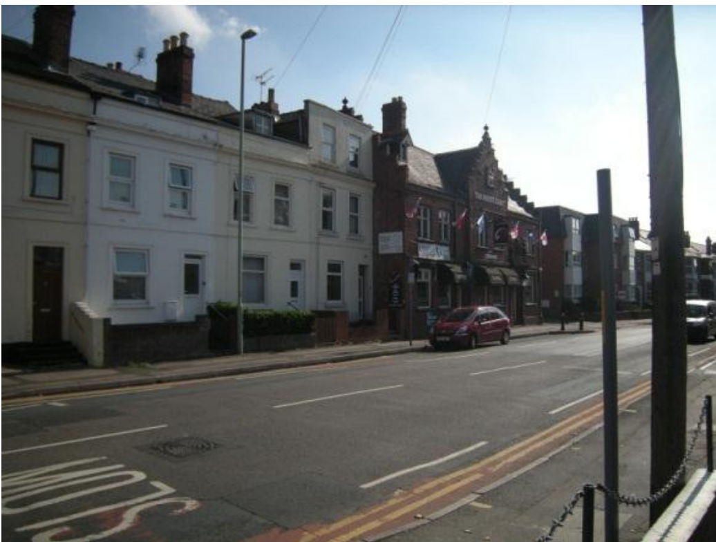
Plate 8 View south east from site along Kingsholm Road towards the White Hart public house
