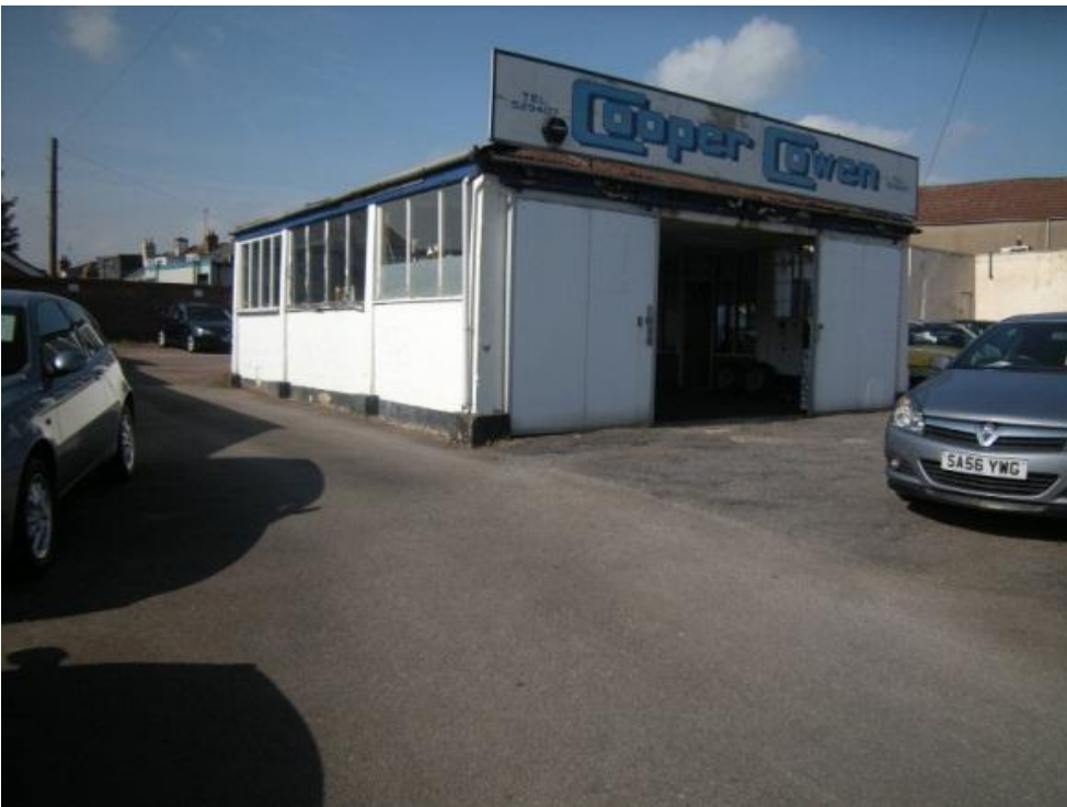
Plate 2 Looking north west toward car workshop bulding
