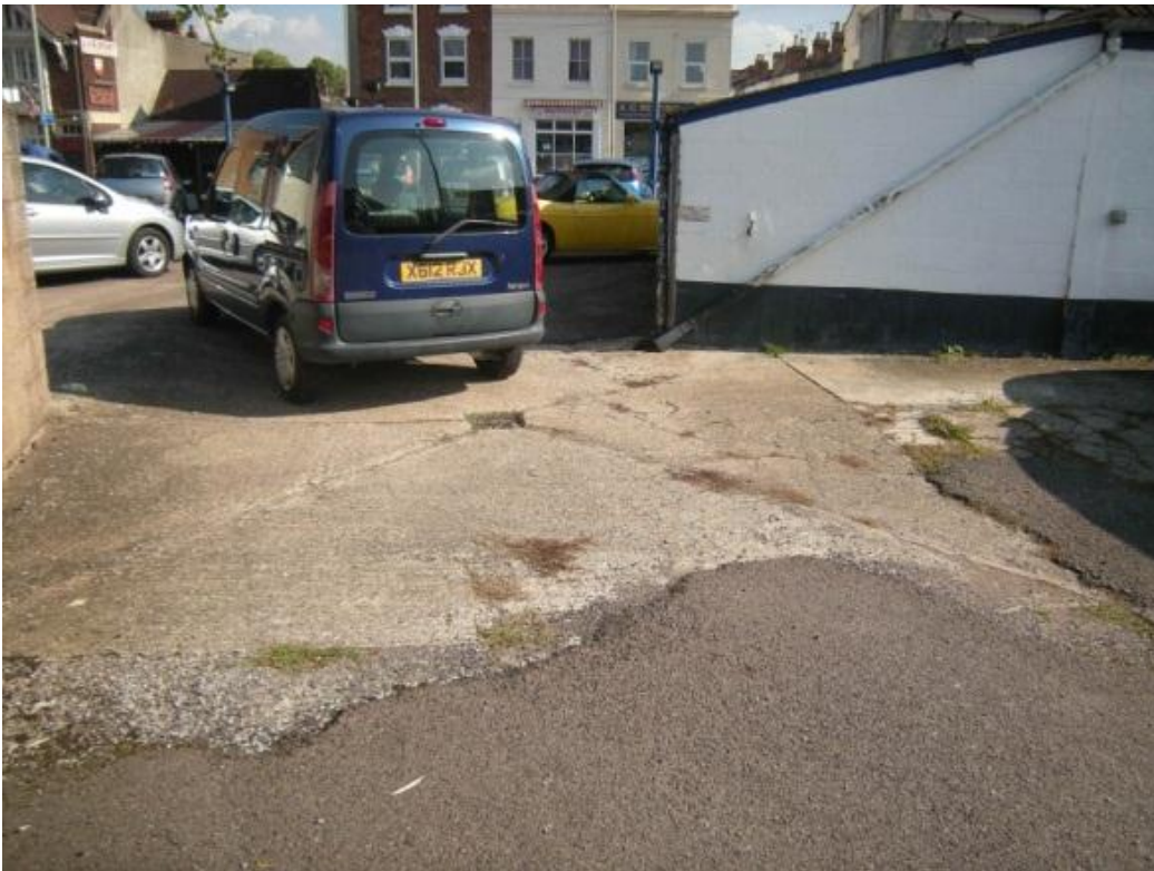
Plate 7 Detail of drainage to north-west of car workshop
