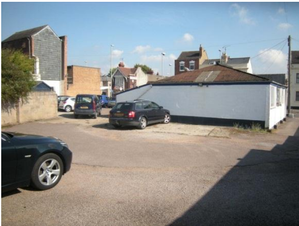
Plate 3 View east from rear of the site showing the car workshop and concrete floor to rear
