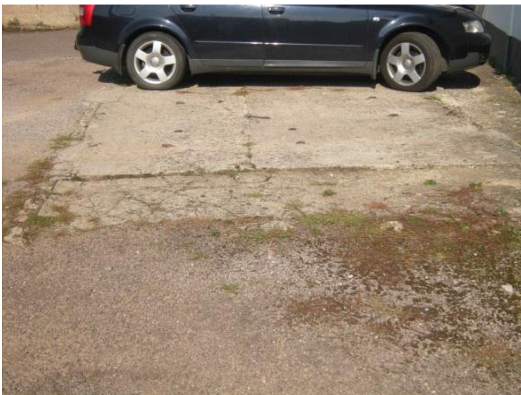
Plate 4 Detail of concrete floor from south
