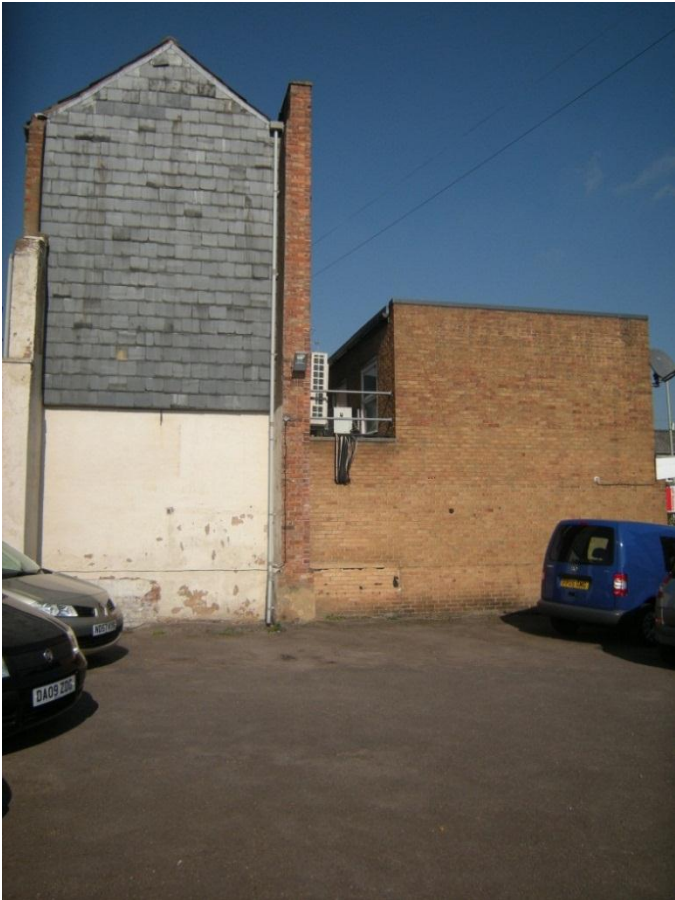
Plate 6 Three storey building and shop to north of site
