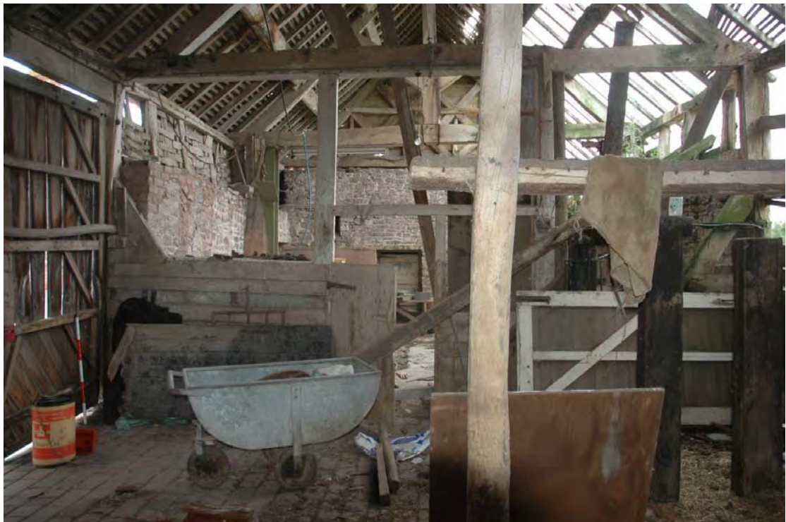
Plate 14: The Barn, Truss 2 with boarding and door of division across barn.
