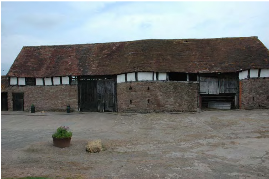
Plate 4: The Barn, south elevation
