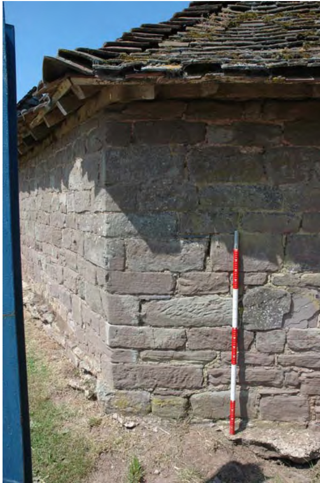
Plate 18: The Animal Shed, south western corner showing construction.
