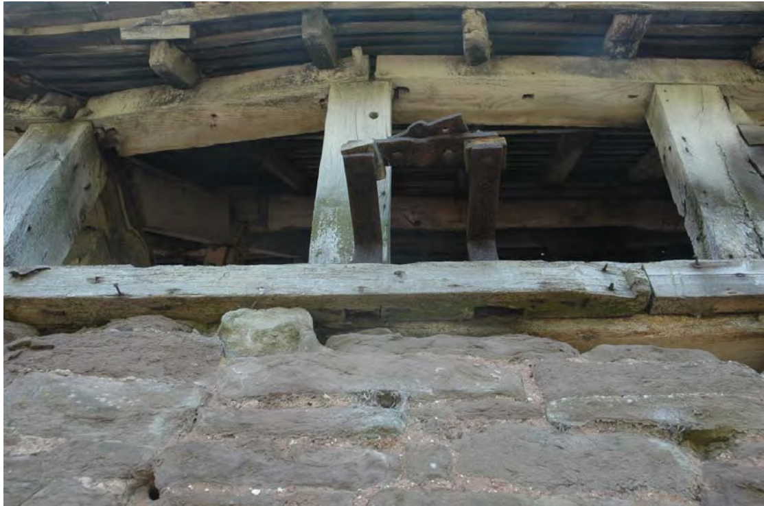
Plate 36: The Barn, north elevation, mid-section showing metal fixture which may relate to horse-powered threshing machine.
