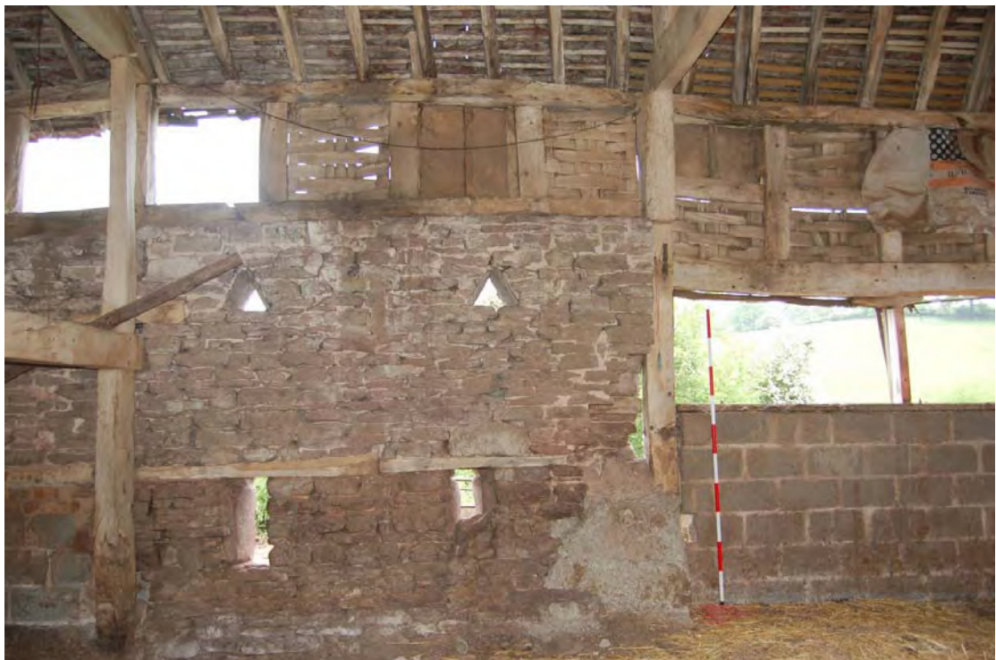
Plate 8: The Barn, north wall interior showing two types of ventilation holes.
