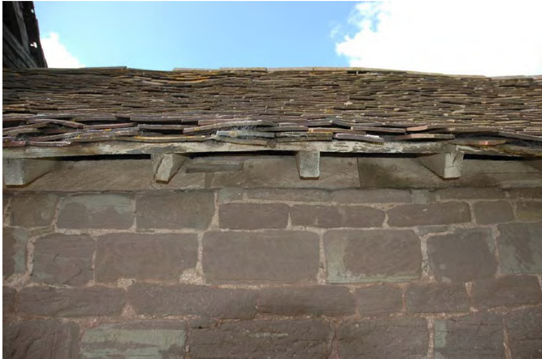
Plate 38: The Animal Shed, south wall exterior showing empty mortice suggesting re-used timbers were included in its construction.
