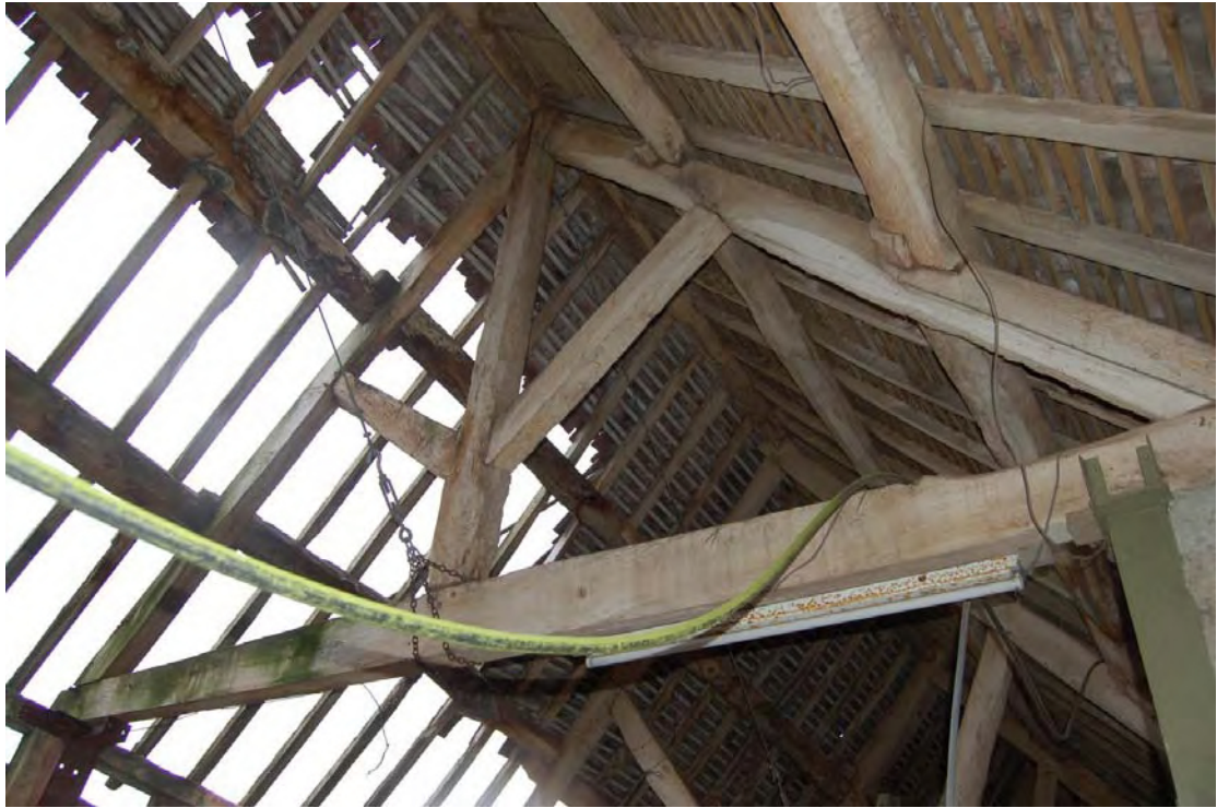
Plate 16: The Barn, Truss 1, King Post.
