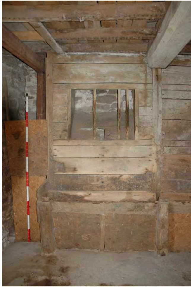
Plate 26: The Stable, west room, ground floor, showing chamfered beam to right of photograph.
