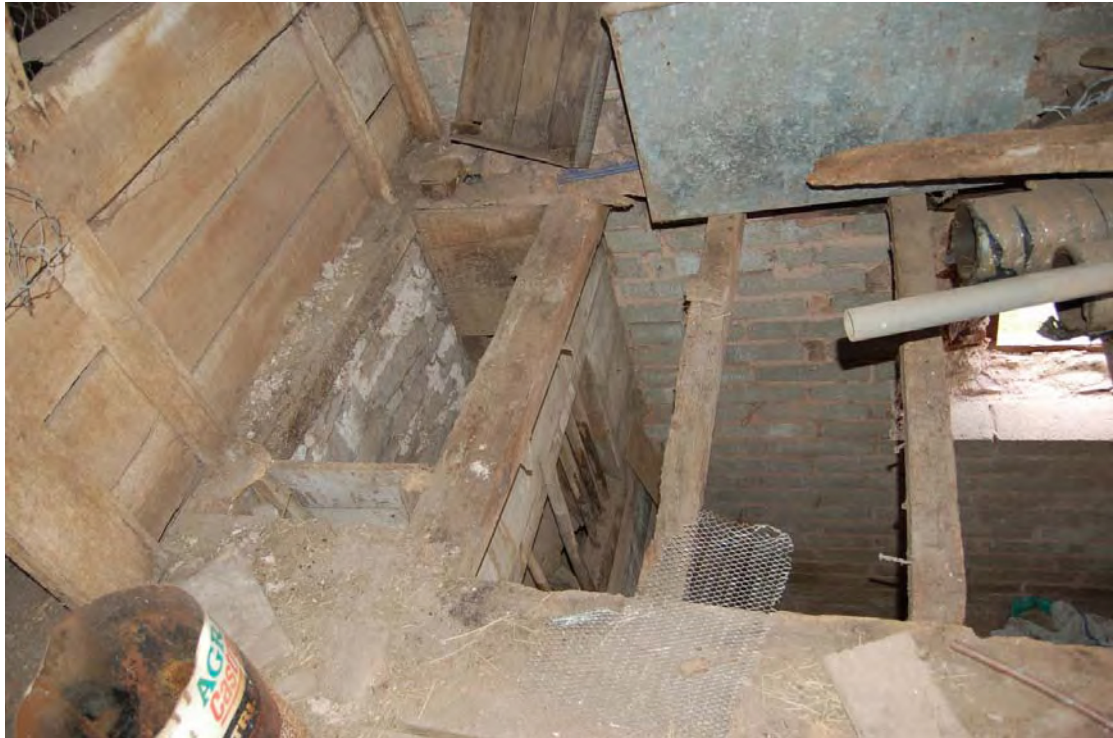
Plate 30: The Stable, west room upper floor showing shute to manger in lower room
