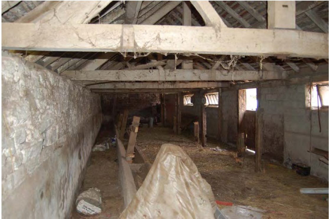
Plate 20: The Animal Shed, Room C, looking south east showing remains of the posts of stalls and a trough running down the building.
