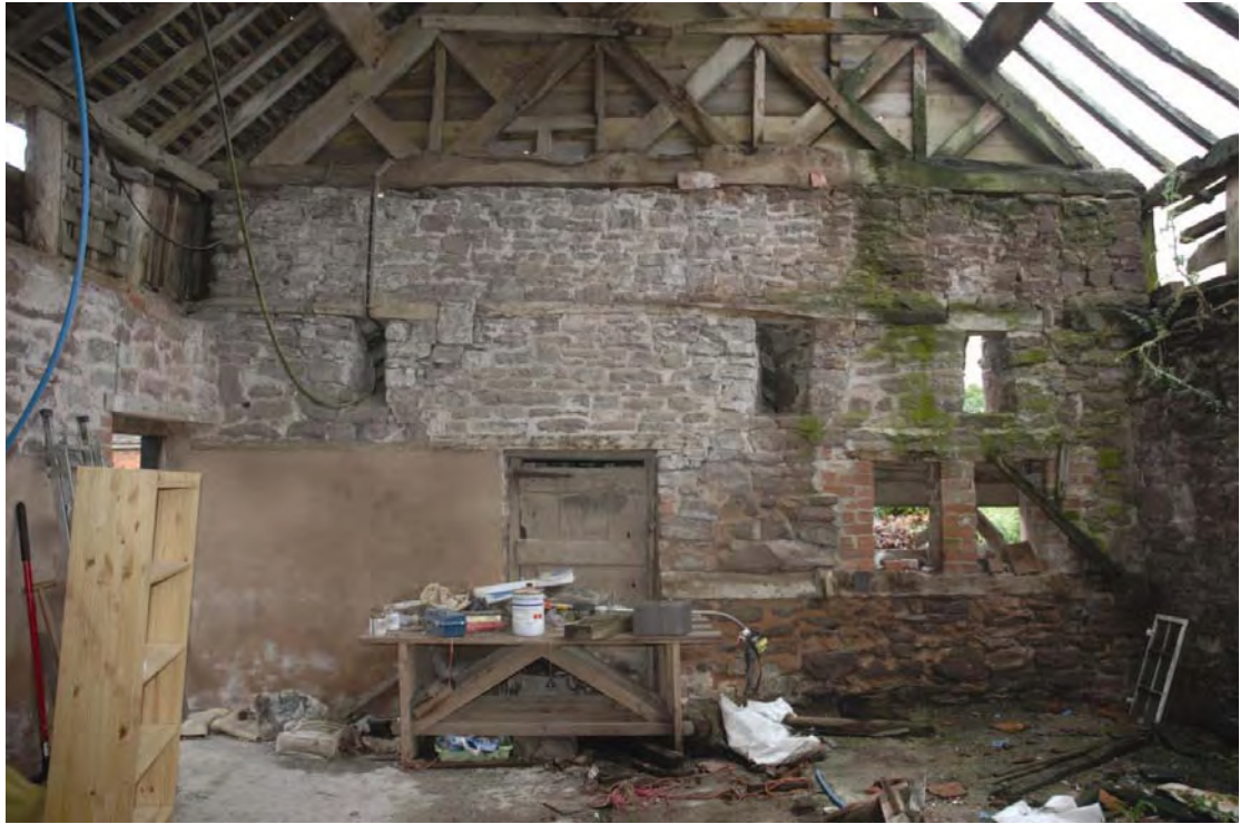
Plate 13: The Barn, eastern wall with small central door
