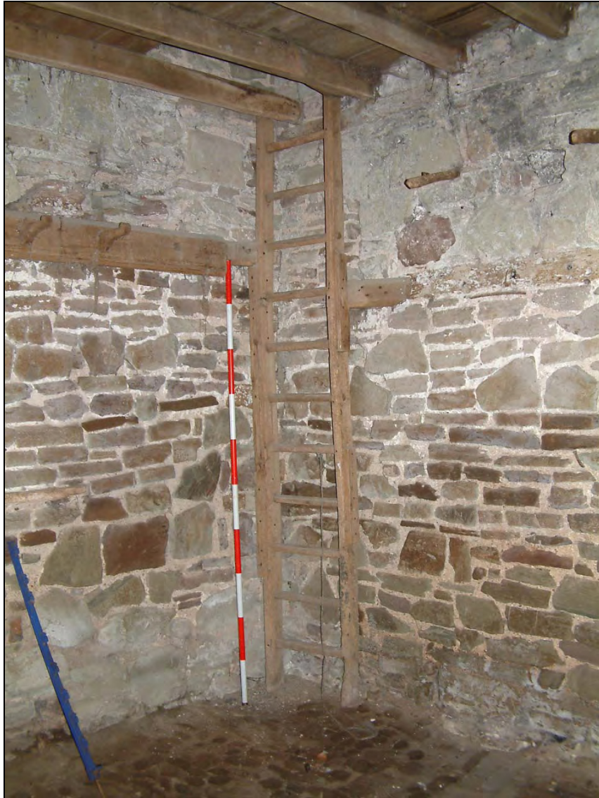
Plate 17: Building 3 ladder access to hayloft
