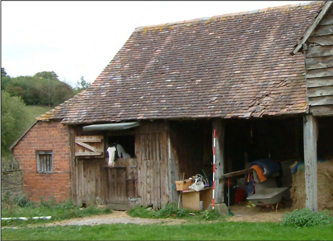
Plate 27: Building 2 loose box
