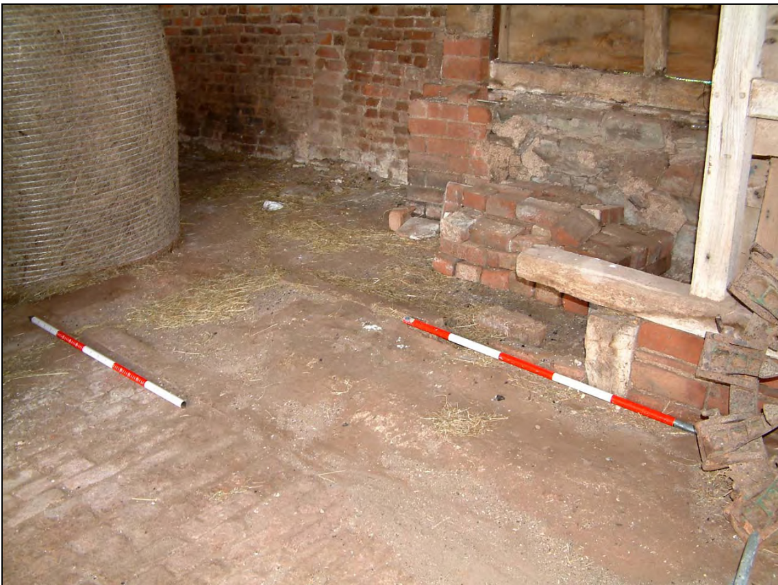
Plate 8: Interior of building 2 showing former position of feeding trough
