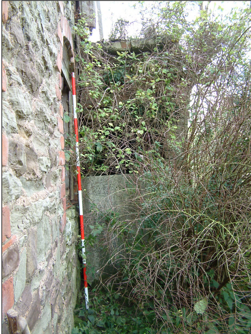
Plate 19: Building 3 kennel under granary stairs
