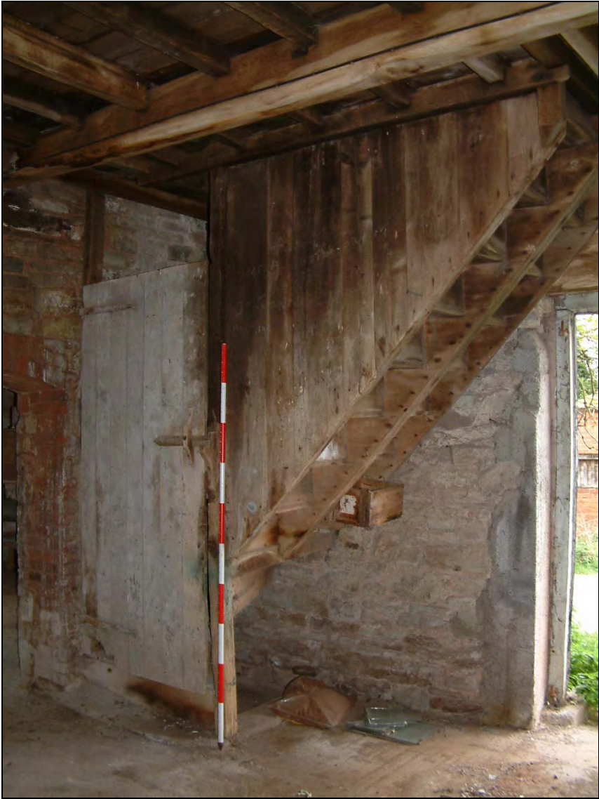
Plate 4: Staircase in building 1
