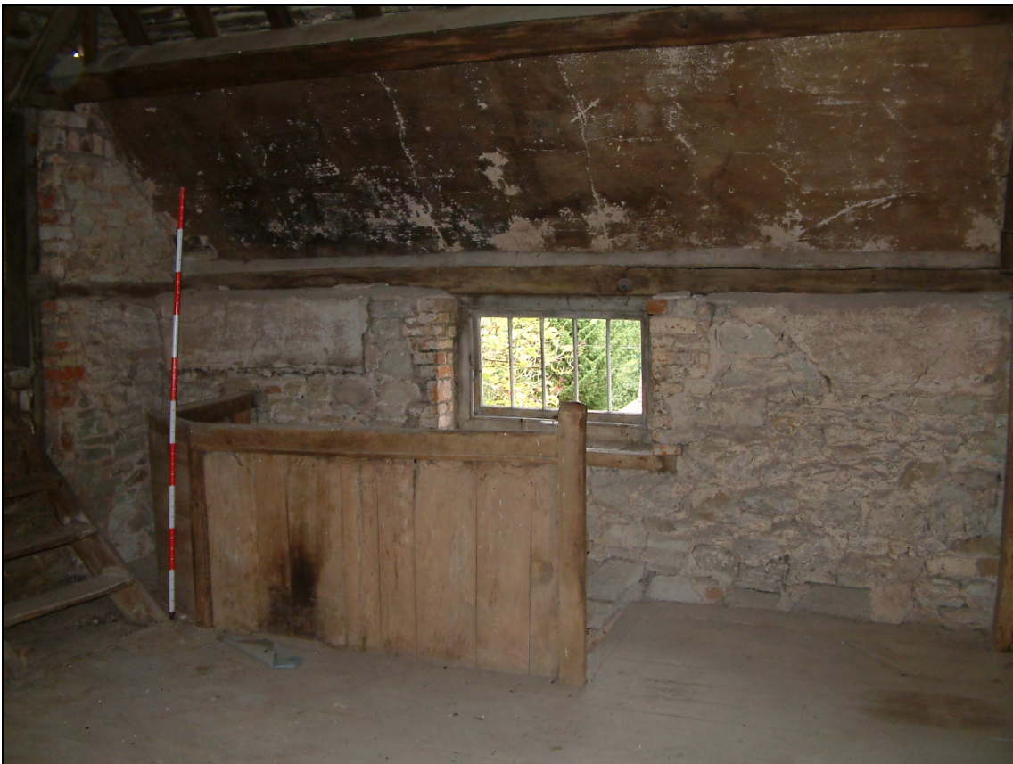
Plate 2: Internal elevation of building 1 showing painted plaster at north east end
