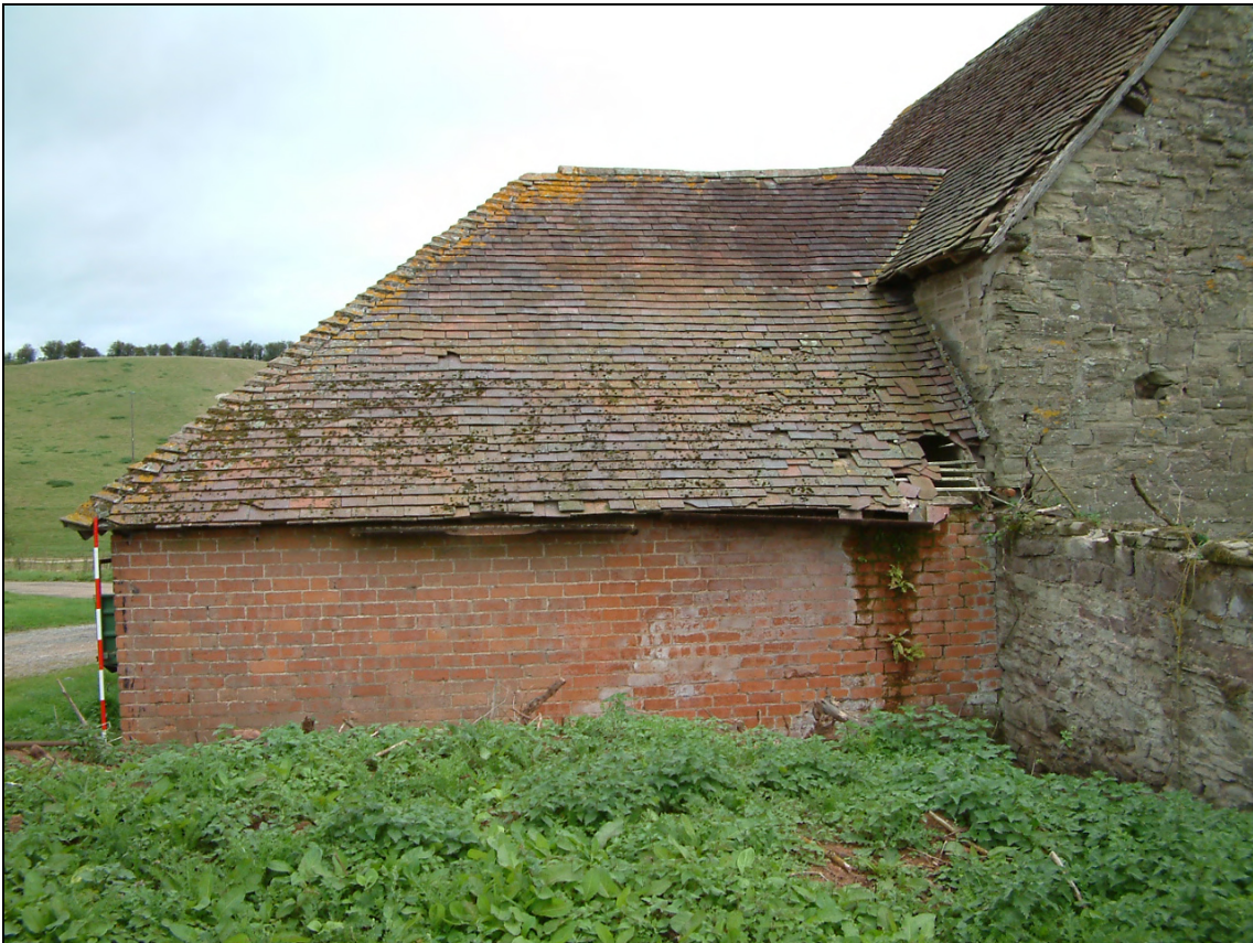
Plate 22: Building 1 cart shed wall
