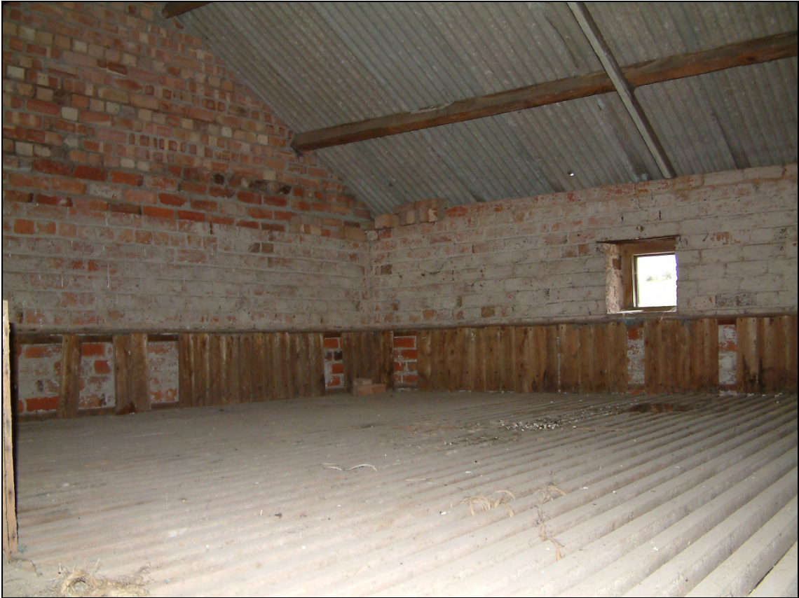
Plate 25: Building 1 hop kiln drying floor
