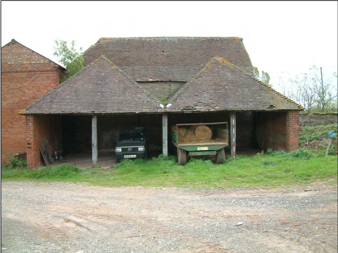
Plate 23: Building 1 cart shed open front
