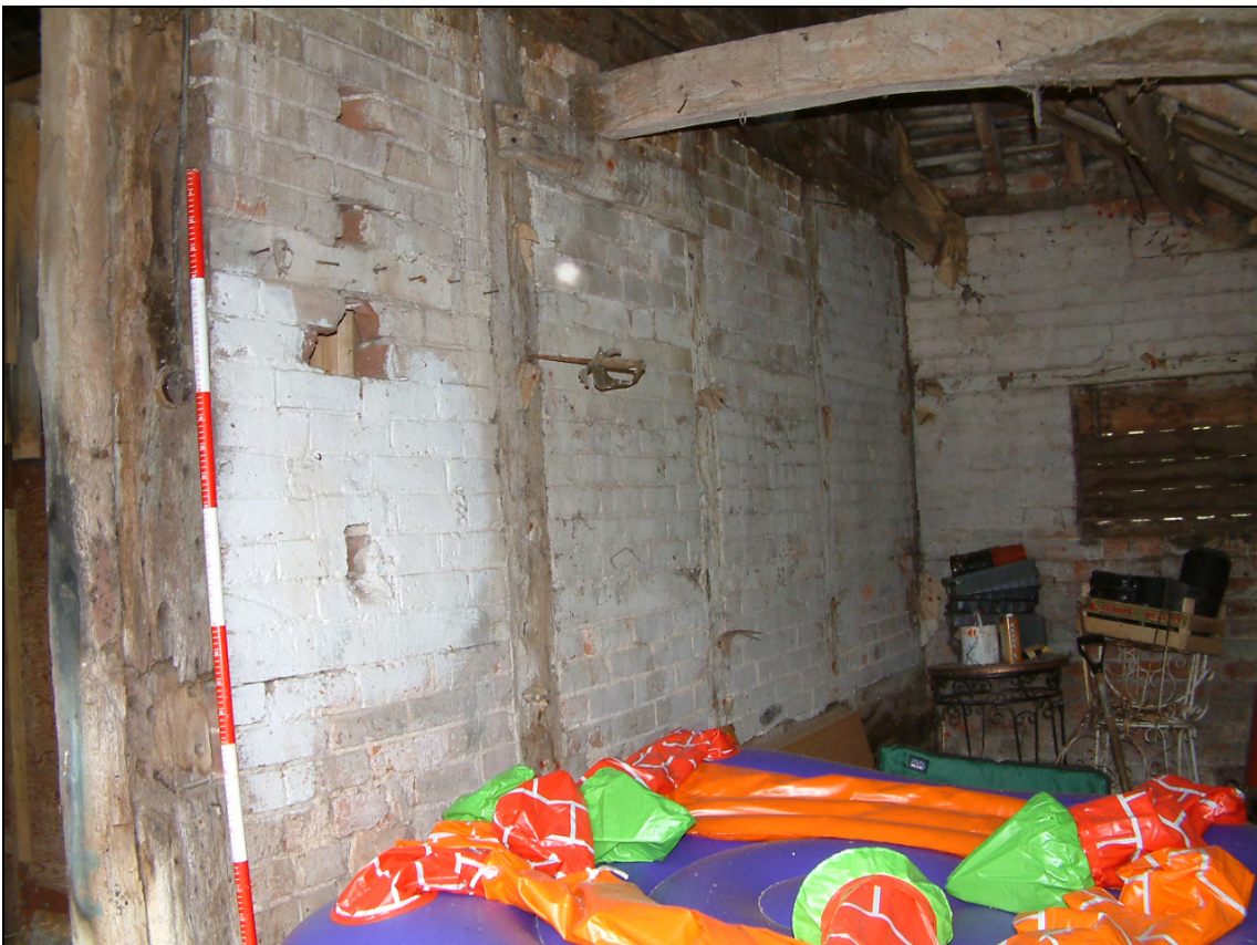
Plate 6: Timber wall of the original phase of building 2
