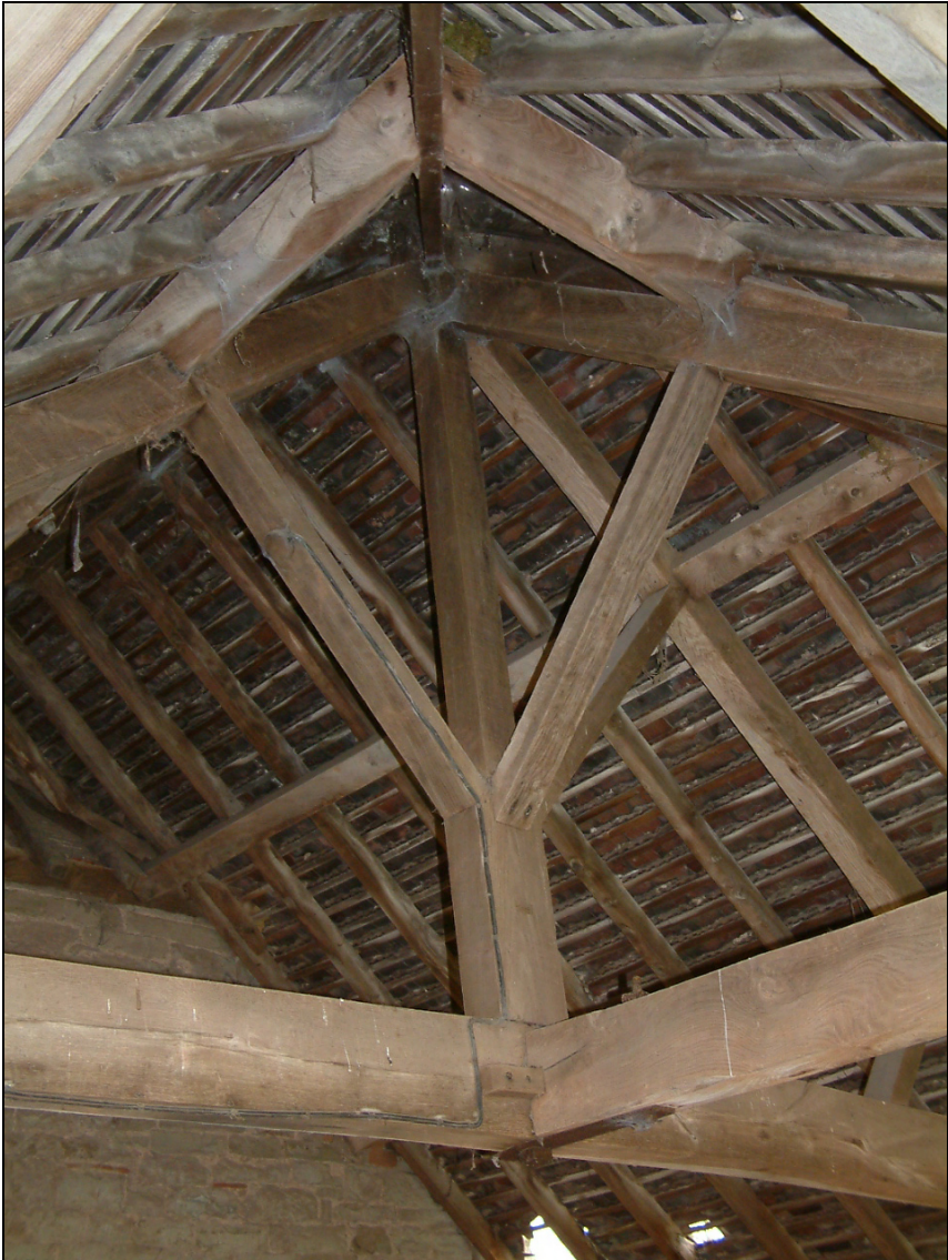
Plate 24: Building 1 cart shed crown post truss
