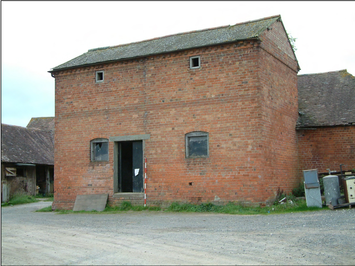
Plate 10: Hopkilns of building 1 from the north
