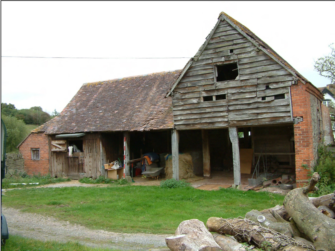
Plate 7: West elevation of building 2 showing timber posts of shelter shed
