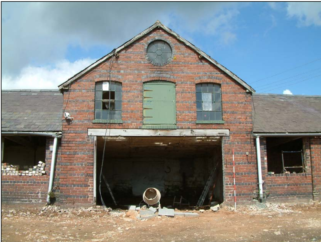
Plate xiv: South-east facing elevation, Unit 8
