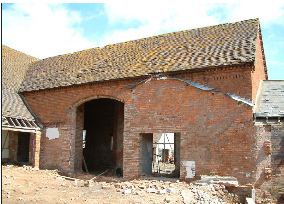
Plate xii: South-west facing elevation, Unit 7
