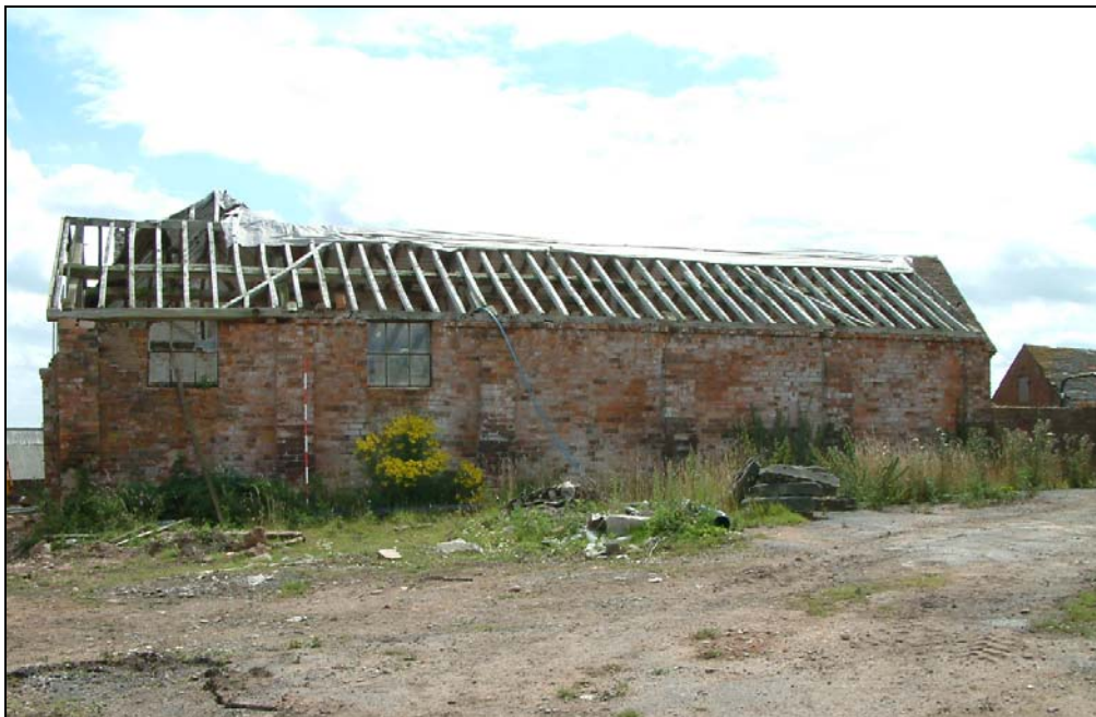
Plate vi: North west facing elevation of Unit 4
