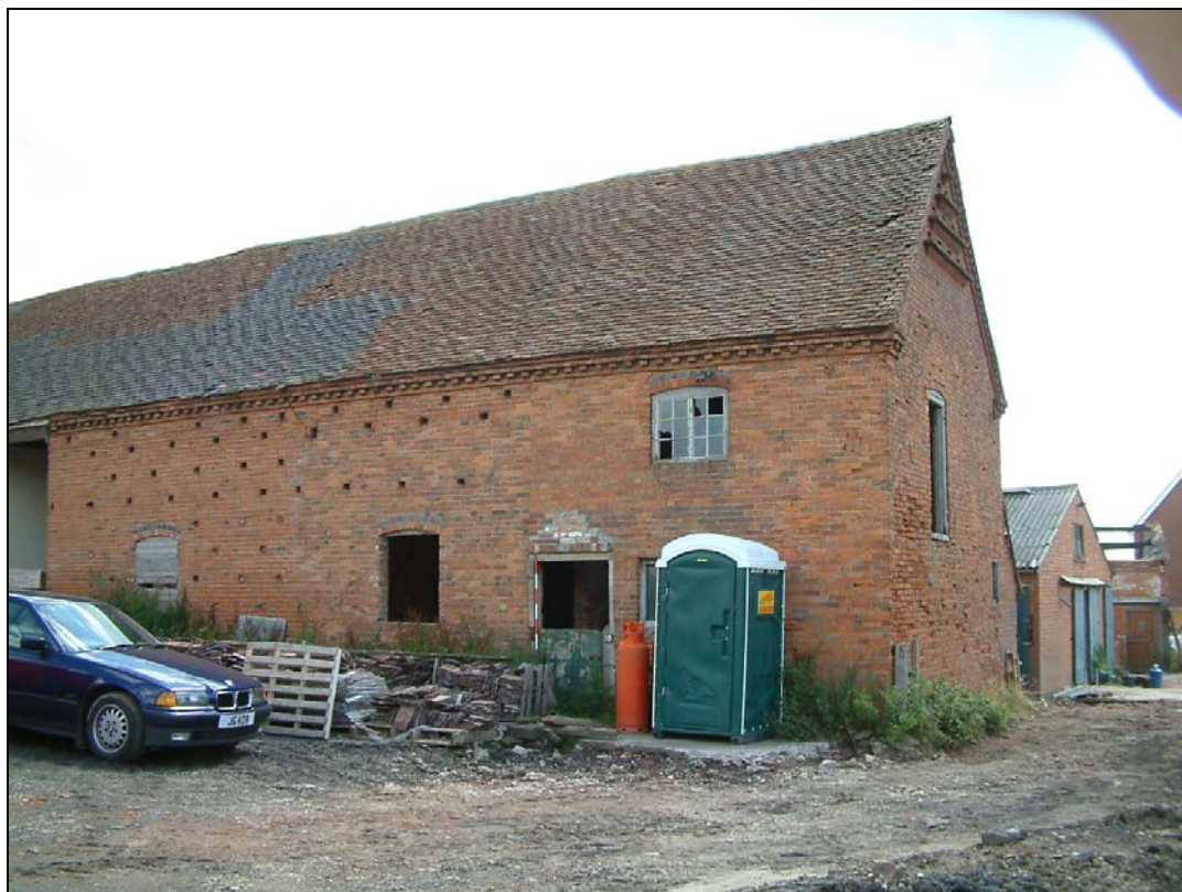
Plate iii: North-west facing elevation of Unit 2
