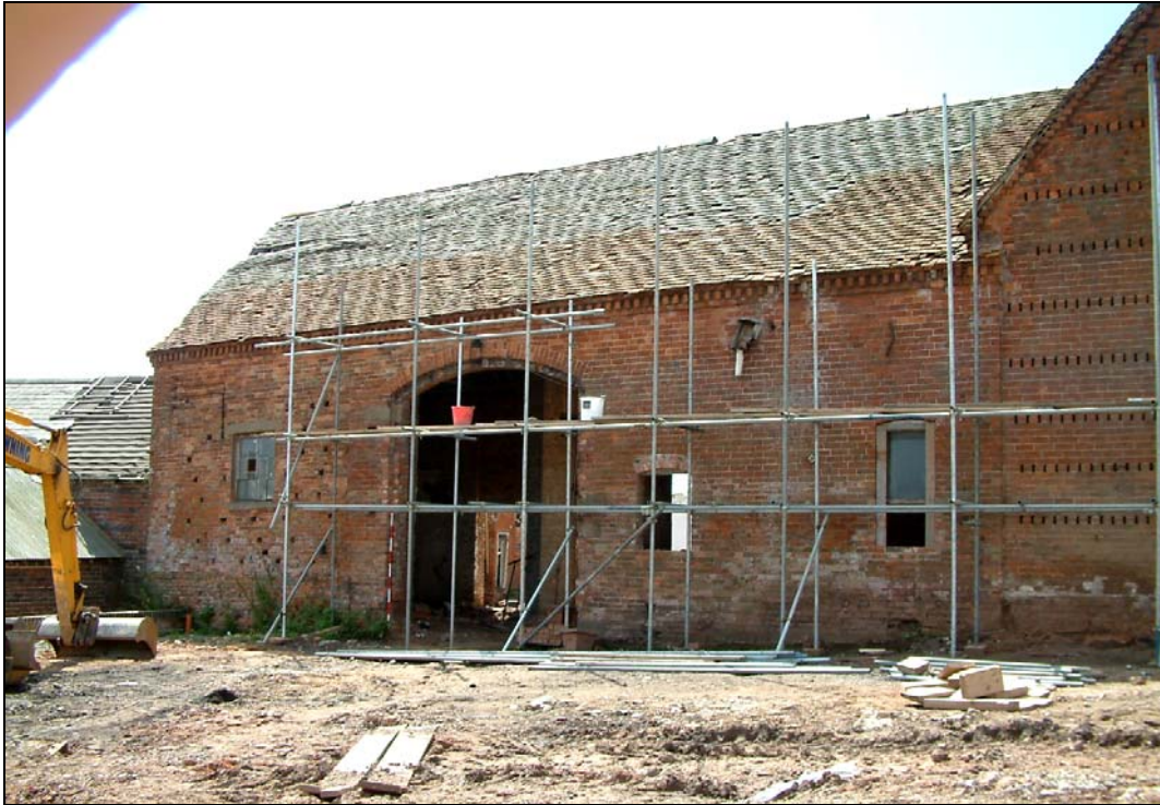
Plate xiii: North-east facing elevation, Unit 7
