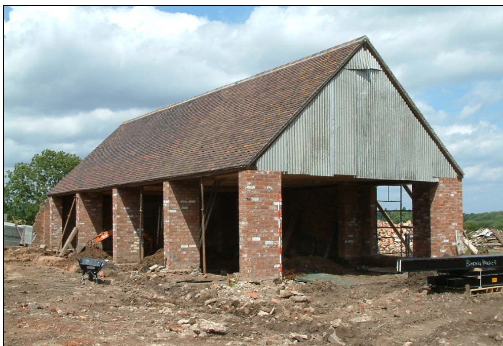
Plate viii: Gable and south-west elevation of Unit 5
