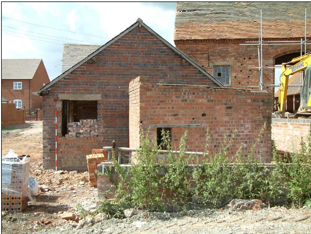
Plate xv: North-east facing gable, Unit 8
