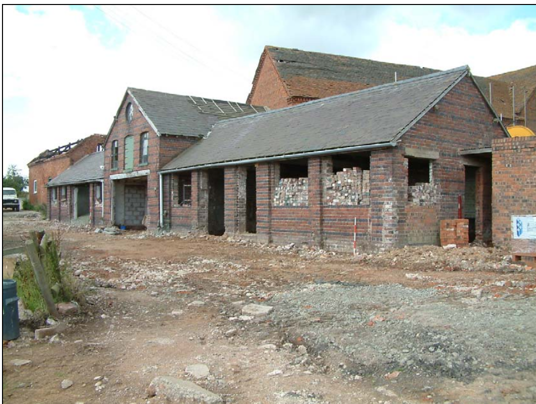
Plate xvi: South-east facing elevation, Unit 8, 10 and 9
