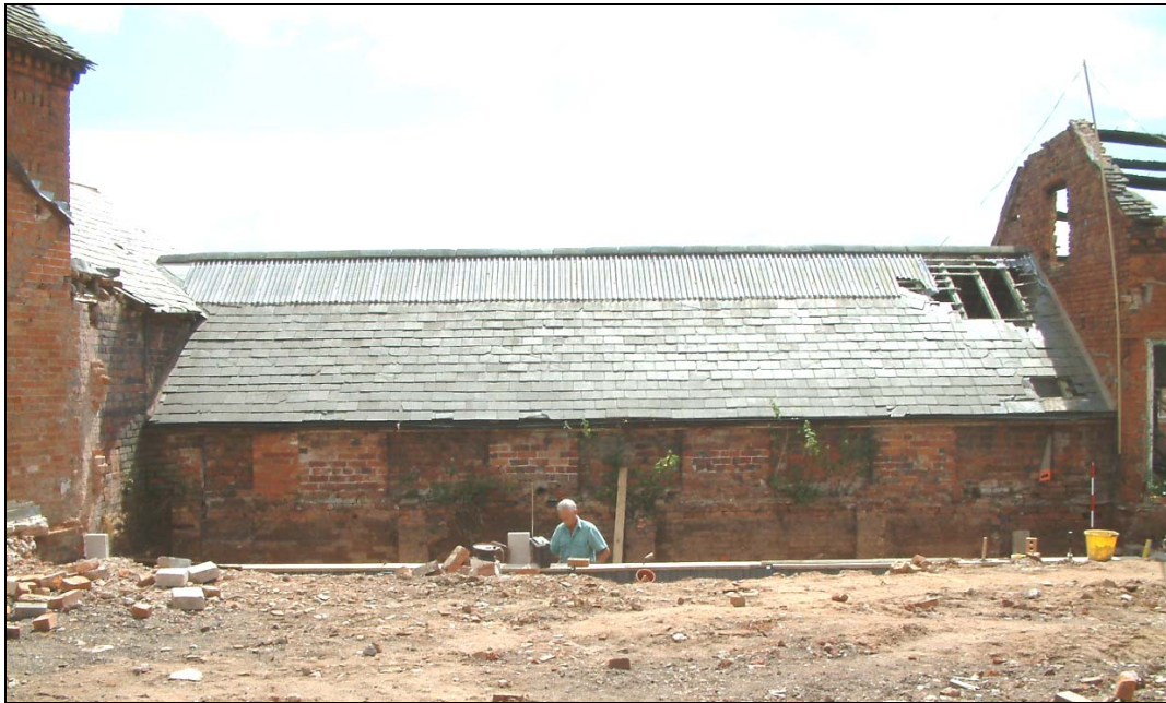
Plate xxi: North-west facing elevation, Unit 10
