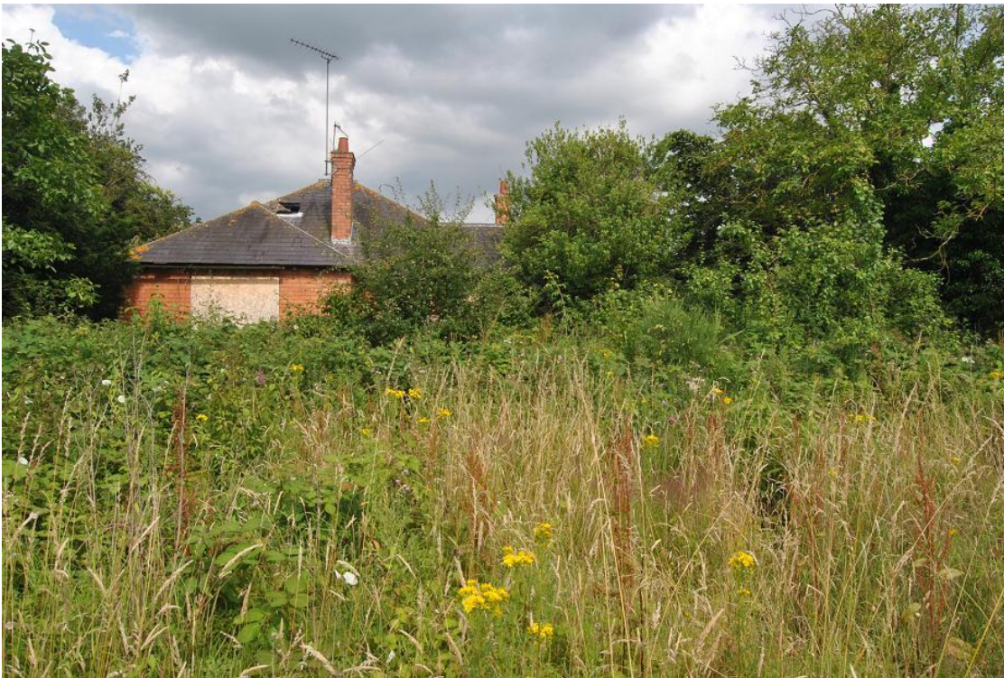
Plate 2 Derelict house standing within the proposed development area; looking east
