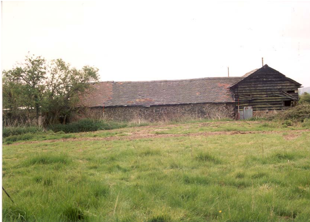
Plate 1: Animal shelter shed (building 1) and hay storage barn (building 2), northeast elevation.
