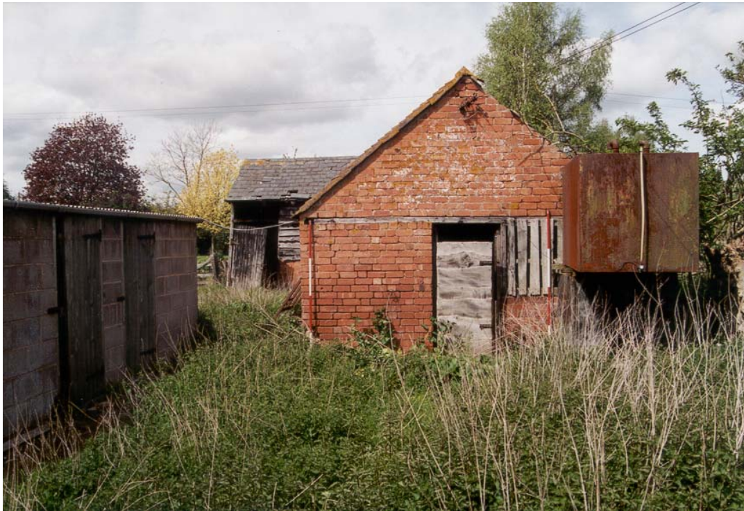
Plate 3: Workshop (building 3), southeast elevation.
