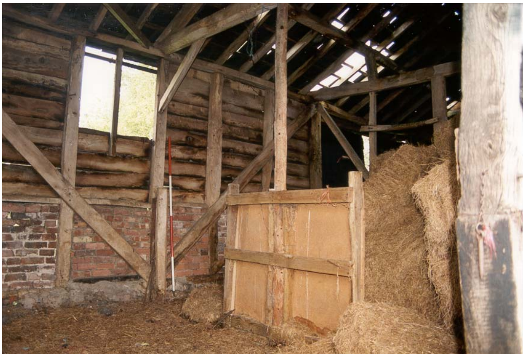
Plate 8: Hay storage barn (building 1), internal detail.
