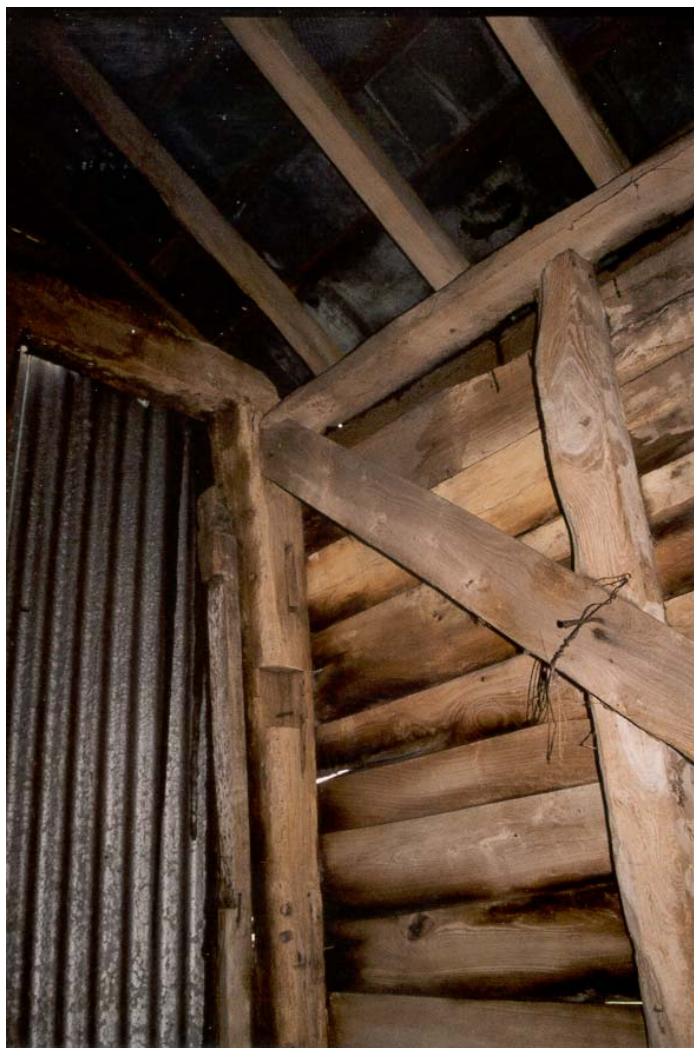
Plate 9: Hay storage barn (building 1), internal detail.
