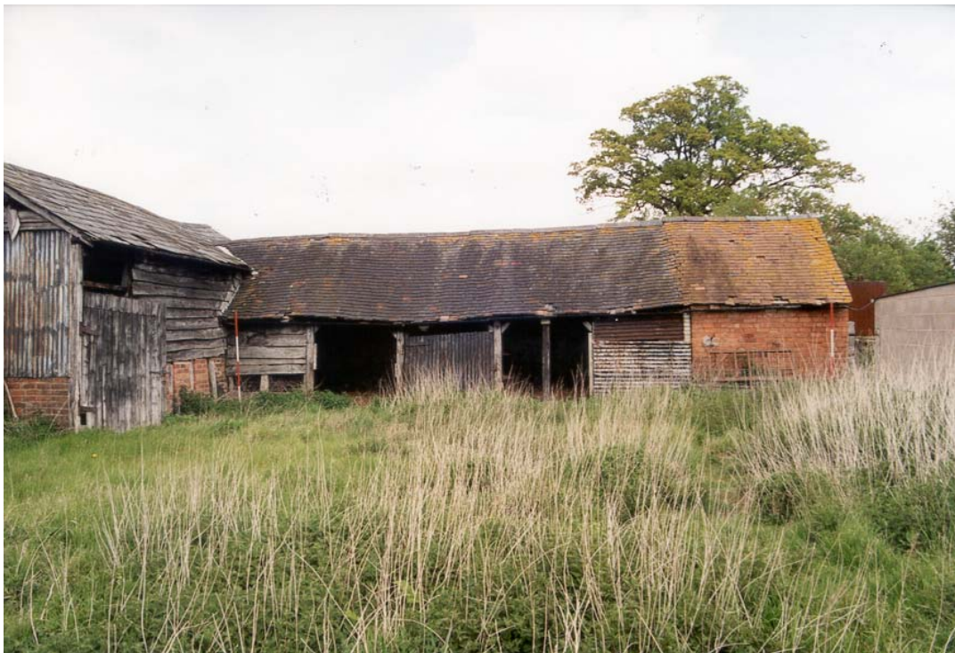
Plate 4: Animal shelter shed (building 2) and workshop (building 3), southwest elevation.
