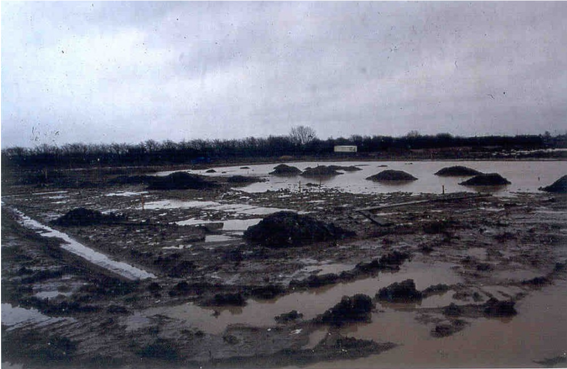
Plate 3: Area 3, flooded during excavation, view south-east
