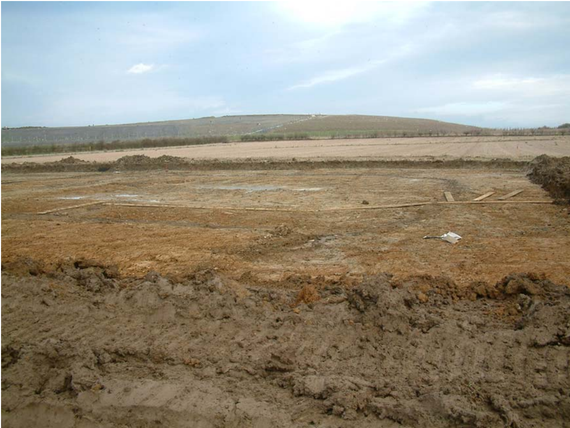
Plate 2: Area 3, as stripped, view north
