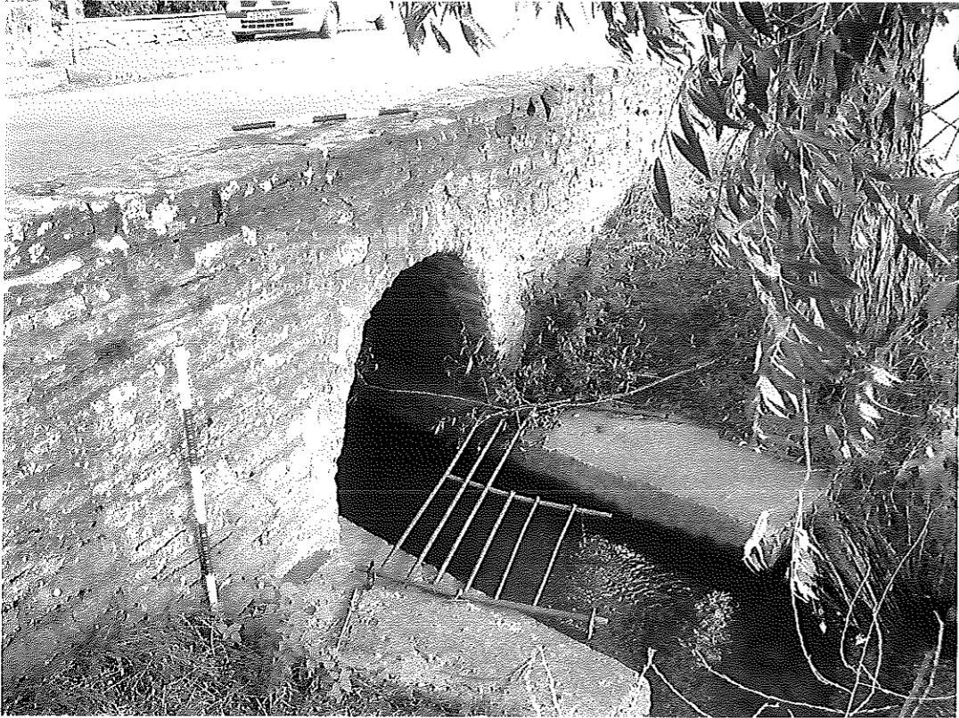
Plate 10 South bridge, looking NE at south side of bridge
