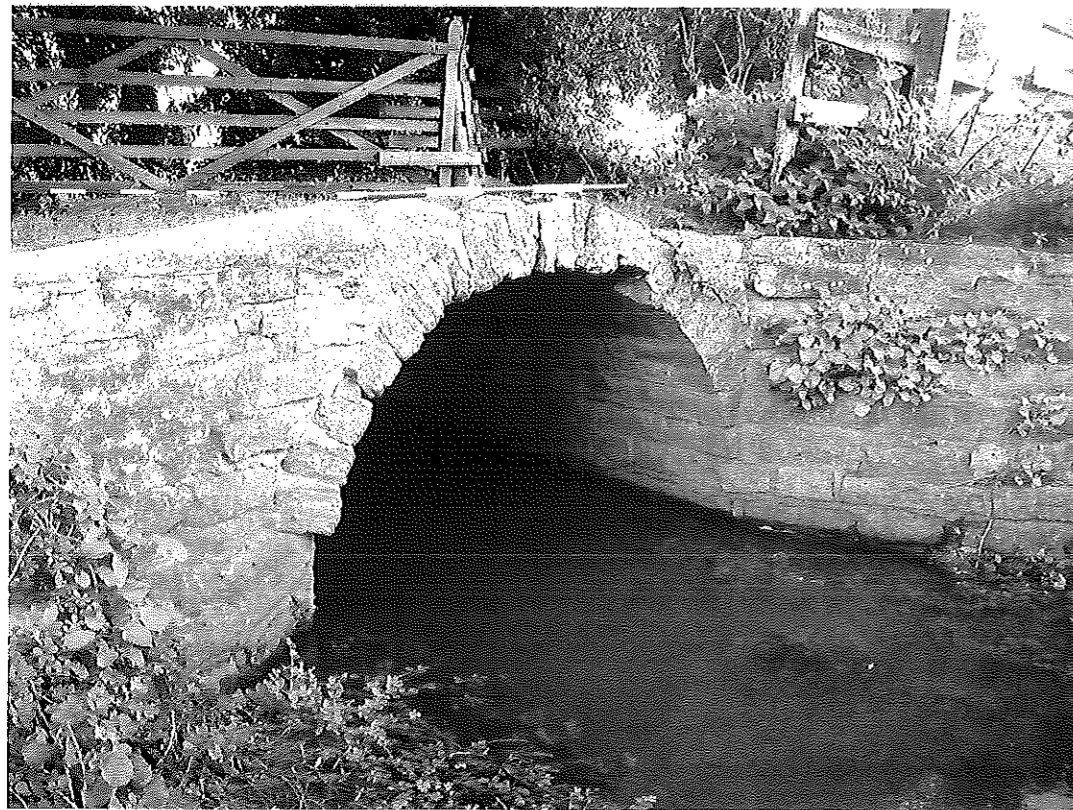
Plate 14 Field bridge, south side of bridge
