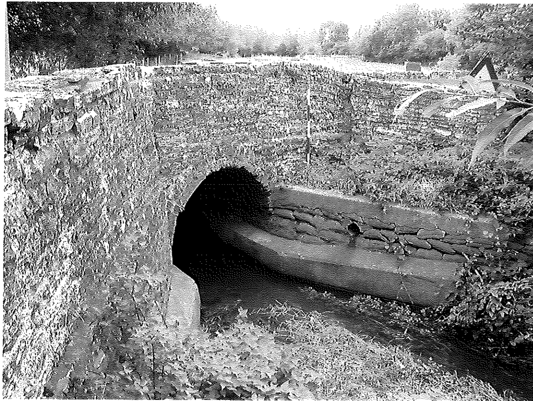
Plate 11 South bridge, culverted north entrance to bridge
