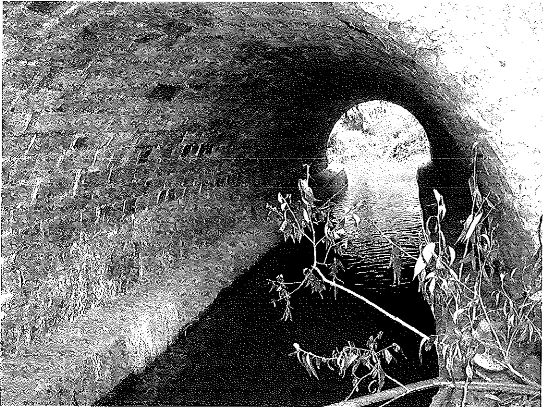
Plate 9 South bridge, view north along tunnel
