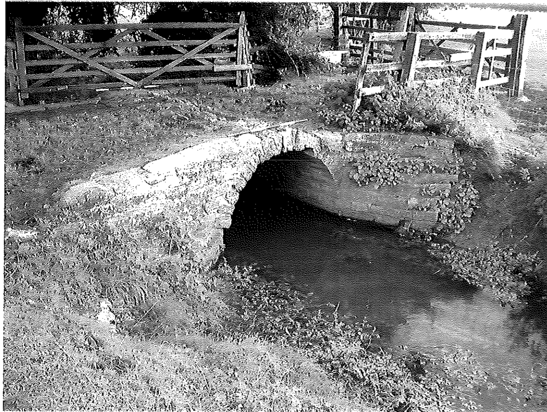
Plate 13 Field bridge, south side of bridge
