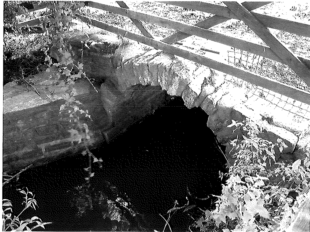
Plate 15 Field bridge, close up of arch
