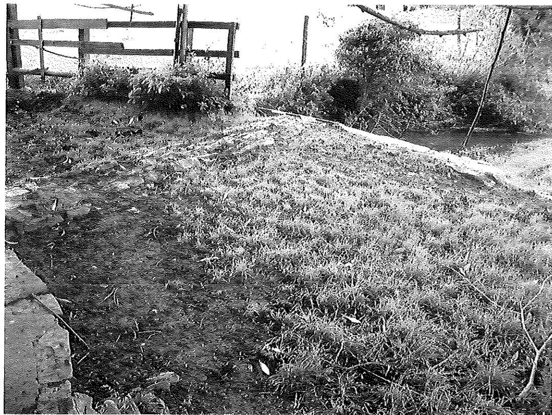
Plate 16 Field bridge, looking SE, top of bridge arch visible on path
