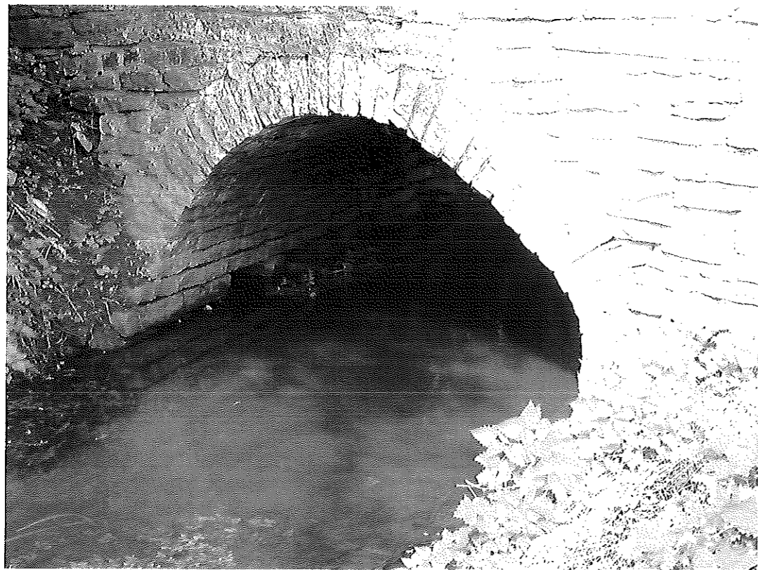
Plate 6 Footbridge, detail of south face
