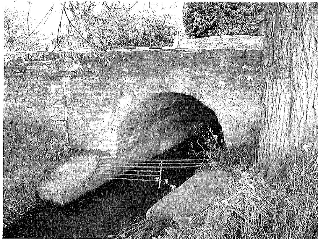
Plate 8 South bridge, south face
