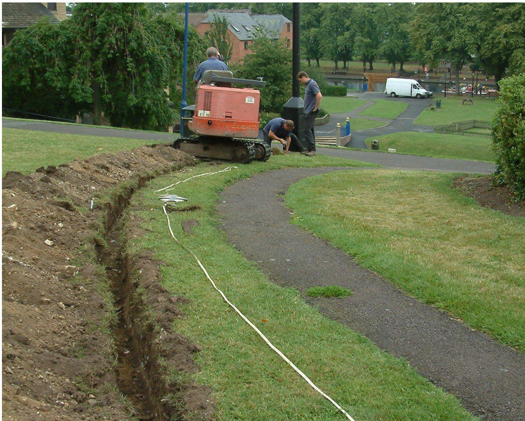
Plate 4: General view of groundworks at northern end, facing east
