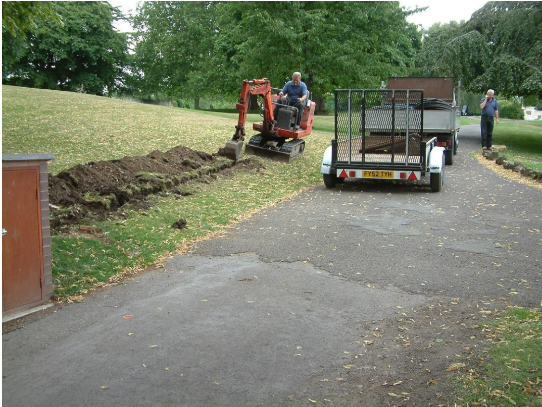
Plate 1: General view of groundworks at southern end, facing north
