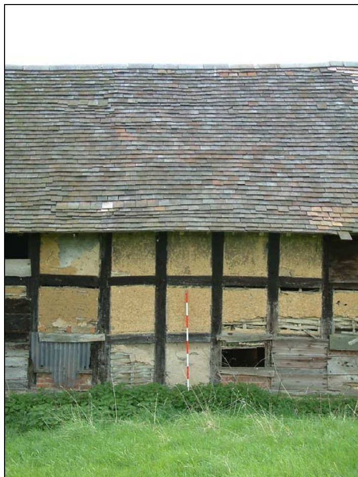
Plate 2: Construction fabric of north wall of barn 1
