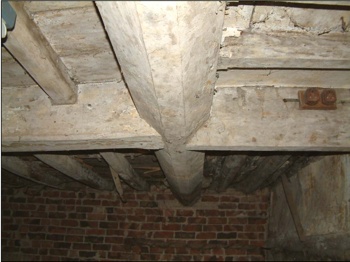
Plate13: Interior of barn 1 wing, shaped ceiling beams and joists
