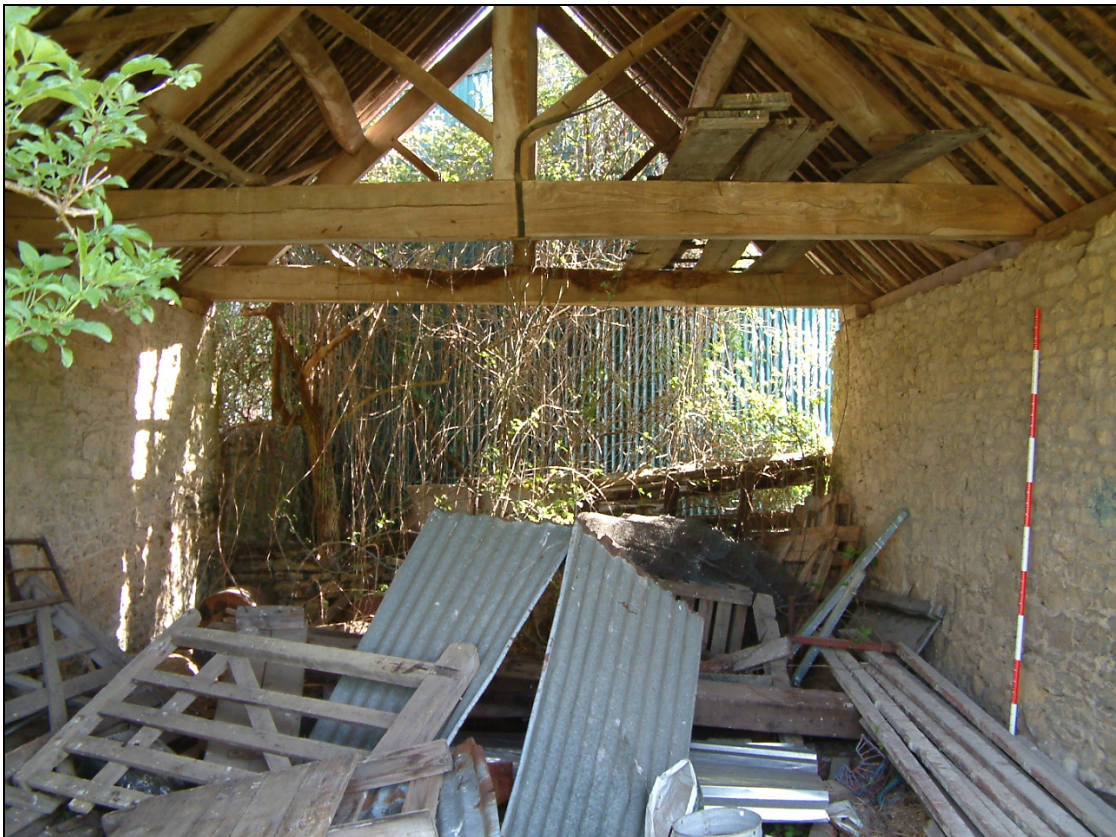
Plate 10: Barn 3 interior showing large king post trusses
