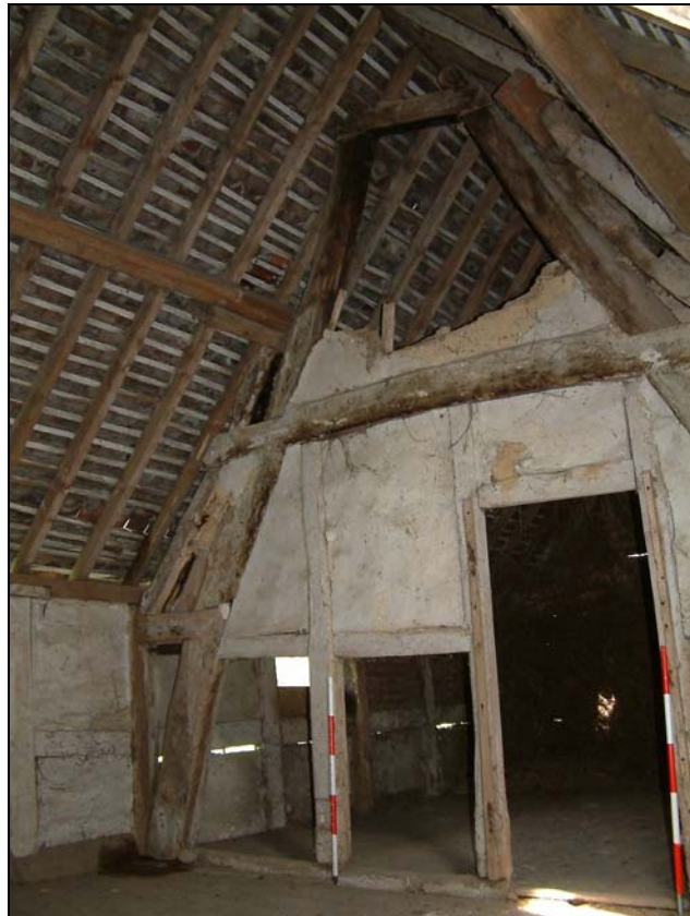
Plate 11: Interior of barn 3 showing cruck truss
