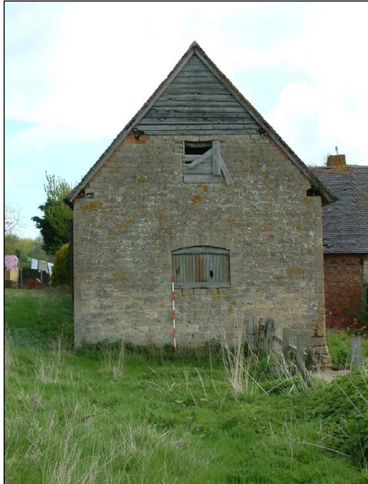
Plate 24: Barn 1 west gable, with pitching opening
