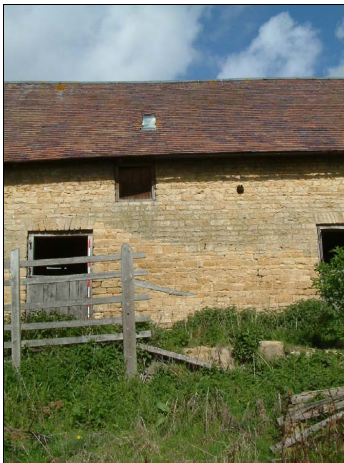
Plate 3: Construction fabric of south wall of barn 1
