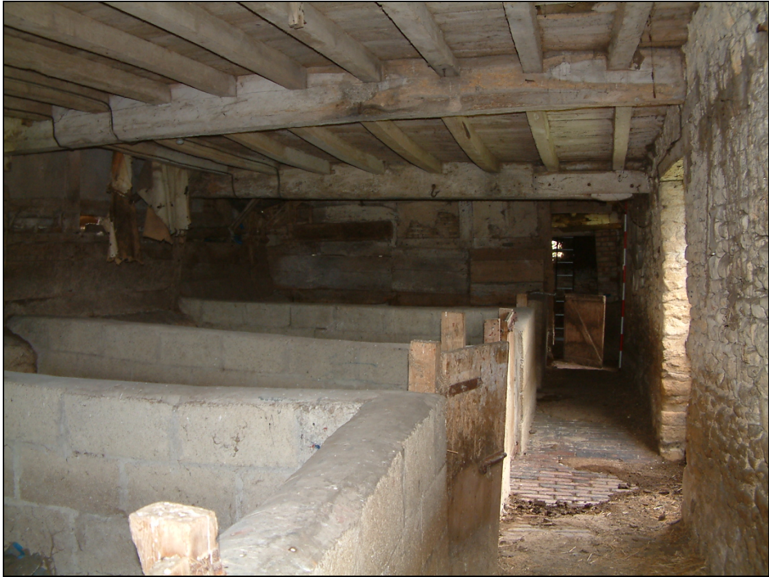
Plate 5: Interior of barn 1 showing breezeblock stable divisions
