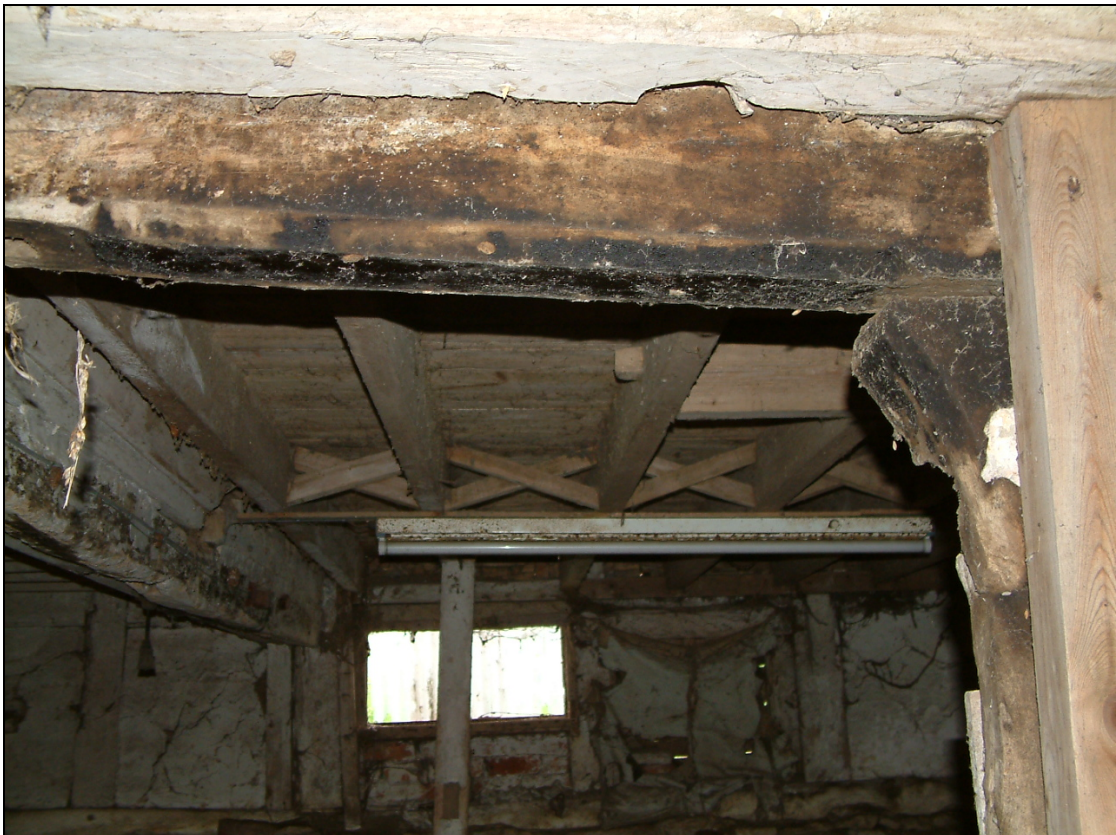
Plate 14: Barn 1 shaped bressumer and door opening
