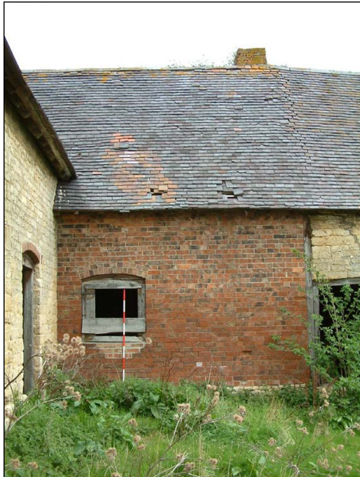
Plate 22: West elevation of barn wing, rebuilt in brick
