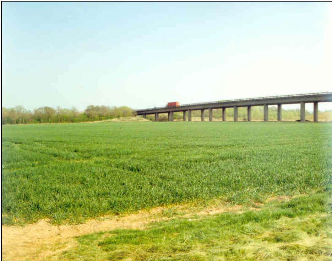
Plate 1: M50 road bridge spanning northern extent of field 3 and 4
