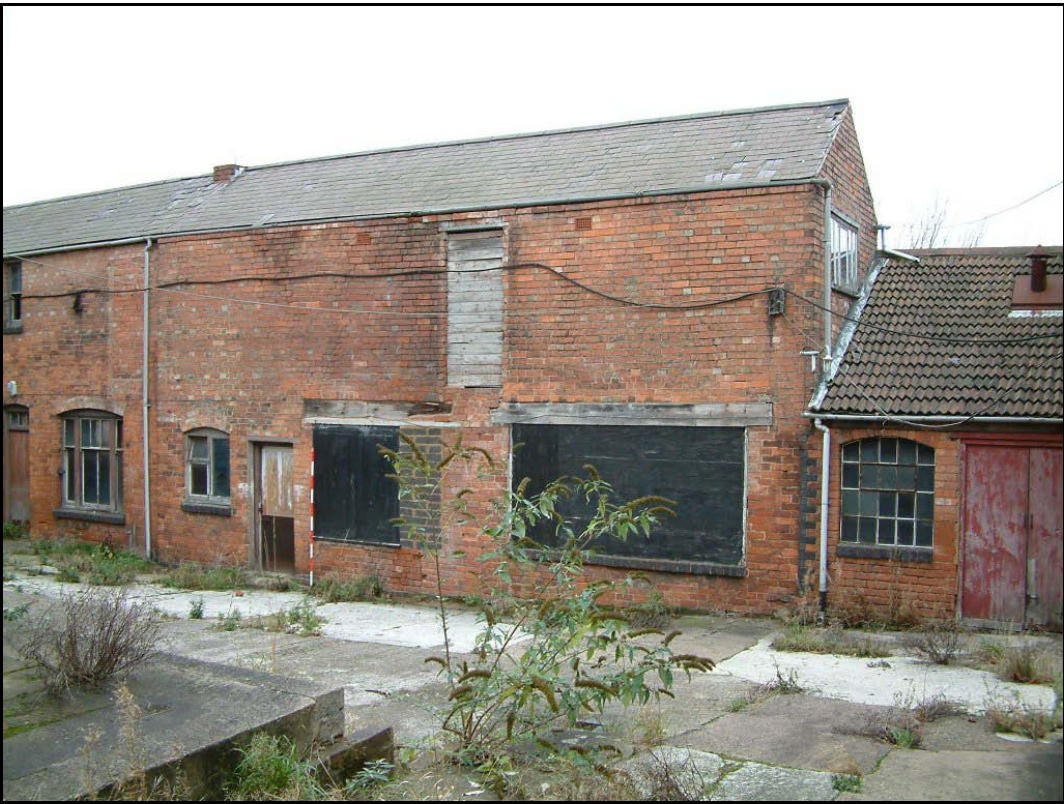
Plate 22: Range 3 building C, from the east
