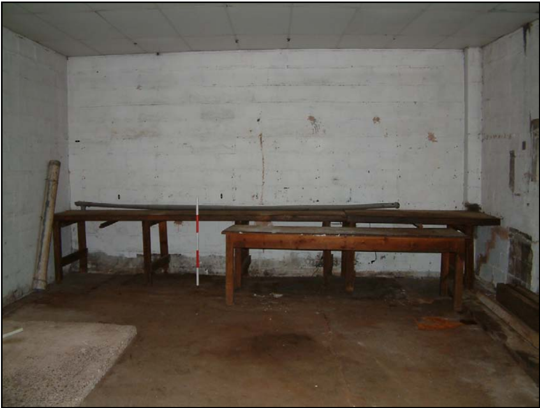
Plate 29: Range 4 building B interior
