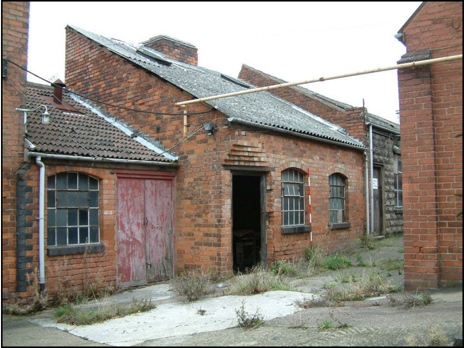
Plate 26: Range 4 building A, from the south
