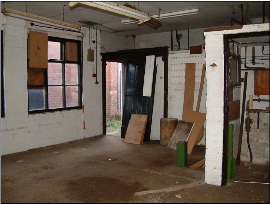
Plate 30: Range 4 building B interior
