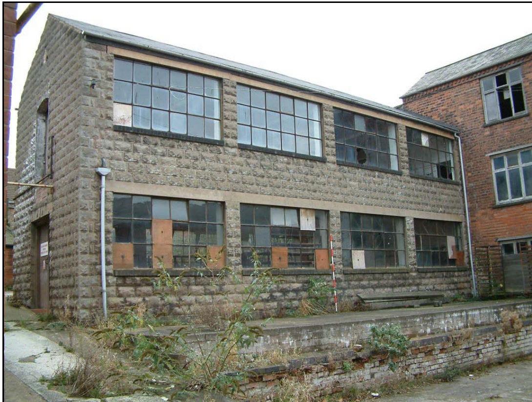
Plate 13: Range 2 from the north-west
