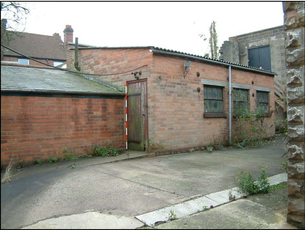
Plate 36: Range 7 building A, from the west
