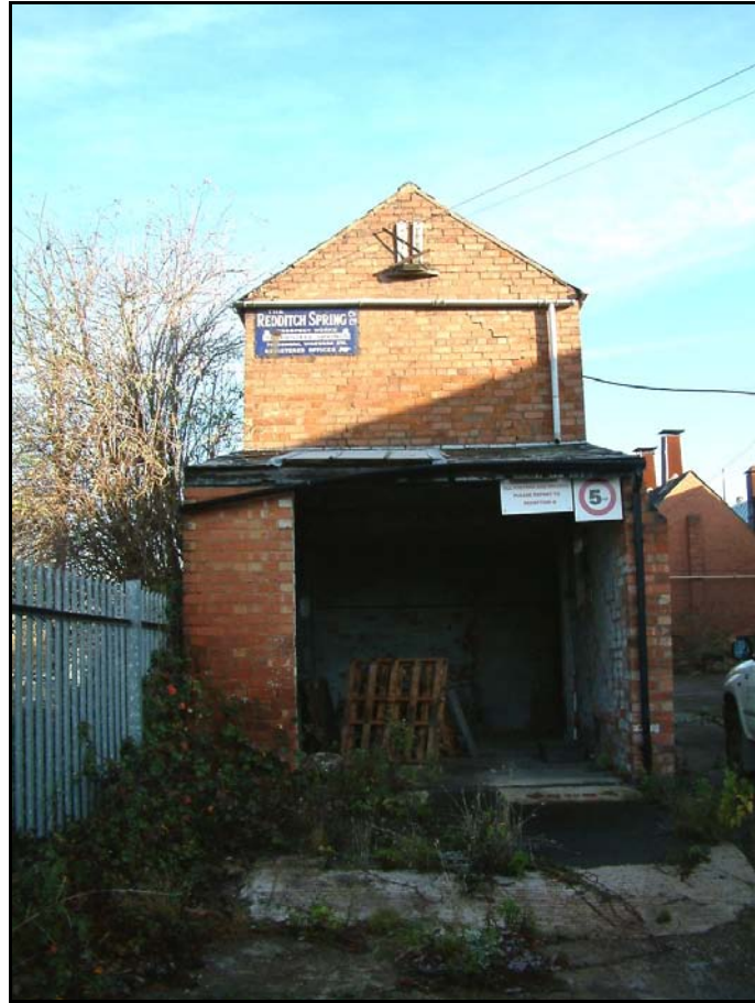
Plate 15: Range 3 building A, from the south
