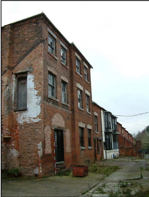
Plate 8: Range 1 building D from the north
