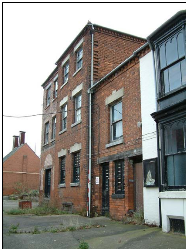
Plate 6: Range 1 building C (left centre) from the south
