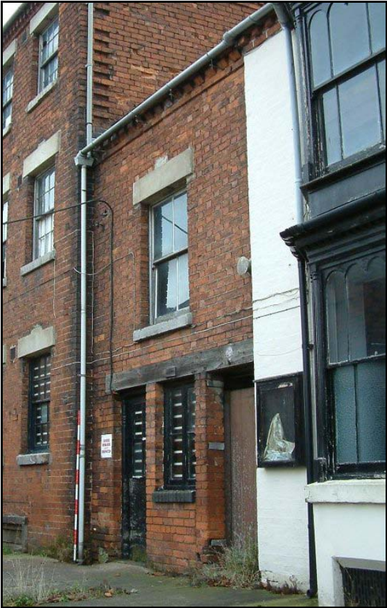
Plate 3: Range 1 building B, from the south
