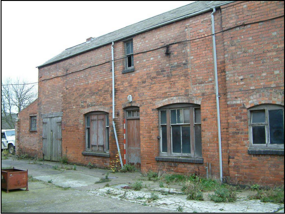
Plate 18: Range 3 building B, from the north
