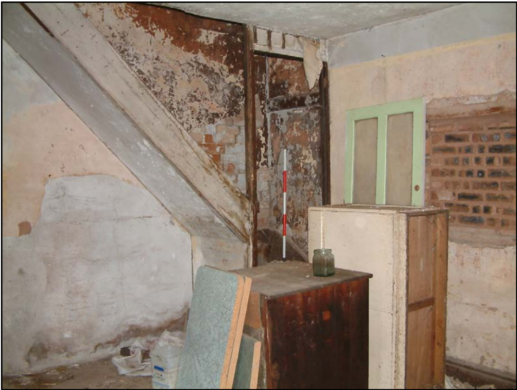
Plate 21: Range 3 building B, showing the staircase
