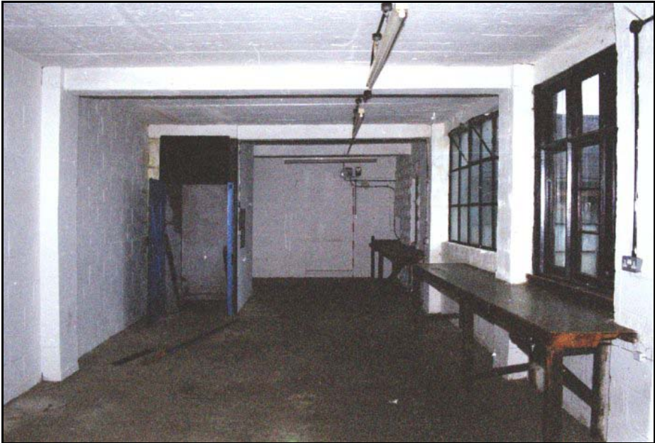
Plate 12: Interior of Range 1 building E
