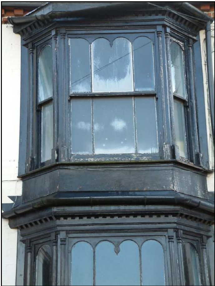
Plate 2: Windows of range 1 building A
