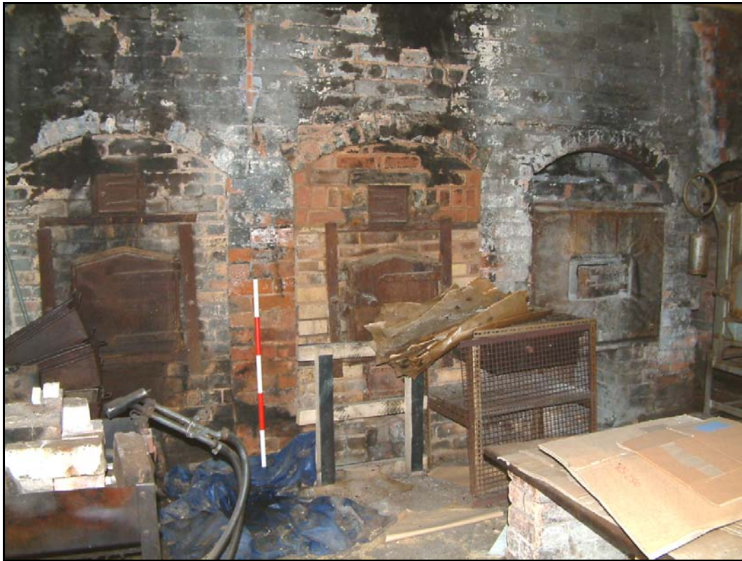
Plate 27: Range 4 building A, the forges
