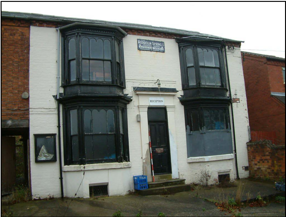
Plate 1: Range 1 building A, from the west
