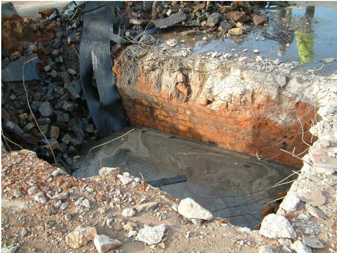
Plate 3: Basement at north end of Trench55.
