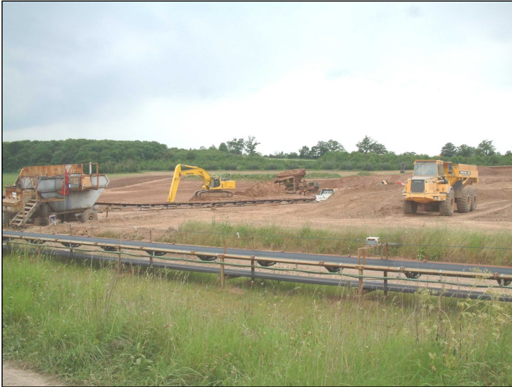
Plate 3: Area currently under extraction – looking west
