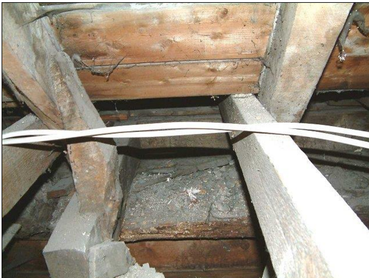
Figure 29: Investigation hole B, truss supported by wall plate
