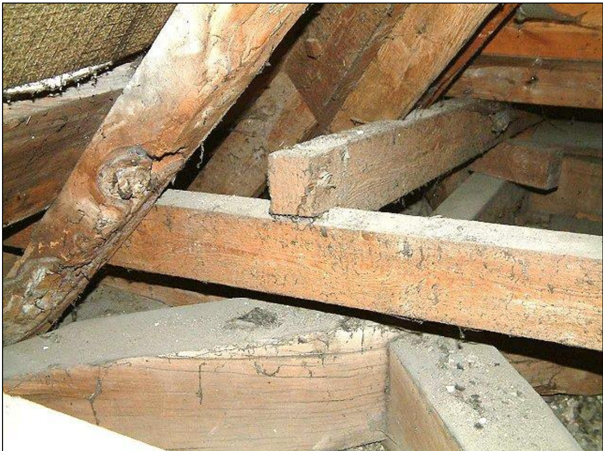
Figure 31: Investigation hole C, dragon tie beam and truss
