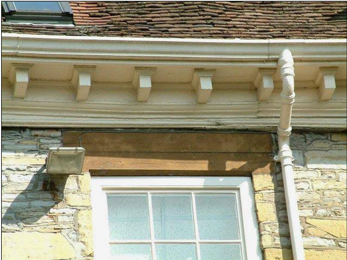
Figure 30: Investigation hole B, window lintel from exterior
