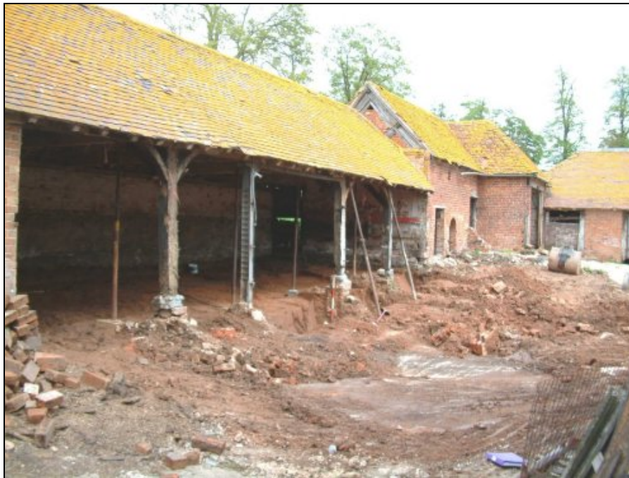
Plate xxvi Milking parlour following ground works
