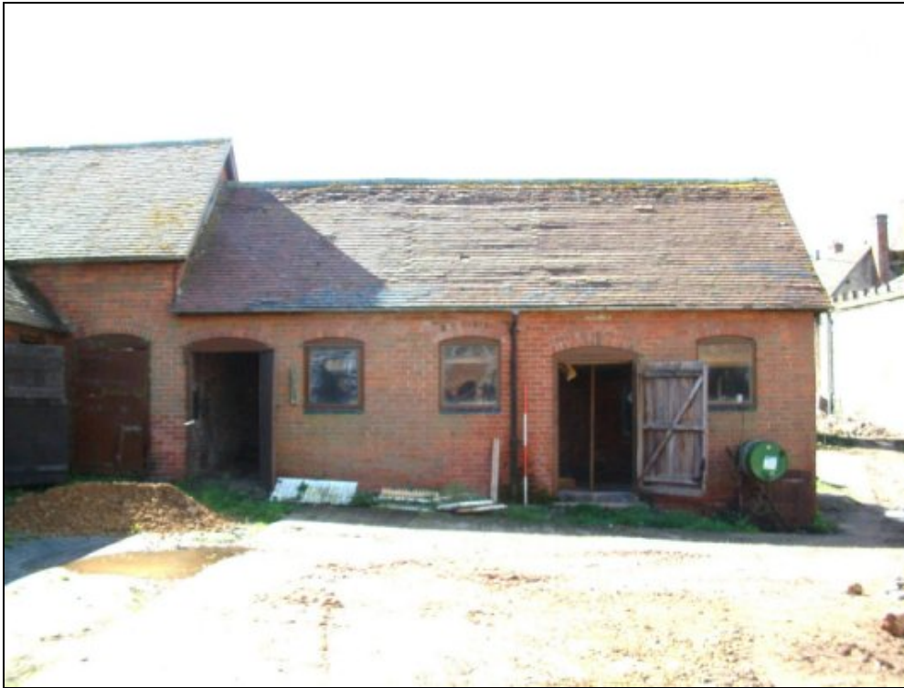
Plate xxi North facing elevation of southern range – wood shed and stores A and B
