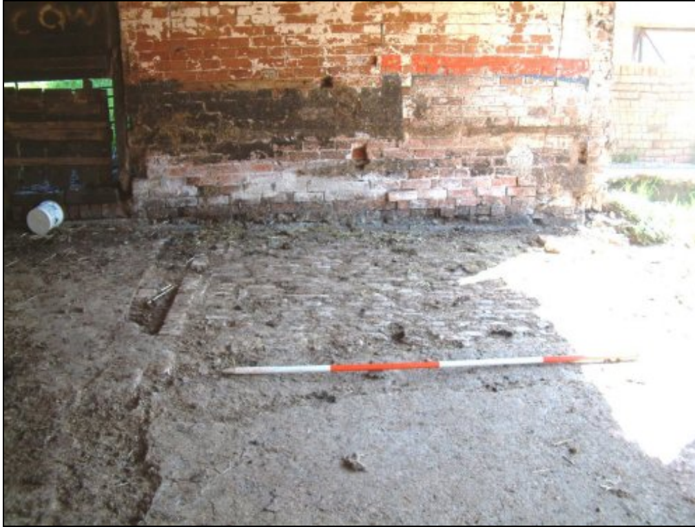
Plate vii Internal floor at east end of milking parlour
