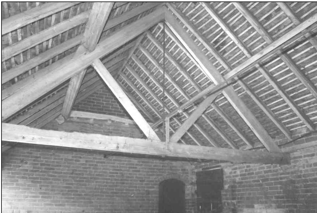
Plate xx Truss in implement store A
