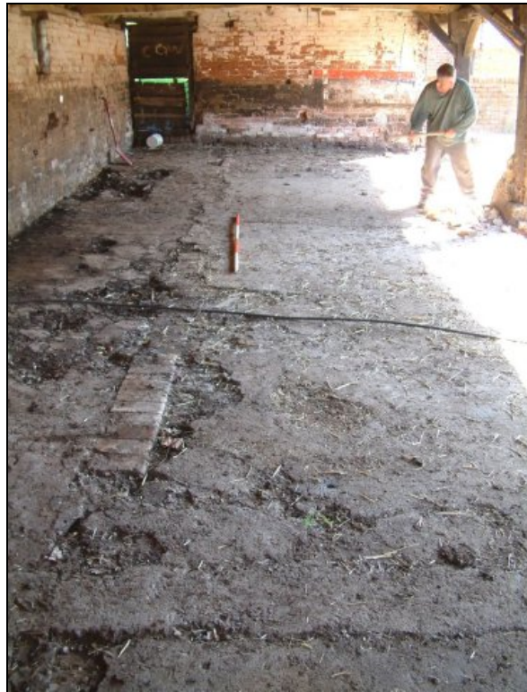
Plate xxiv Floor of milking parlour during ground works
