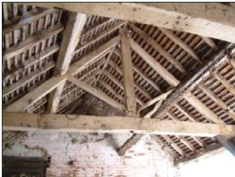
Plate iv Truss in milking parlour
