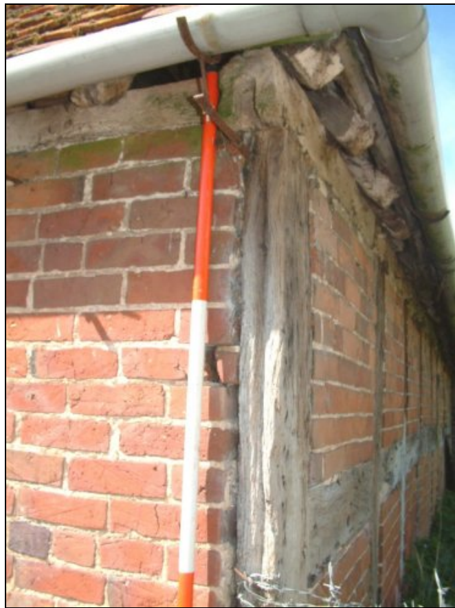
Plate xii Detail of mortice joint and groove at east corner of pig cote
