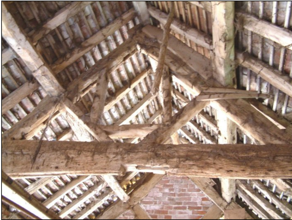
Plate xiii Truss in pig cote
