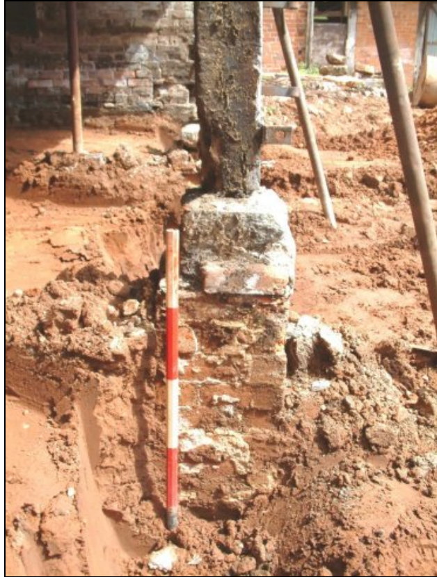
Plate xxvii Detail of brickwork below frontage beam of milking parlour
