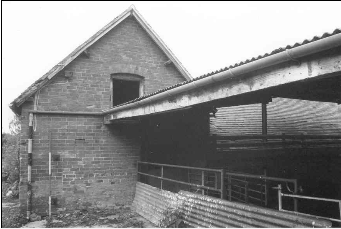
Plate xxiii East facing elevation of wood shed
