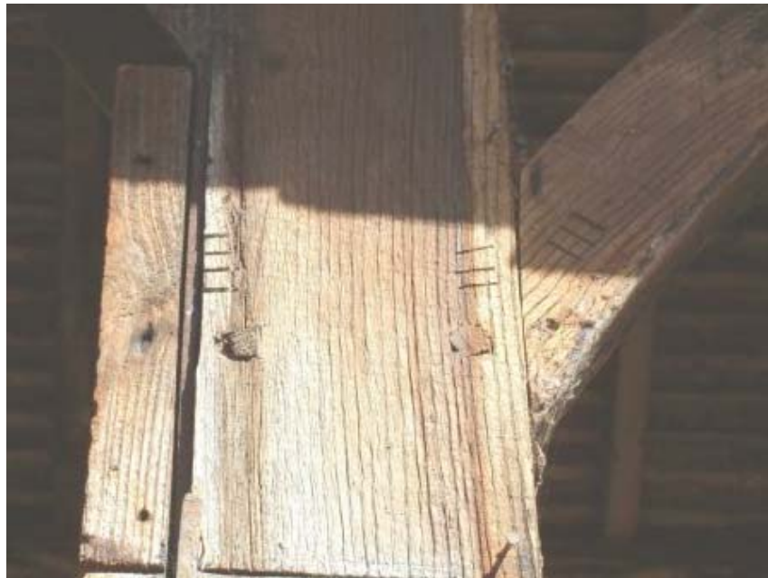
Plate vi Carpenters marks on main support beam of milking parlour south elevation
