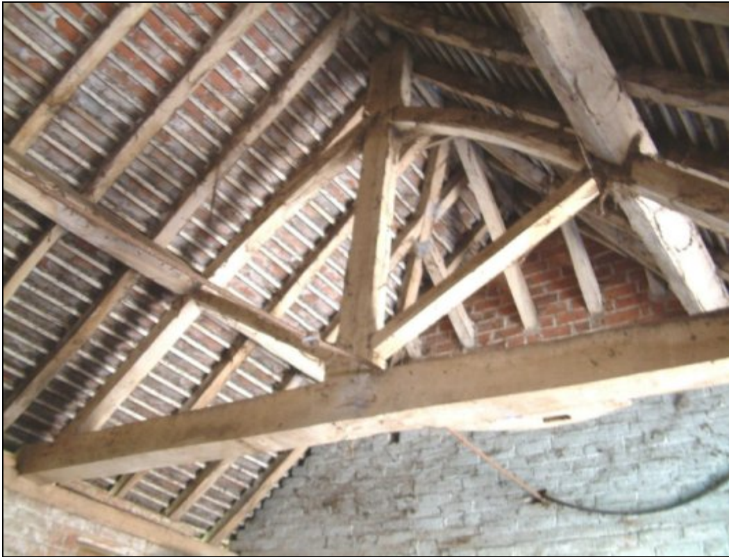
Plate xix Truss in byre
