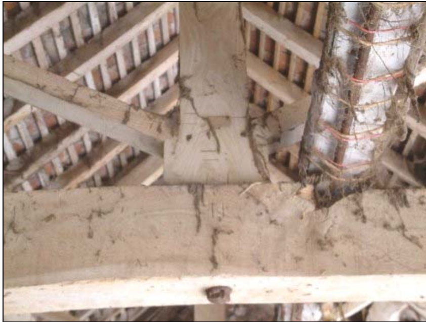
Plate v Carpenters marks on milking parlour truss
