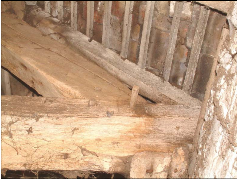
Plate xvii Detail of truss in store C
