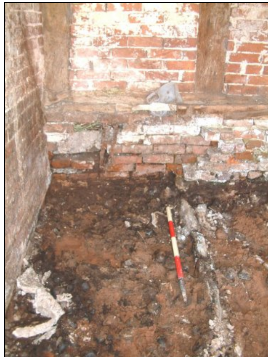
Plate xxix South facing elevation and ground following ground reduction in store C
