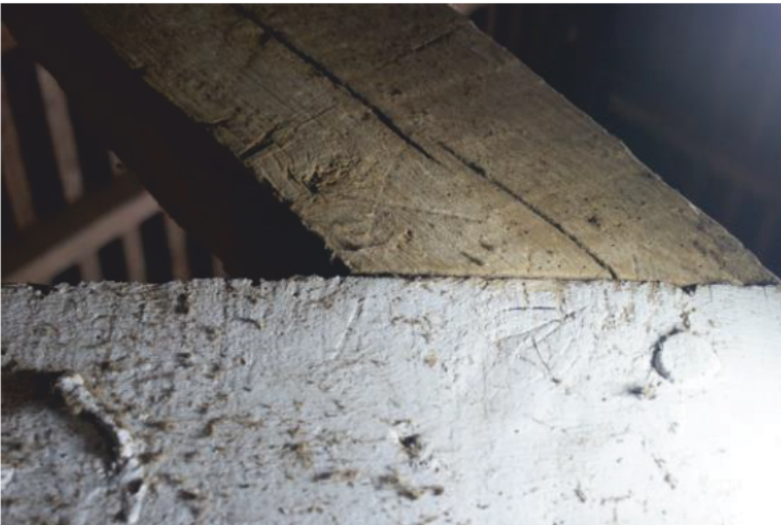
Plate 12 Phase 1 shelter shed, looking north-east
