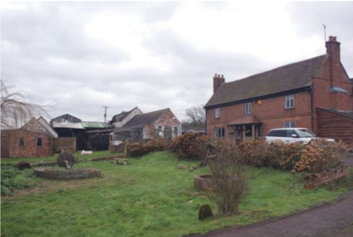
Plate 1 The house and farm buildings, looking north-east
