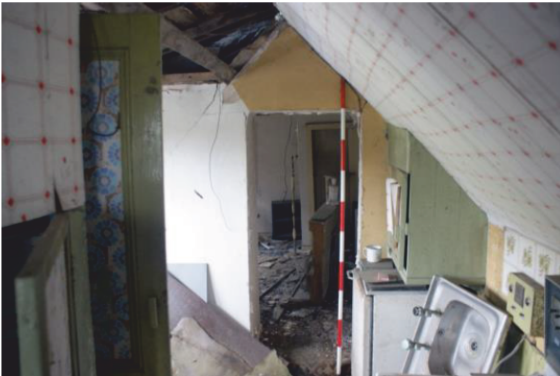
Plate 47 Phase 5 first floor conversion of the cart shed, looking south-west
