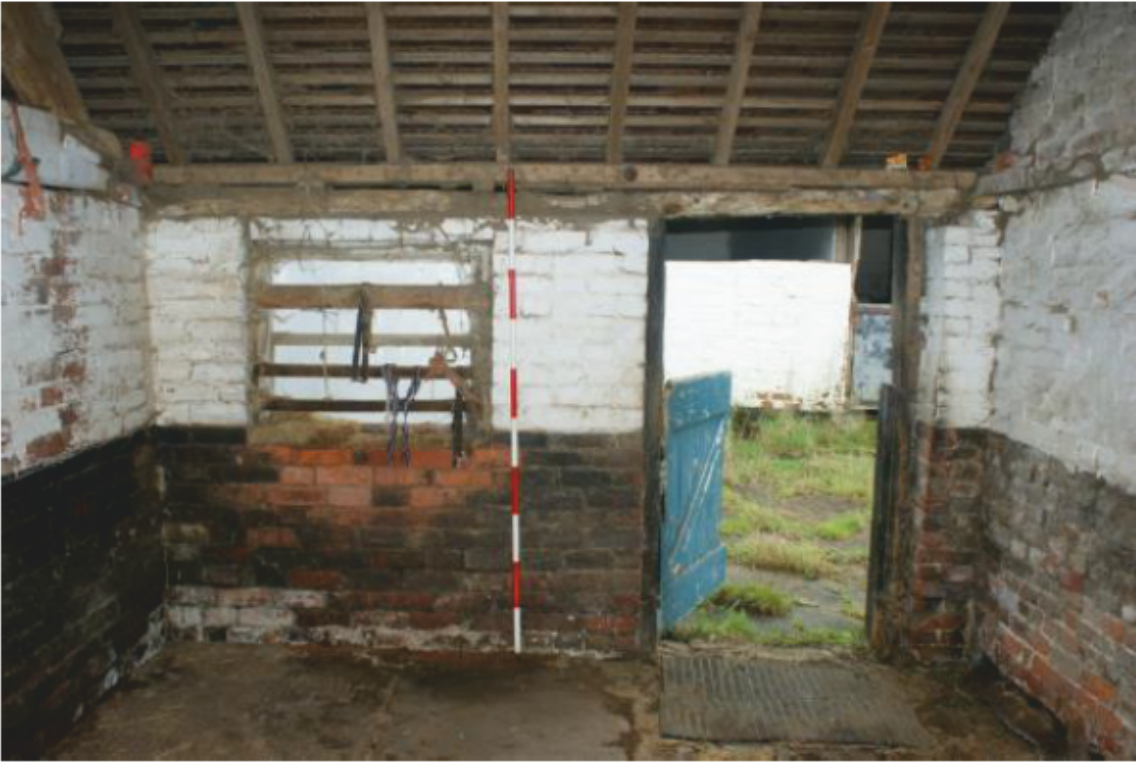
Plate 7 Phase 1 shelter shed, looking south-east
