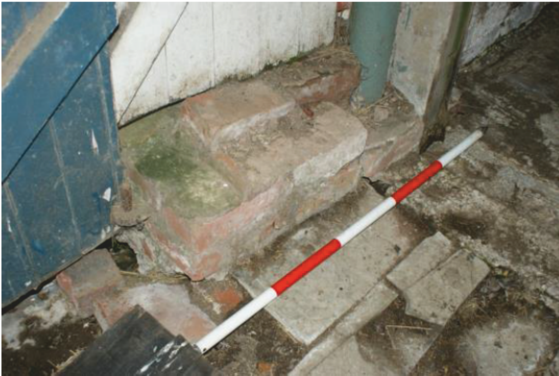
Plate 17 Remnant of Phase 1 threshing barn, looking south-west
