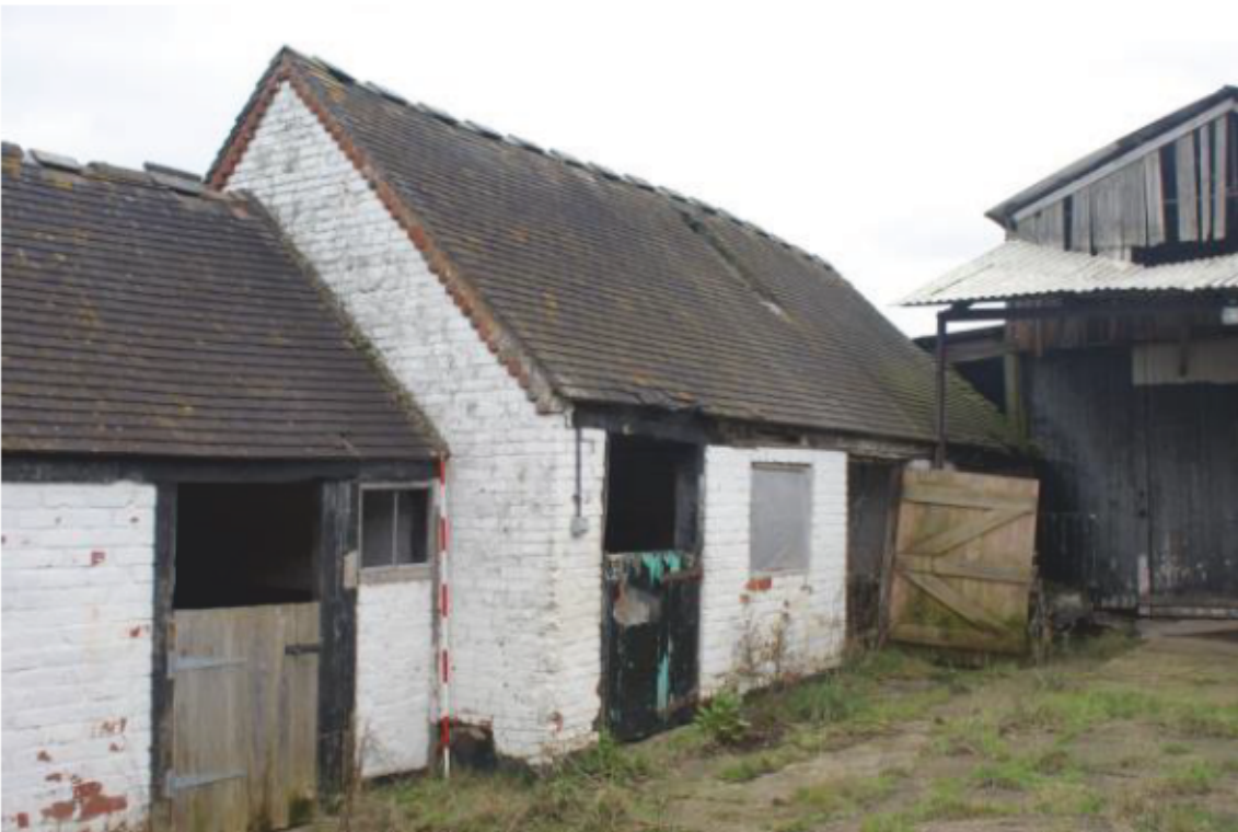
Plate 4 Phase 1 shelter shed, looking north
