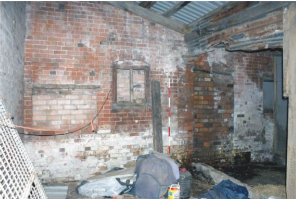
Plate 27 Phase 2 stable and hayloft, looking south-east
