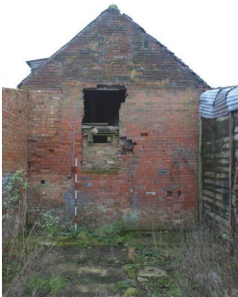
Plate 30 Phase 2 stable and hayloft, looking south-west
