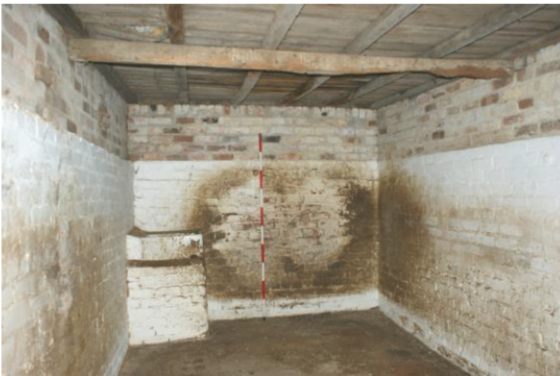
Plate 39 Phase 4 stables, looking north-west
