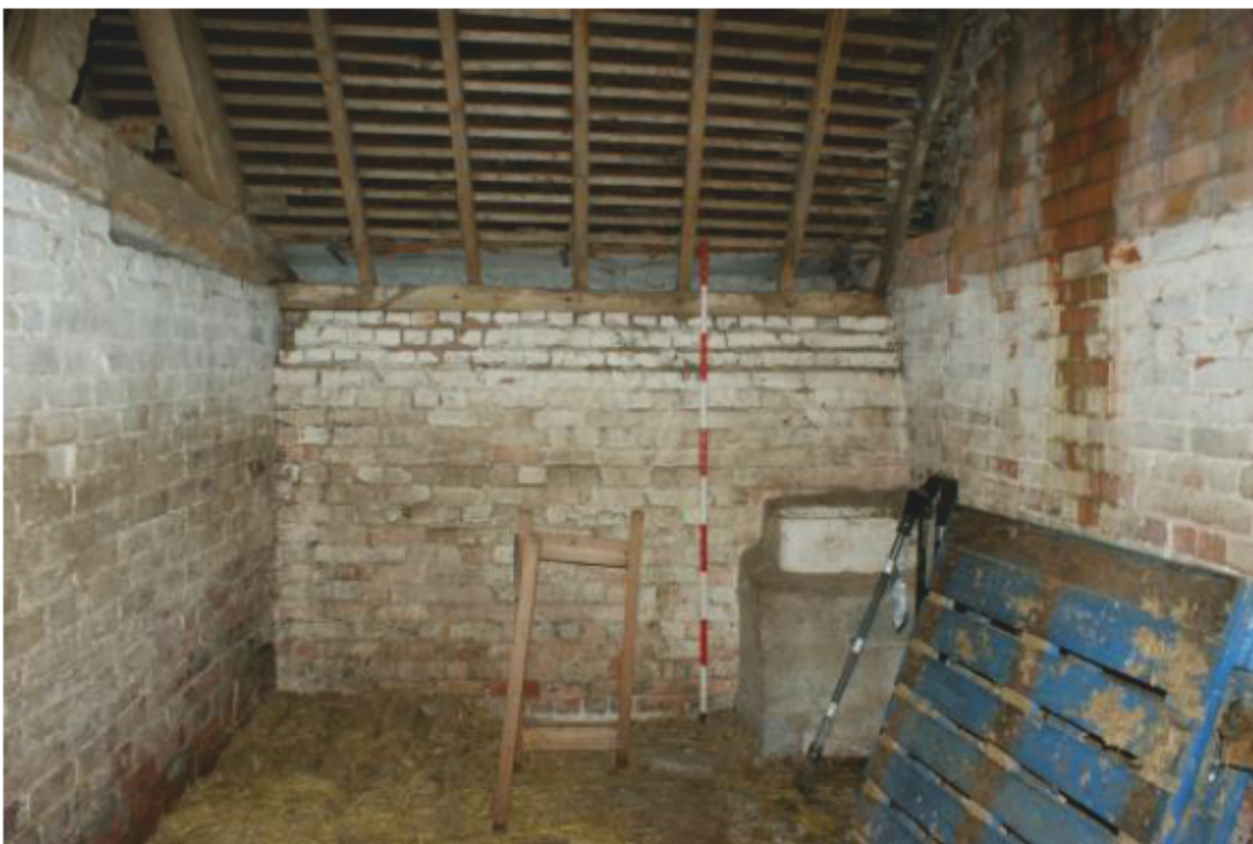
Plate 6 Phase 1 shelter shed, looking north-west
