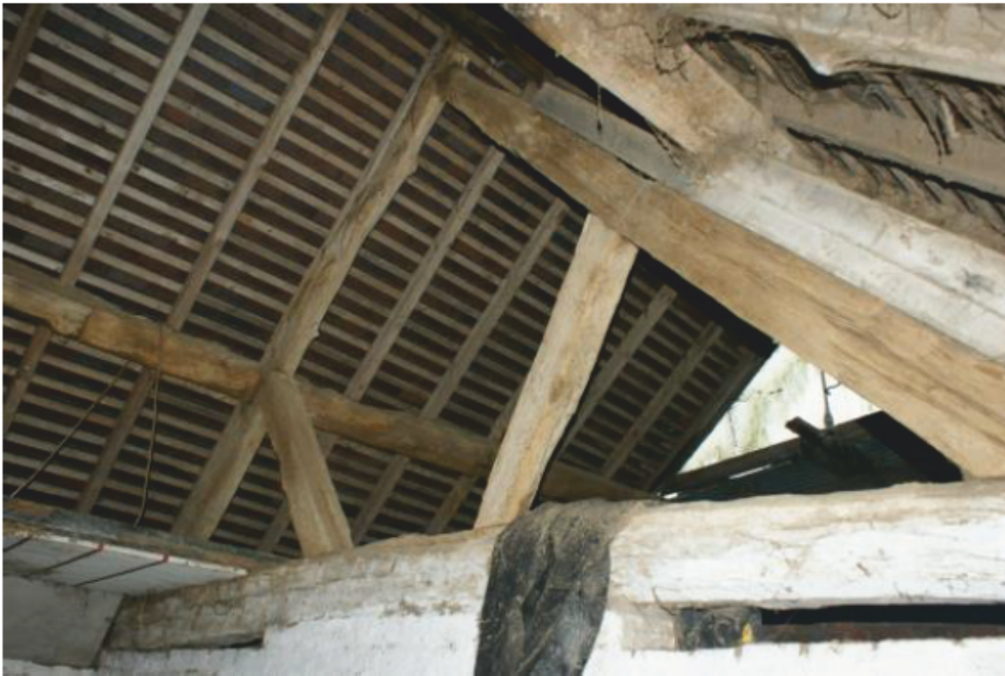
Plate 5 Phase 1 shelter shed, looking north
