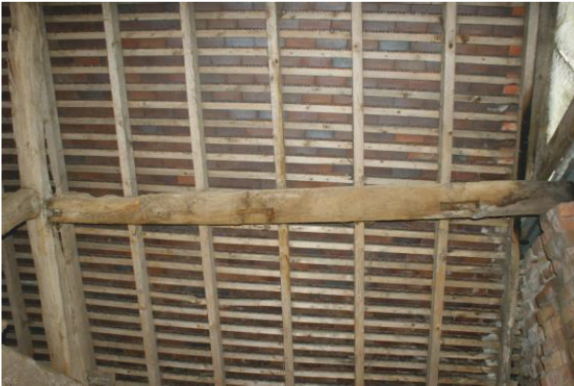
Plate 13 Phase 1 shelter shed, looking north-west
