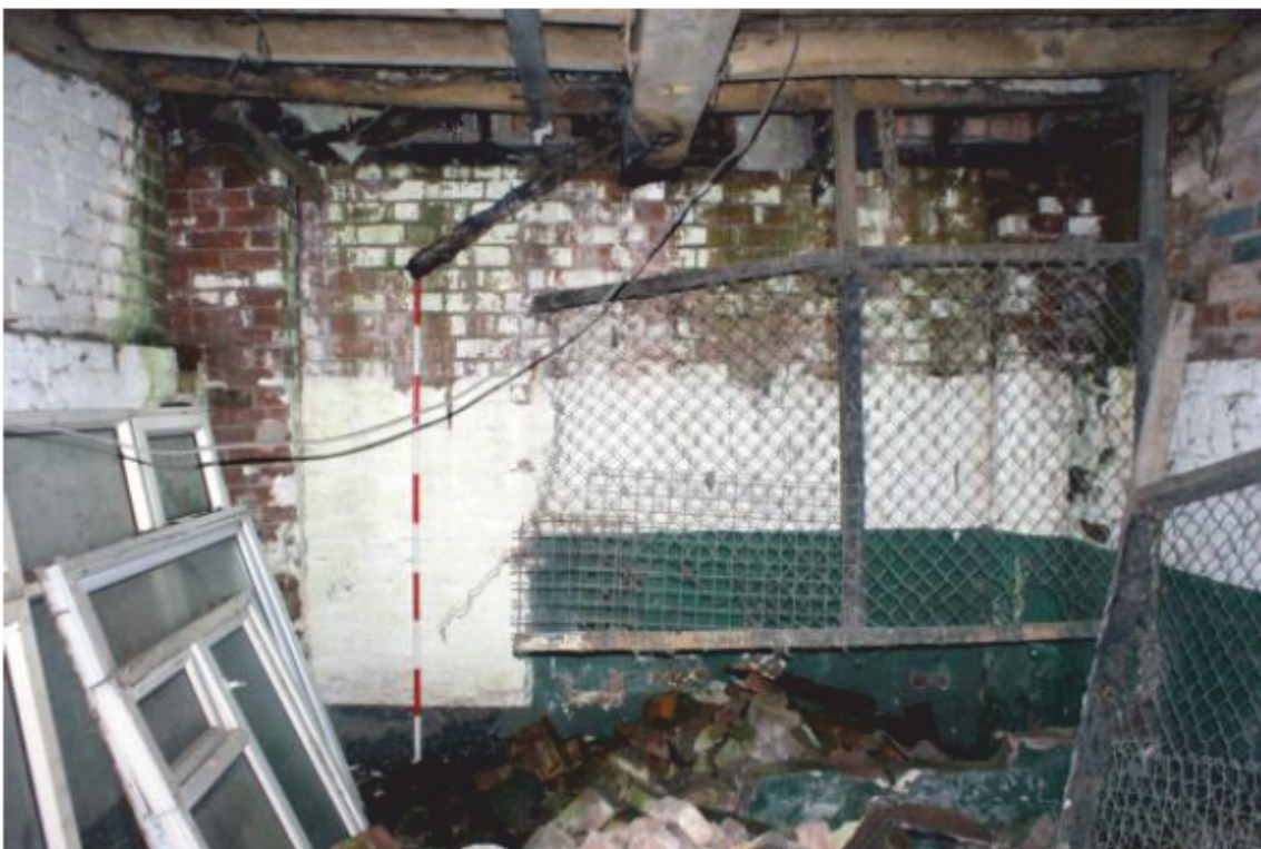
Plate 25 Phase 1 Cart shed, looking north-west
