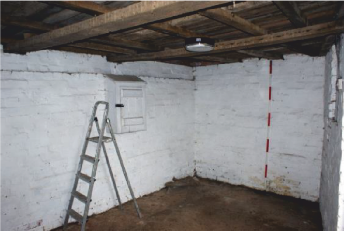
Plate 40 Phase 4 feed room, looking east
