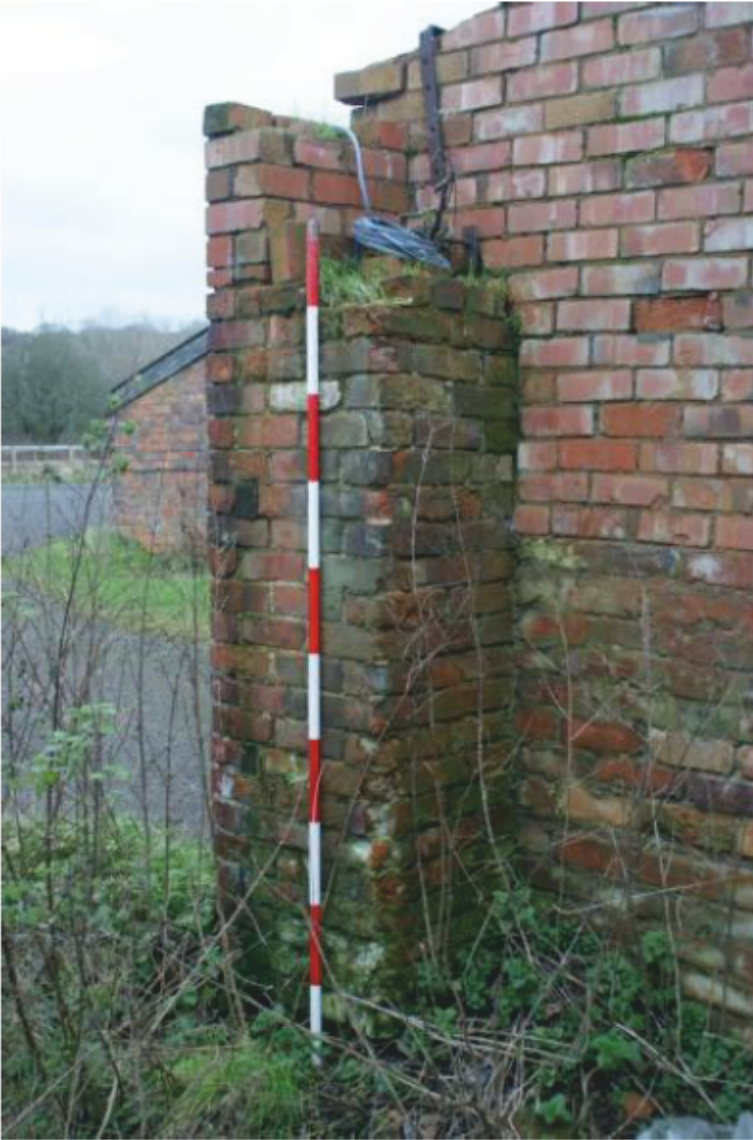
Plate 19 Possible remnant of Phase 1 structure, looking north-east
