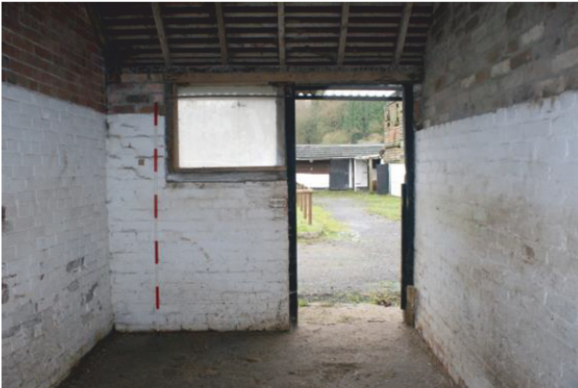
Plate 38 Phase 4 stables, looking south-east
