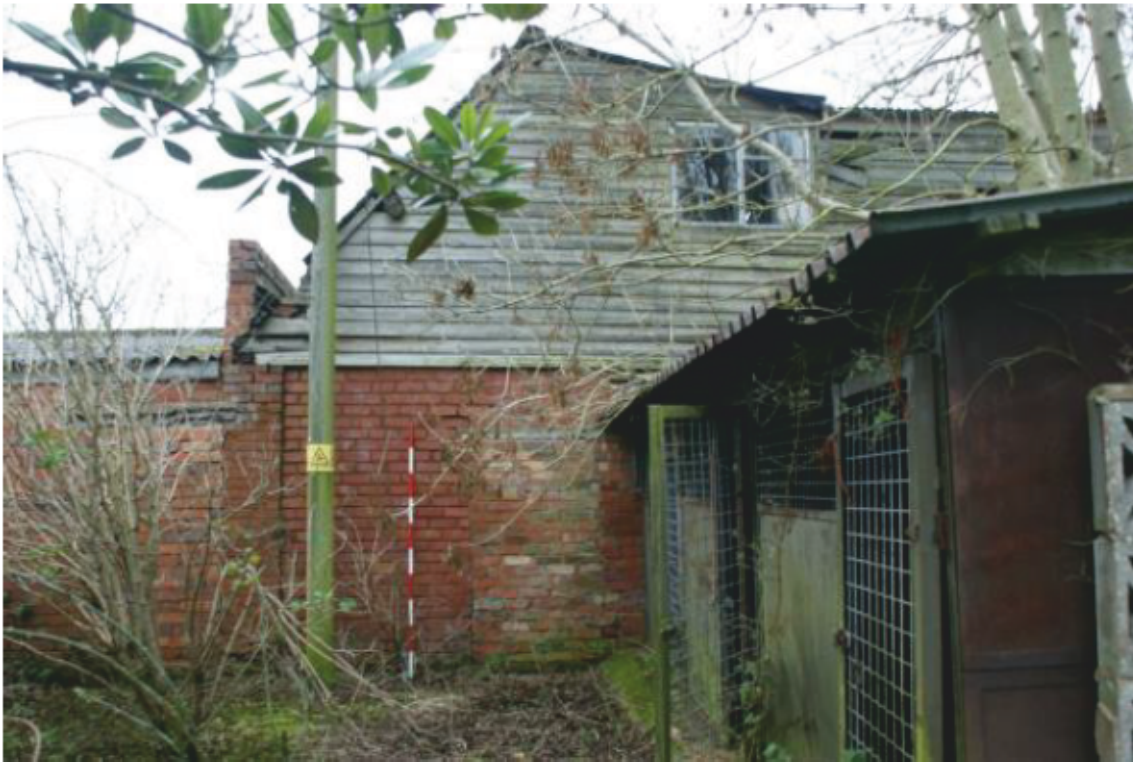
Plate 22 Phase 1 Cart shed, looking north-east
