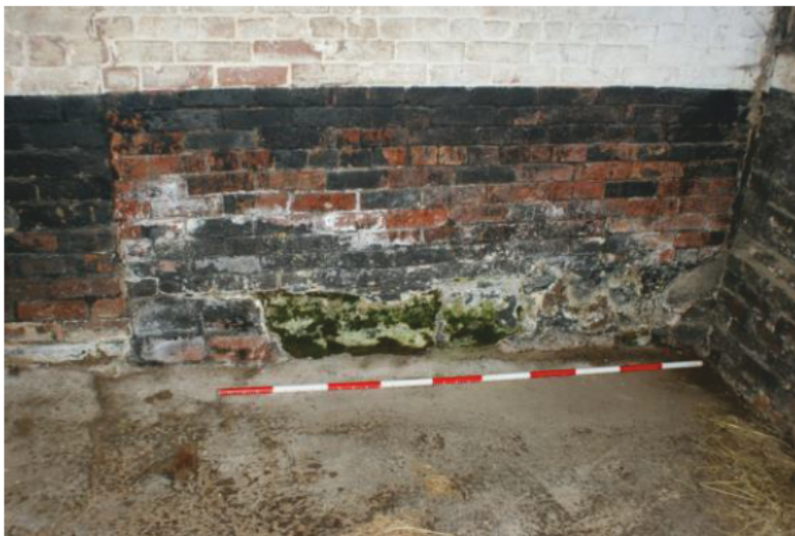
Plate 9 Phase 1 shelter shed stone foundation, looking north-east
