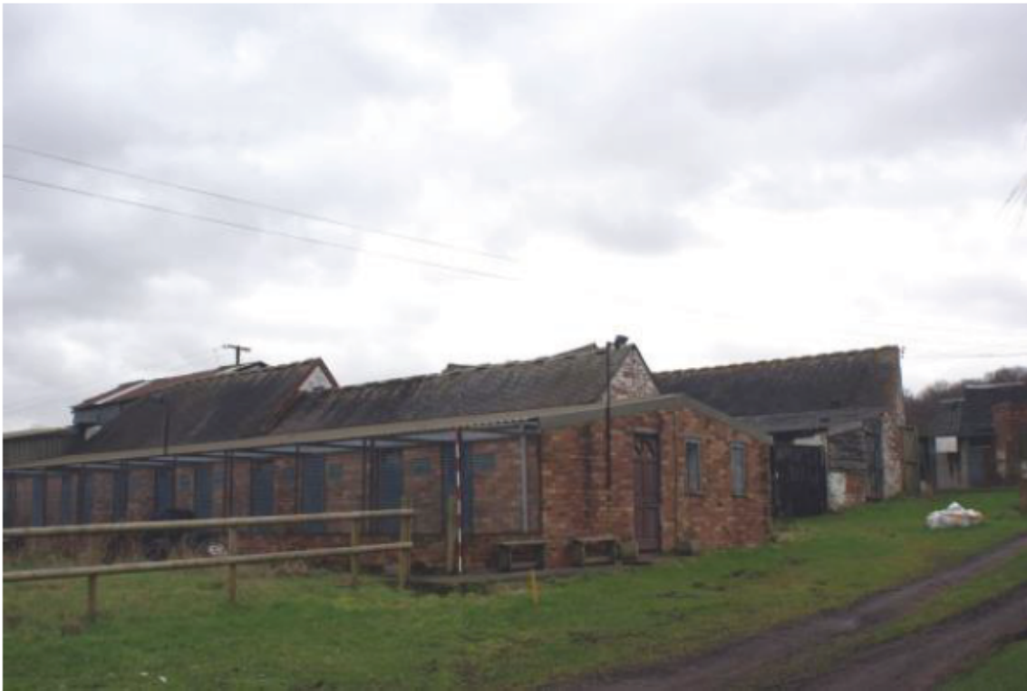
Plate 46 Phase 4 re-roofing, looking east
