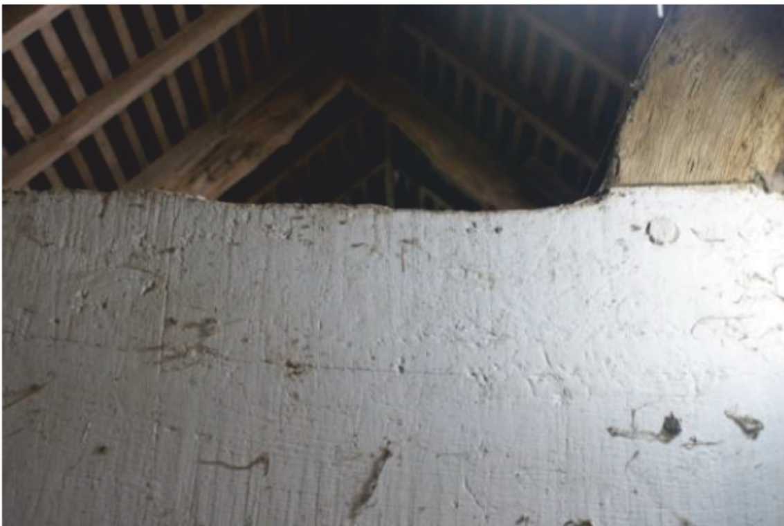
Plate 16 Phase 1 shelter shed, looking north-east
