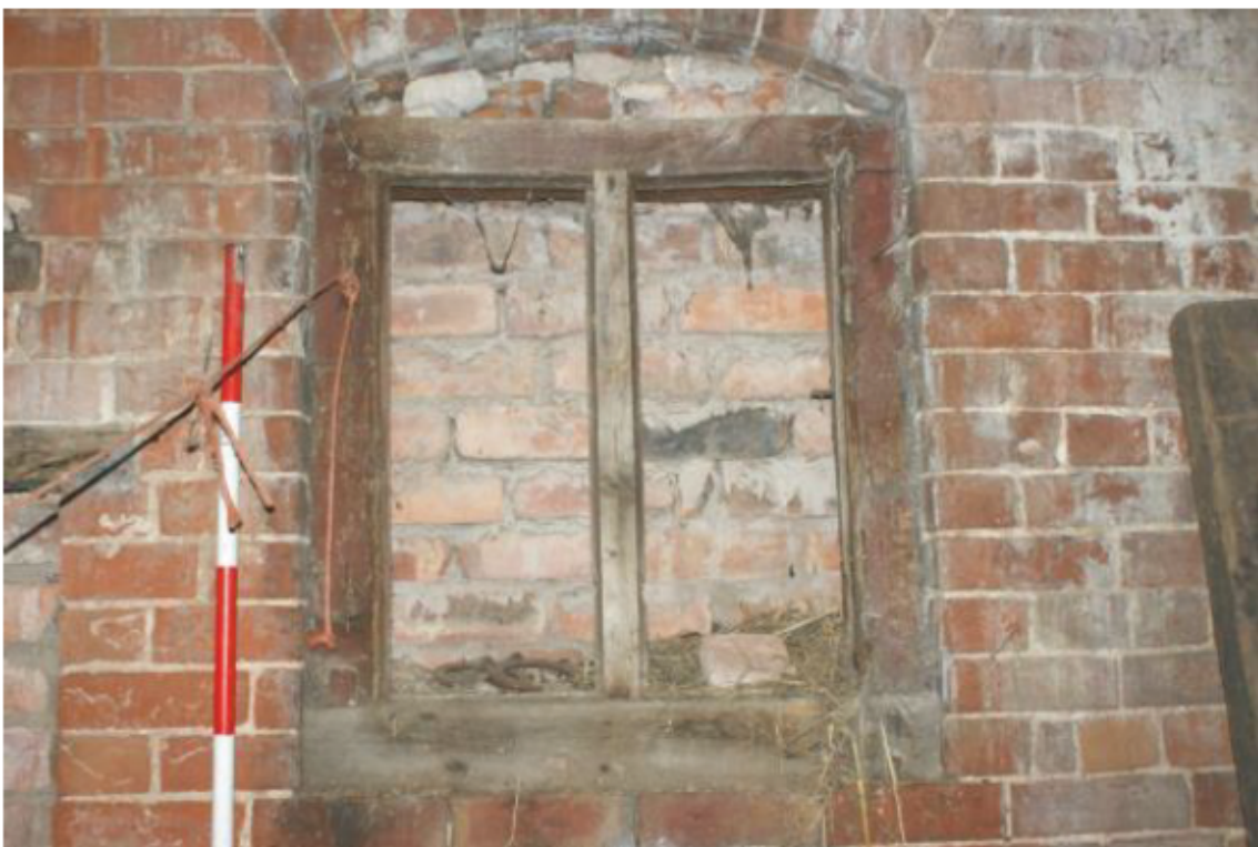
Plate 29 Phase 2 stable and hayloft, looking south-east
