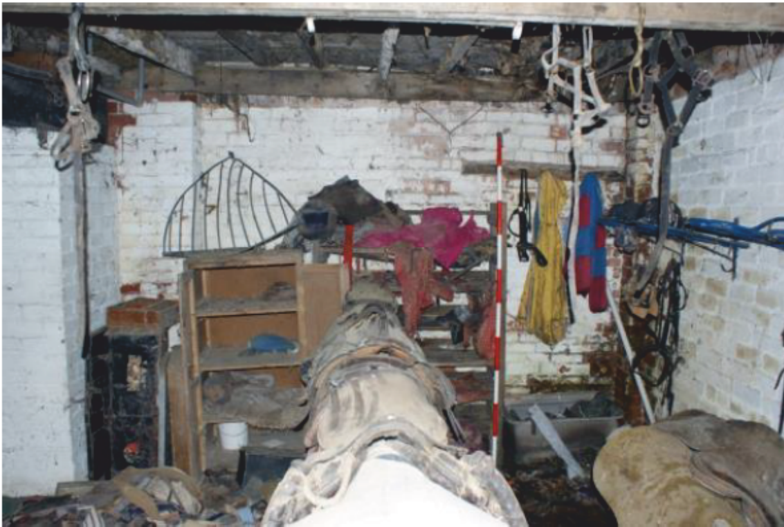
Plate 24 Phase 1 Cart shed, looking south-east
