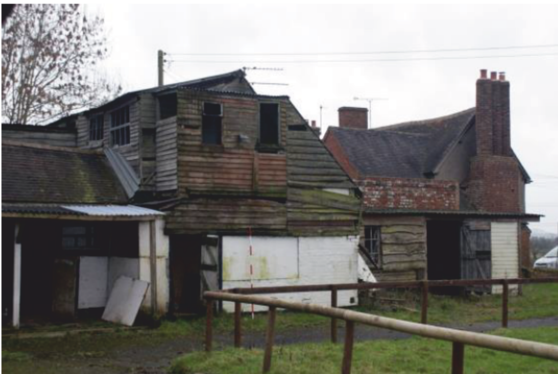
Plate 21 Phase 1 Cart shed, looking west
