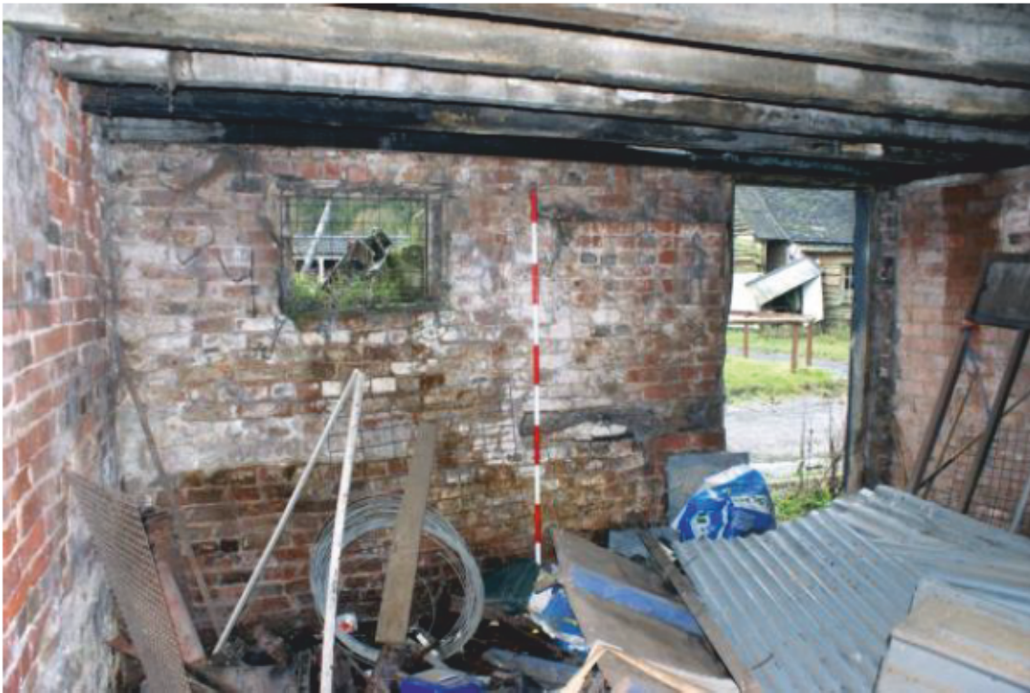
Plate 31 Phase 2 stable and hayloft, looking south-east
