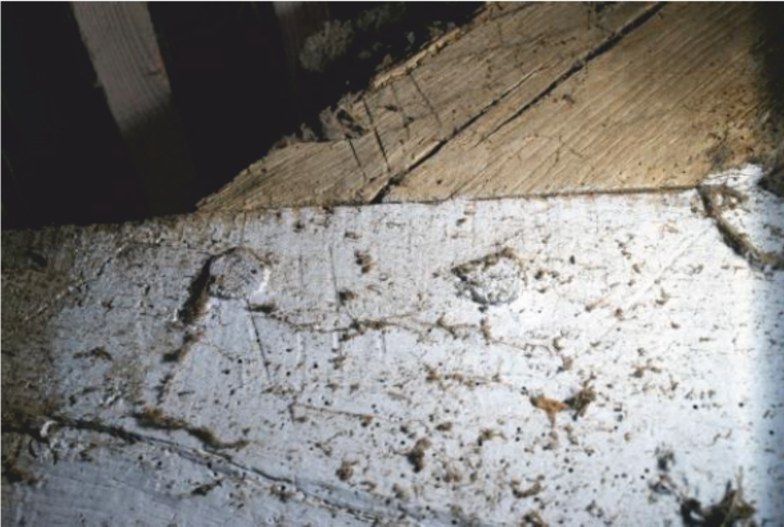
Plate 11 Phase 1 shelter shed, looking north-east
