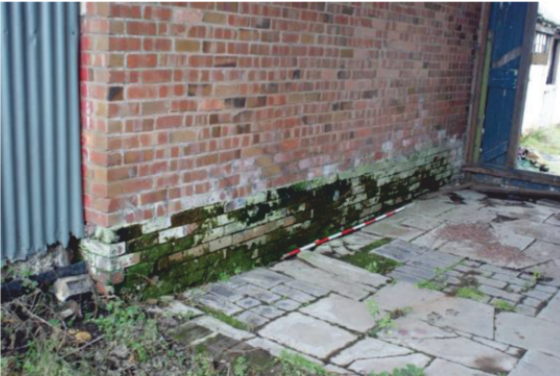
Plate 36 Phase 3 rebuild of the threshing barn, looking south
