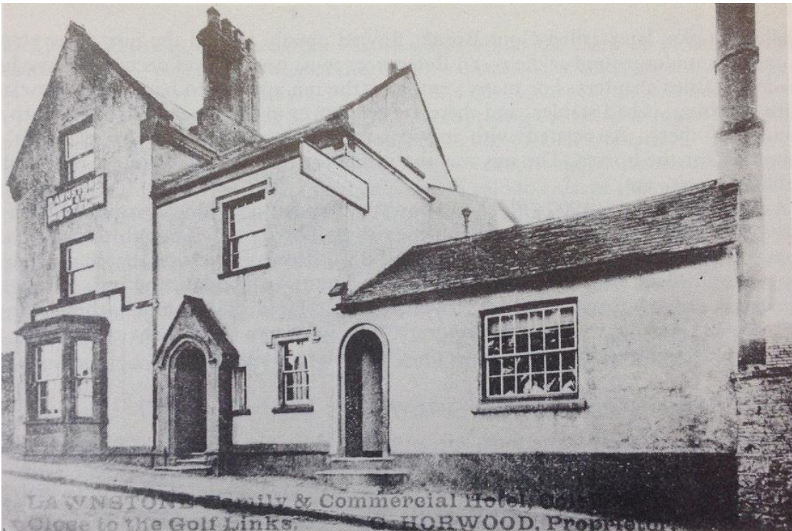
Plate 10: East elevation of Lawnstone House, c 1910; with bay window and two doorways (subsequently removed), and the single storey north wing (subsequently raised to two storeys) (Hart 1983, plate 25a)
