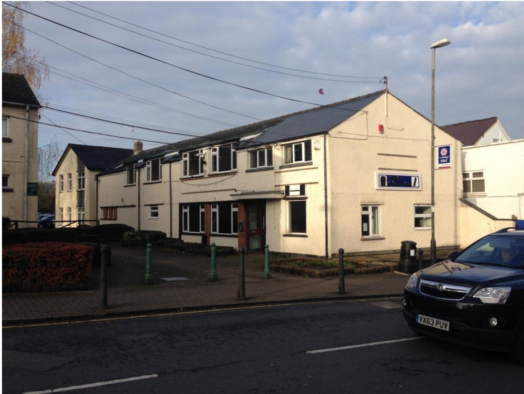
Plate 3: The Annex from the south-east; part of this building may originally have been stables
