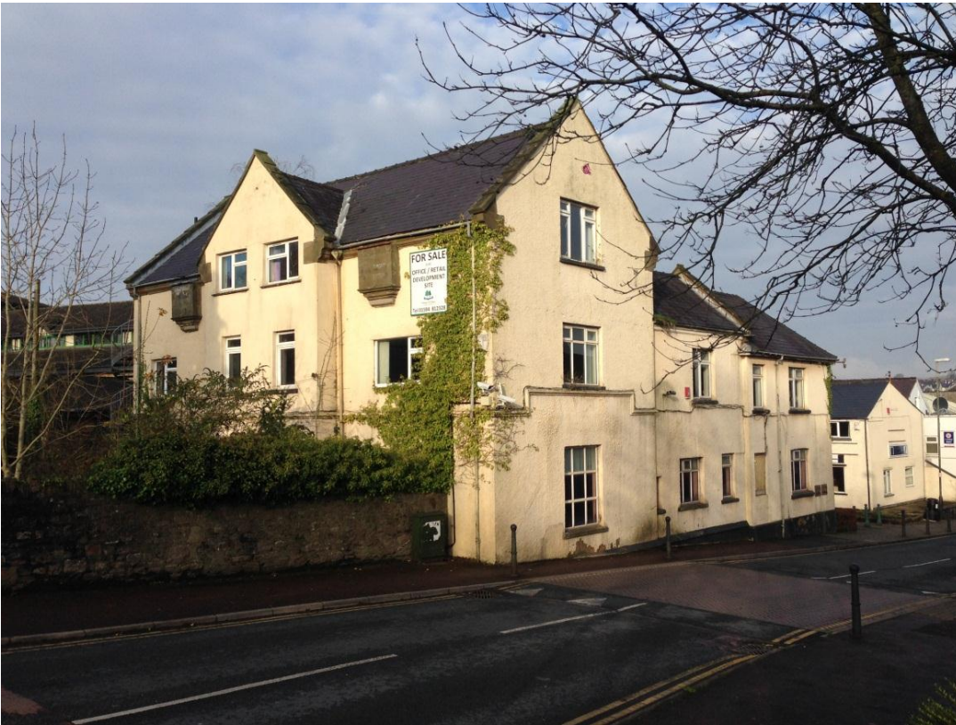
Plate 1: Lawnstone House from the south-east; comparison with a historic photograph dated c1910 (Plate 10) indicates two doors and a bay window have been removed from the east elevation
